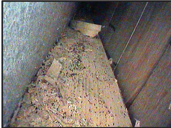
**Figure 3.5.** Videoscope image of interior fenestration cavity showing termite frass.
