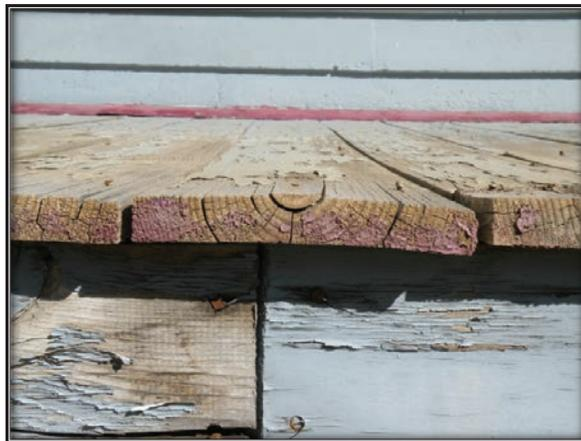
**Figure 4.27.** Flat-sawn deck board that has crowned due to differential shrinkage and swelling (material not from the Salk).
