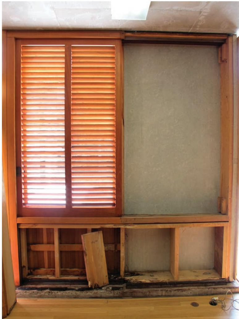
interior walls of the studies and offices. The gap between the tops and bottoms of the window walls and adjacent concrete wall is filled with a sealant. Although base and head flashing was called for in the original design and shop drawings, none was observed during the two investigative probes carried out as part of this project.
