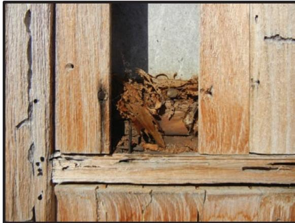
**Figure 4.12.** Location of specimen E and the surrounding teak slats showing superficial drywood termite damage.
