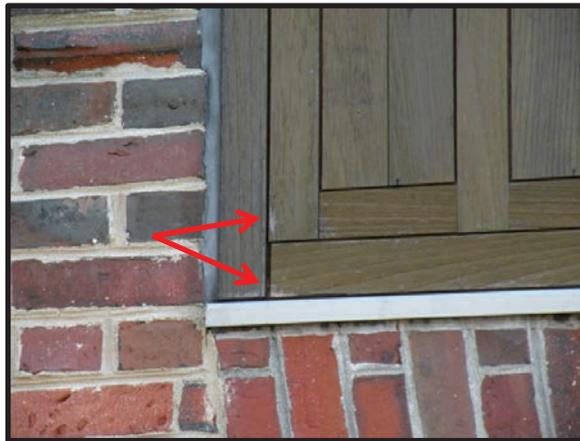
**Figure 7.7.** North elevation, first-floor teak fenestration unit. The arrows indicate where that the treatment has begun to fail.
