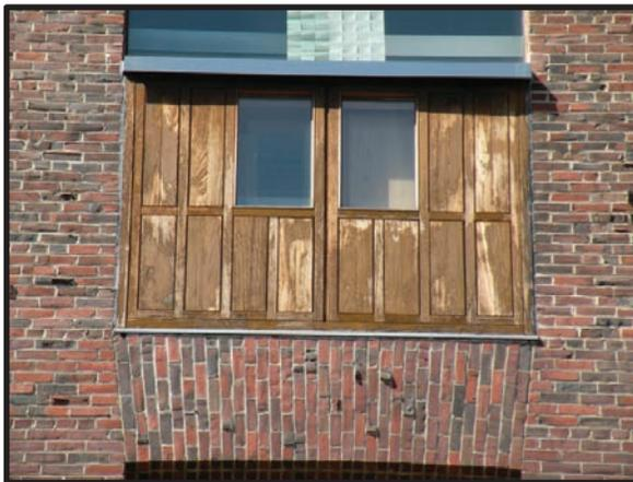
**Figure 7.11.** Third floor, teak fenestration unit, south elevation.
