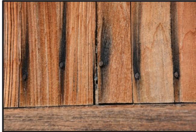
**Figure 6.1.** Vertical-sawn and rift-sawn slats on the left show a rough, ridged surface texture, while flat-sawn slats on the right show a smoother, more uniform appearance. The black stains are due to corrosion of the nails, not to the cut of the wood.
