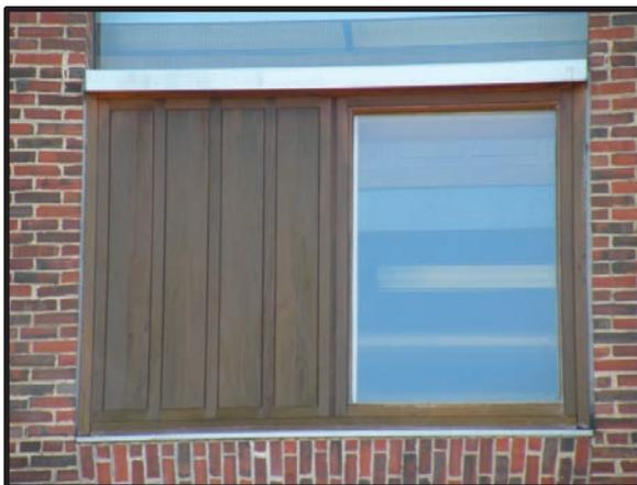
**Figure 7.5.** Third floor, teak fenestration unit, north elevation.
