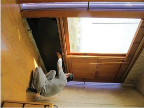
SO4B, AFTER REMOVAL OF OAK PANELING, SHOWING BUILDING PAPER AT INSIDE FACE OF FRAMING
