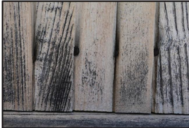
**Figure 6.2.** Two flat-sawn slats with minimal biological growth adjacent to rift-sawn and vertical-sawn material with more concentrated biological growth.
