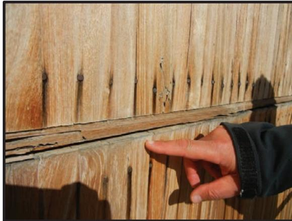
**Figure 3.3.** Visual inspection of a panel with significant weathering and erosion.
