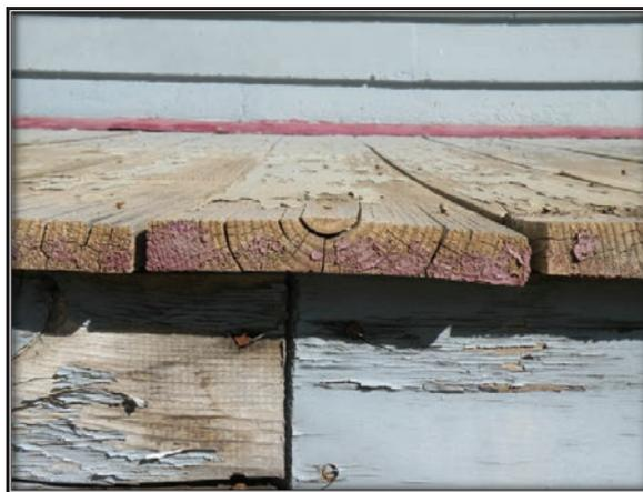
**Figure 4.27.** Flat-sawn deck board that has crowned due to differential shrinkage and swelling (material not from the Salk).
