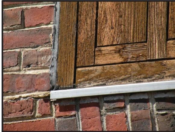
**Figure 7.12.** Close-up of teak fenestration unit on south elevation showing that the treatment has weathered severely and has been largely ineffective in maintaining the appearance or protecting the wood.
