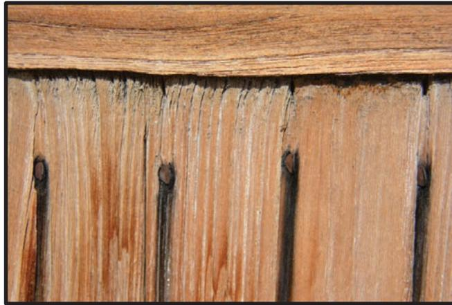
**Figure 2.3.** Stains on teak slats caused by a combination of moisture and a chemical reaction between extractives in the wood and the exposed metal fasteners after significant weathering occurred.
