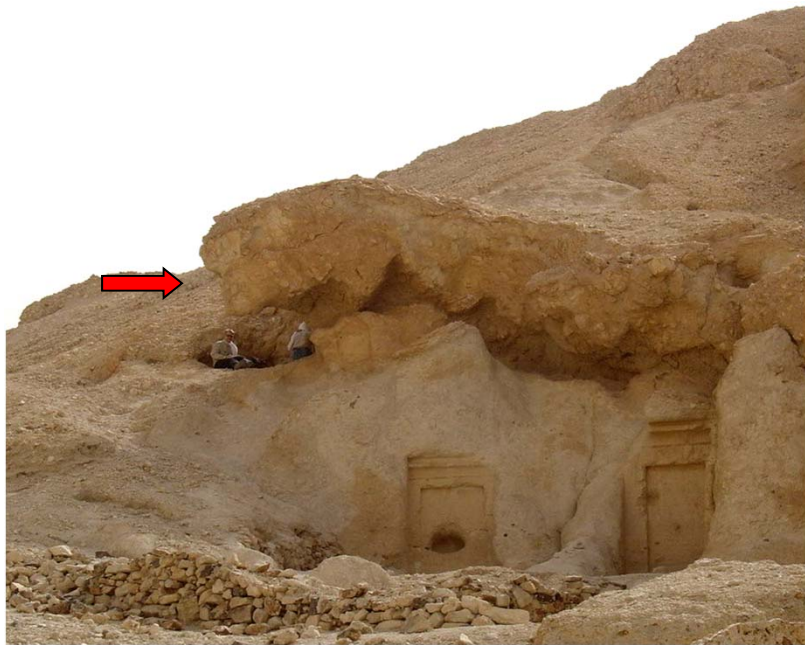
Breccia rock outcrop above chapels A and B undercut by preferential erosion of the shaley marl layer underlying it. The breccia outcrop's lack of structural support, particularly in the area of Chapel A (indicated by arrow), puts it at risk of collapse.
