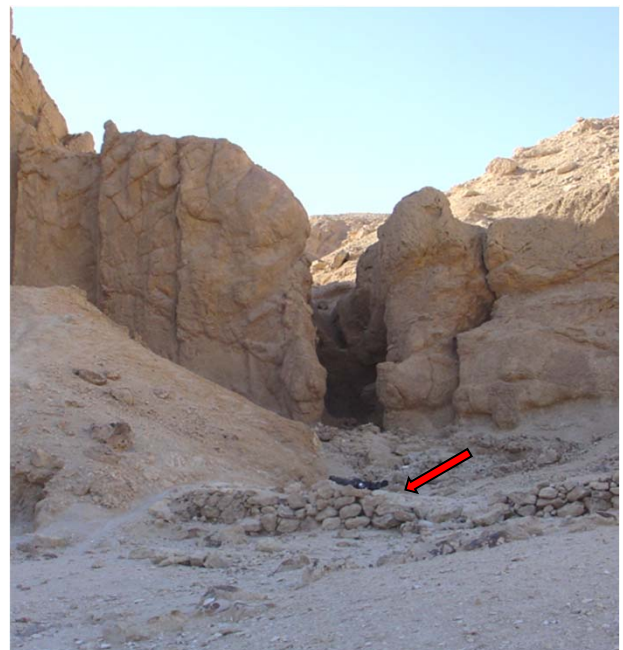
2008 view showing Dam (indicated by arrow) after debris clearance.
