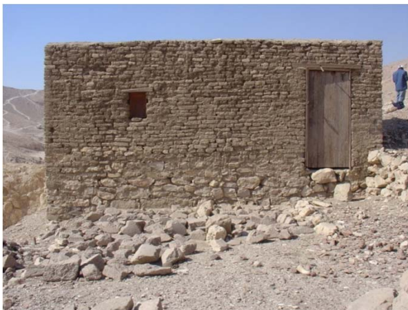
East elevation with door and window.
