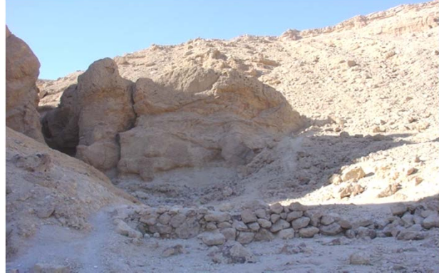
2008 view of Dam in 2007.
