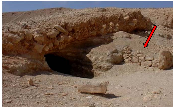
A similar view of QV 1 in 2006 showing loss of stones in the upper part of the masonry wall (indicated by arrow) and around the shelter's opening.
