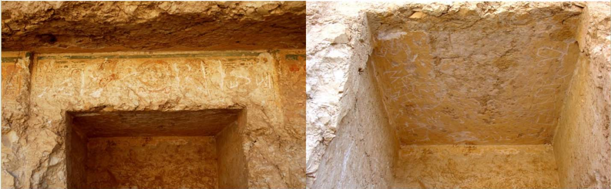
Graffiti damage to the decorated surfaces of the stele of Chapel D.
