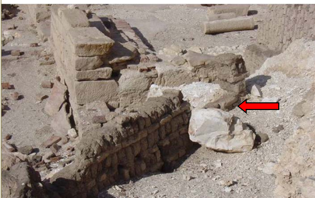
February 2008 image showing large rock leaning against lost wall section of granary.
