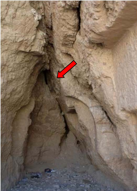
Fault (F1) running vertically through the southwest room of Chapel G.
