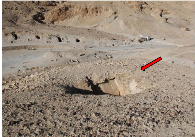
Hermit Shelter 2. Exterior view (2006) of hole in the ceiling (arrow).
