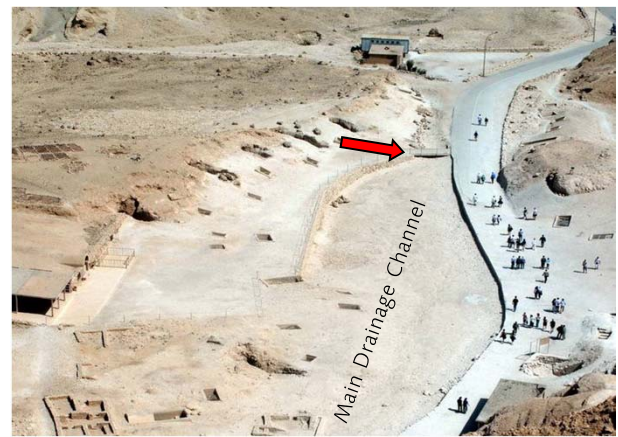
View of main drainage channel looking downstream showing channel narrowing and point of constriction at bridge (arrow).
