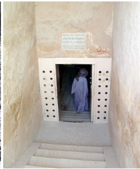
QV 52. Schiaparelli era door protects the tomb (left). There are no retaining walls or arched cover to protect the tomb from debris flow from slope above entrance; nor is there protection from flooding from the adjacent wadi. Visitors congregating in front of the tomb awaiting access put undue pressure on the entry as they attempt to gain access and seek shade.
