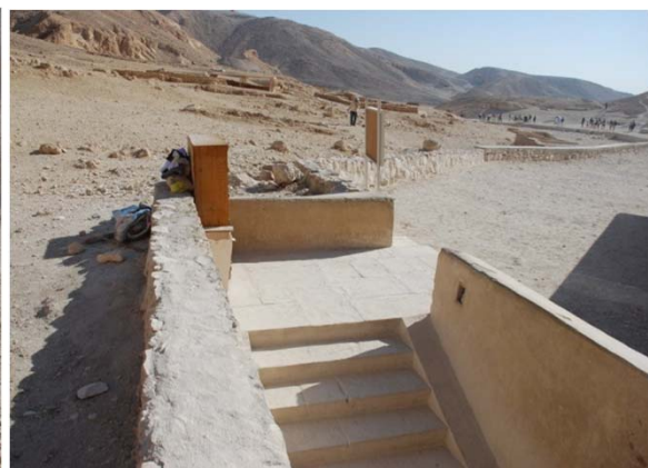
QV 55. Retaining walls and brick arched cover as built by Schiaparelli c.1905 (top left) (Image: Museo Egizio); entry with door and plaque installed by Schiaparelli as it looks today (2005) (top right). The retaining walls and brick arched cover built by Schiaparelli (the walls extended and entry created at a later date) provide some, though insufficient, protection against flooding from the wadi, as seen bottom left). The platform at the top of the steps (bottom right) becomes easily congested as groups attempt to enter and exit the ramp.
