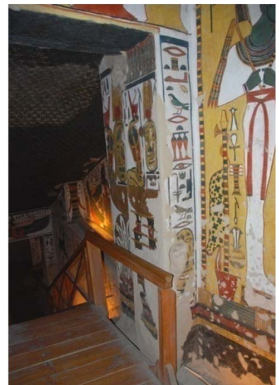
Wooden walkways and platform in Chamber K (foreground) leading to rear Chamber Q. The wooden walkways are in generally good condition, but are not of modular construction making it impossible to remove them to clean dust and lint below them.
