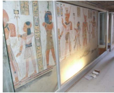
QV 44: general view of glass barriers and missing large glass panel in the corridor (right)
