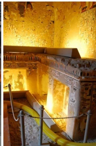
Housing for fluorescent lights on ledge in Chamber K (left), and on floor and ledge in Chamber C (right). Illumination is strong at source and falls off on upper parts of walls.
