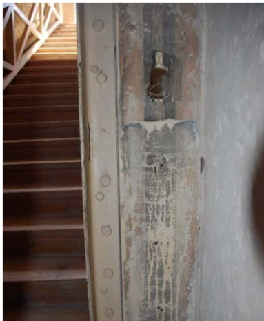
Screen over vent holes is torn and sand-clogged. Door is left open during visitation allowing air-borne particulates to enter tomb.
