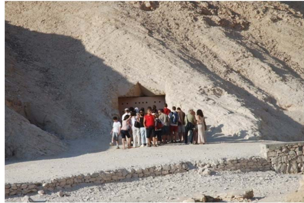
QV 52. Schiaparelli era door protects the tomb (left). There are no retaining walls or arched cover to protect the tomb from debris flow from slope above entrance; nor is there protection from flooding from the adjacent wadi. Visitors congregating in front of the tomb awaiting access put undue pressure on the entry as they attempt to gain access and seek shade.
