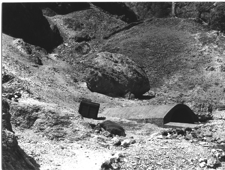
QV 52. Schiaparelli era door protects the tomb (left). There are no retaining walls or arched cover to protect the tomb from debris flow from slope above entrance; nor is there protection from flooding from the adjacent wadi. Visitors congregating in front of the tomb awaiting access put undue pressure on the entry as they attempt to gain access and seek shade.
