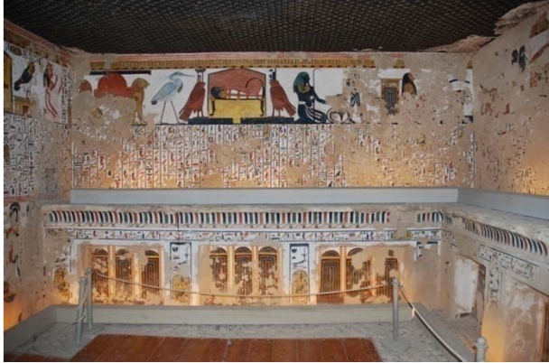
Lighting, stanchions and wooden platform in Chamber K. Note platform ends approx. 30cm from wall. Stanchions and platform function more as psychological than physical barriers. This system is viable because of the restricted number of visitors allowed at any one time in the tomb, but stanchions are unstable and potentially dangerous. Recommendations were made in the past to anchor the stanchions, which are at risk of being knocked over, to the walkways.
