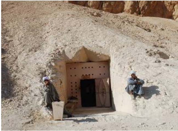
QV 52. Schiaparelli era door protects the tomb (left). There are no retaining walls or arched cover to protect the tomb from debris flow from slope above entrance; nor is there protection from flooding from the adjacent wadi. Visitors congregating in front of the tomb awaiting access put undue pressure on the entry as they attempt to gain access and seek shade.
