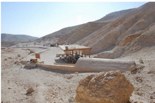
QV 55. Retaining walls and brick arched cover as built by Schiaparelli c.1905 (top left) (Image: Museo Egizio); entry with door and plaque installed by Schiaparelli as it looks today (2005) (top right). The retaining walls and brick arched cover built by Schiaparelli (the walls extended and entry created at a later date) provide some, though insufficient, protection against flooding from the wadi, as seen bottom left). The platform at the top of the steps (bottom right) becomes easily congested as groups attempt to enter and exit the ramp.
