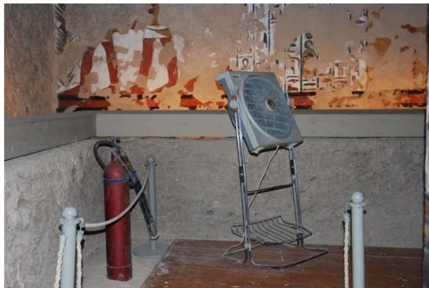
Fire extinguisher and fan for air circulation in lower chambers.
