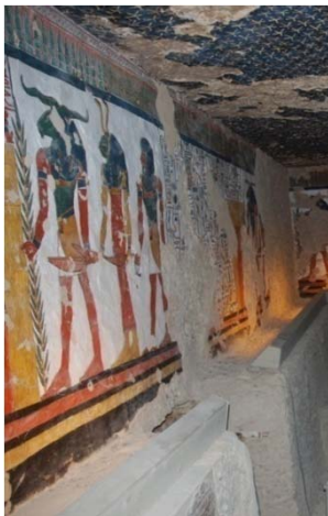
Housing for fluorescent lights on ledge in Chamber K (left), and on floor and ledge in Chamber C (right). Illumination is strong at source and falls off on upper parts of walls.
