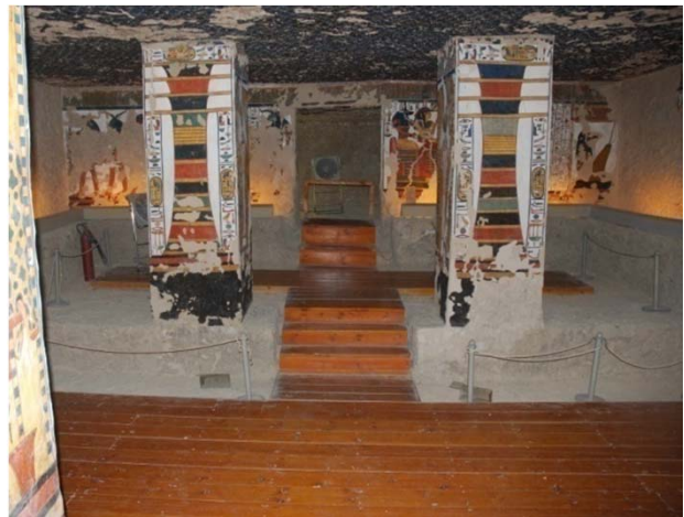
Wooden walkways and platform in Chamber K (foreground) leading to rear Chamber Q. The wooden walkways are in generally good condition, but are not of modular construction making it impossible to remove them to clean dust and lint below them.
