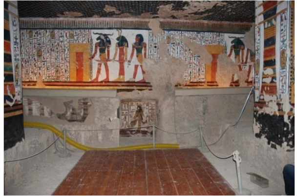
Lighting, stanchions and wooden platform in Chamber K. Note platform ends approx. 30cm from wall. Stanchions and platform function more as psychological than physical barriers. This system is viable because of the restricted number of visitors allowed at any one time in the tomb, but stanchions are unstable and potentially dangerous. Recommendations were made in the past to anchor the stanchions, which are at risk of being knocked over, to the walkways.
