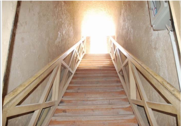
Wooden staircase and handrail constructed on the original stepped ramp (A)
