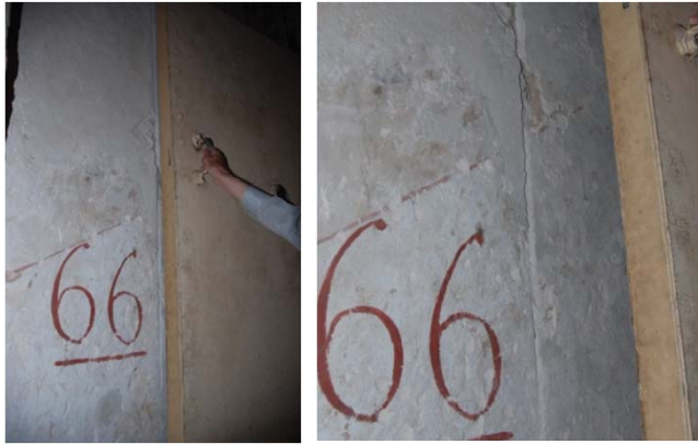
Impact of heavy metal door opening onto the wall of the stepped ramp (left and detail right). A method of preventing the door from hitting the wall is required.
