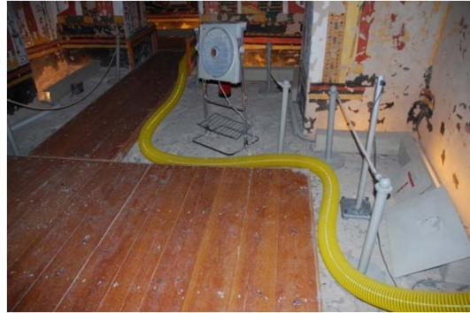
The broken ducts were replaced by new ducting throughout the tomb (yellow ducting in photos above).
