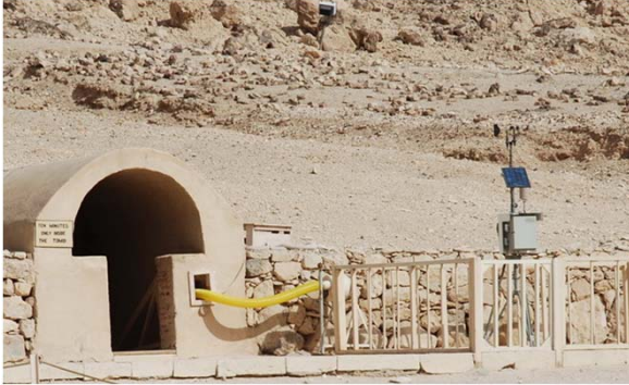
The broken ducts were replaced by new ducting throughout the tomb (yellow ducting in photos above).
