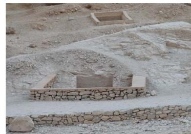
A retaining wall was constructed around the area of instability (above, arrow) in 2009. (Photo also shows new surrounds).
