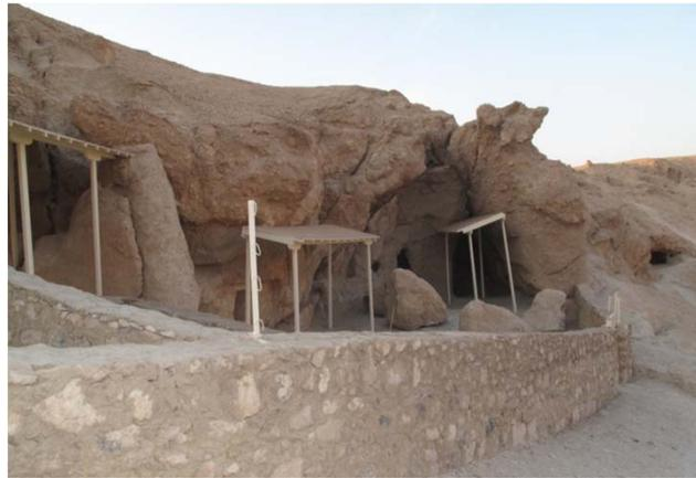
In 2010 a new perimeter wall with fencing was constructed following the line of an existing dry rubble wall along the path adjacent to the Sanctuary to Ptah and Meretseger. Shelters were then constructed to protect engraved stelae. The terrace wall within the sanctuary was also reconstructed.
