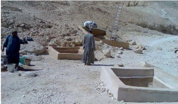
In 2009, new surrounds were constructed on some shaft tombs (QV 39 above) and existing surrounds were re-painted (e.g. left). Bricks for new surrounds were placed directly on loose soil (upper left) and therefore have little structural integrity. They will need to be replaced.
