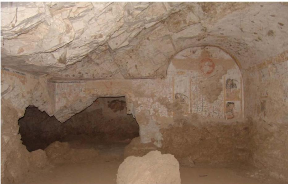
Chamber C with barrel vault (east wall) and structural collapse of ceiling and walls.
