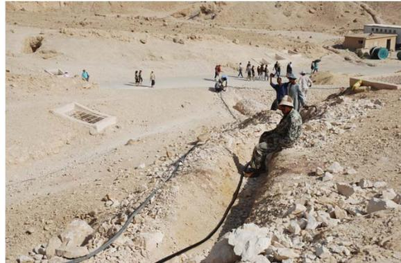
In 2010 trenching for installation of electrical cabling for lighting of the mountains was undertaken across the Valley near the generator building and continuing to the mountains.
