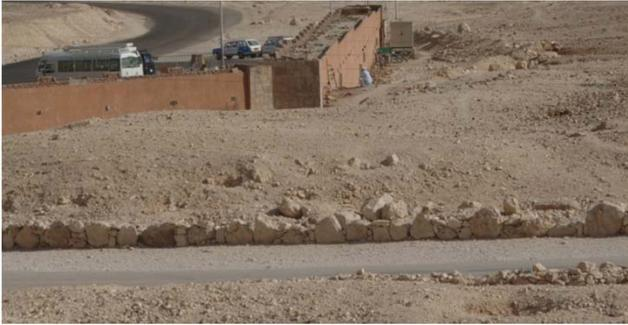
Rubble walls along the south side of main visitor path (left) were dismantled in 2007. New stone masonry walls were built in various stages and versions with painted, cement caps in 2008-2009 (below). Walls edging the SW wadi path were capped with cement (bottom left). The remaining area of tarmac road that constitutes the main path in the valley (seen in photo bottom right) was removed in 2010 (from the security station to the Y-Junction).
