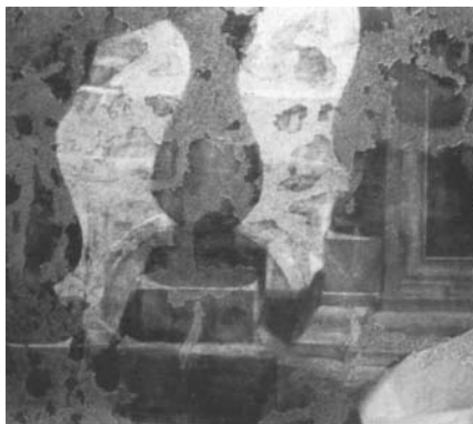
FIG. 9 Detail of balustrade after restoration. Note difference in level between the original layer and the reconstructed areas.
