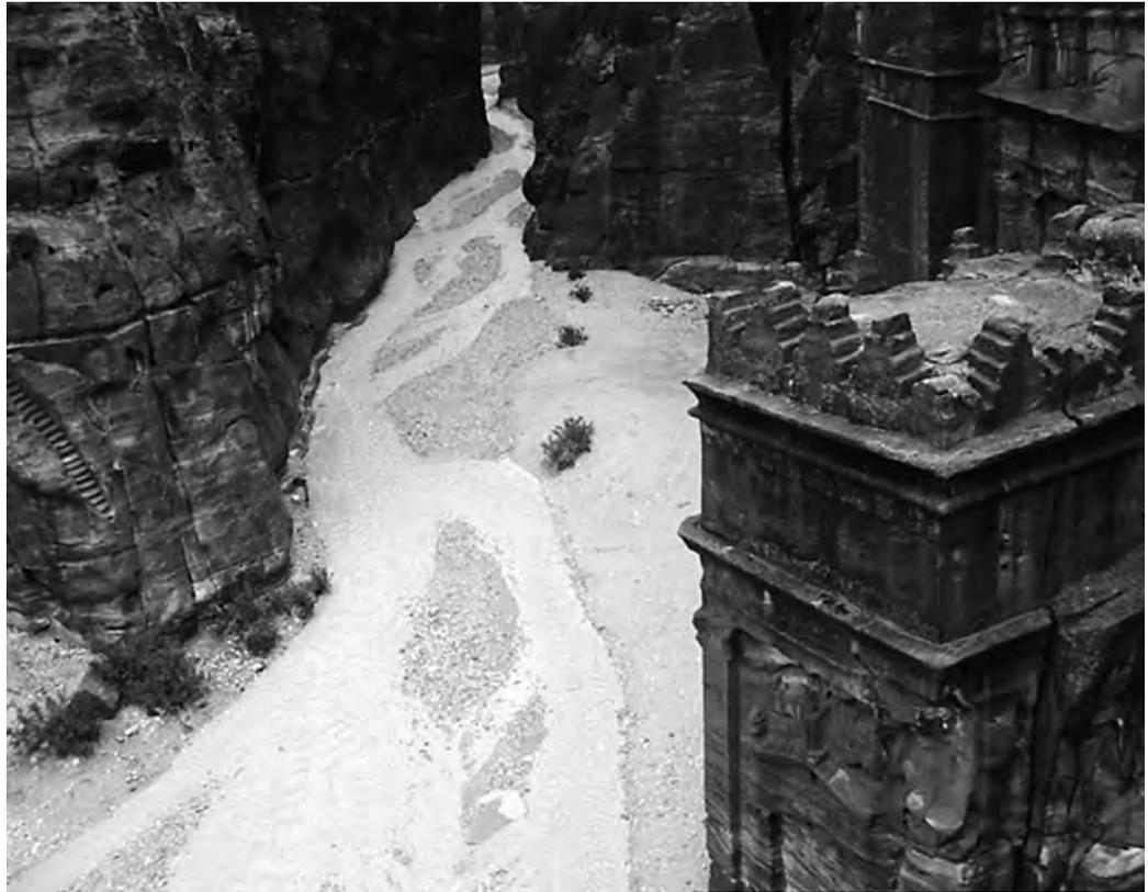
down the facades of tombs. Limestone dust from nearby highlands has settled on the exterior of the tombs, forming a hard but brittle crust. When water finds its way into cracks in the crust, it eventually wears away the softer sandstone beneath. The exterior, on which decoration has been carved, falls away.
