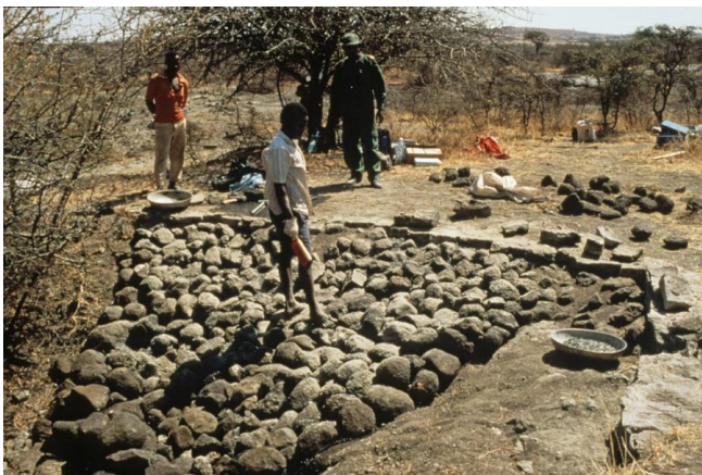
Gully stabilization near completion. Boulders were used to stabilize gully and prevent further erosion and loss of tuff.
