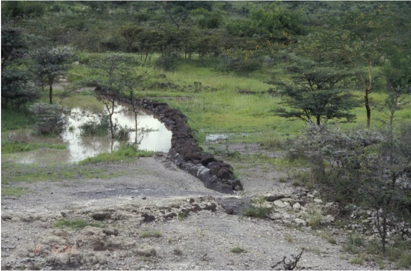
1996. Accumulation of water behind berm in rainy season, prior to completion of drainage plan.
