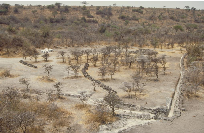
1996. Site-wide drainage was implemented to direct rainfall away from the trackway to the gully north of the site.
