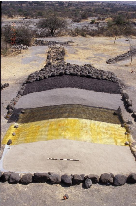
Partial profile of reburial stratigraphy: Layer 3, Biobarrier, Enkamat, Layers 4 and 5, and lava boulders.
