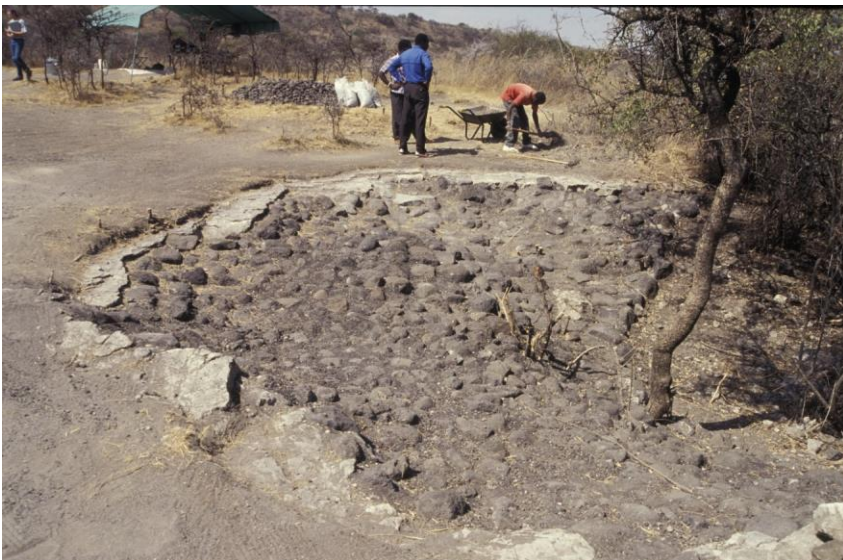
1996. West gully was stabilized in a manner similar to the NW gully.
