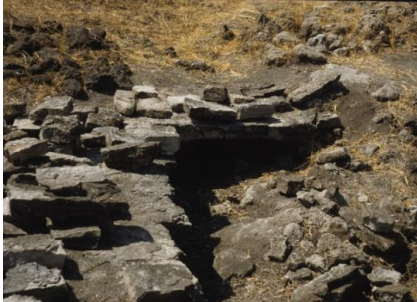
Re-attachment of four collapsed blocks, from left: fallen blocks placed on ledge near where they were found; placement of blocks in original position; re-attachment using fiberglass geo-rods and epoxy adhesive.
