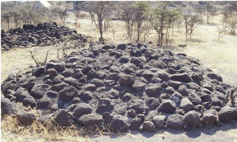
1995. Monitoring trench completed with boulder capping.
