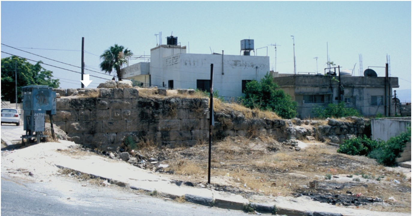
▲ View of a section of the ancient city wall (see arrow), in front of modern buildings. The modern city contains some of the best-preserved sections of the ancient city wall, some of which lie under modern construction. Photo: David Myers, GCI.
