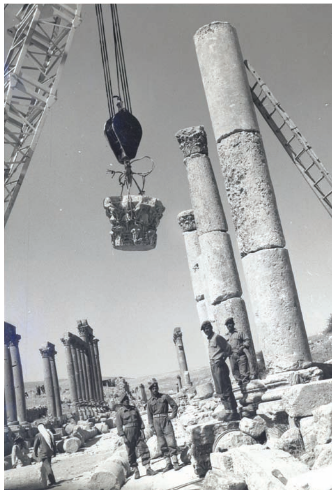
▲ Soldiers re-erecting columns along the Cardo. In the early 1960s, the Jordanian army's Royal Engineering Forces became involved in restoration work at the site. Photo: Department of Antiquities of Jordan.
