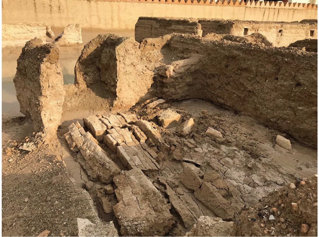
FIGURE 9.4. View of a structure at Hili 2, Al Ain, United Arab Emirates (UAE), showing a collapsed wall following a heavy downpour. Source: Aqeel Ahmed Aqeel, DCT Abu Dhabi.
