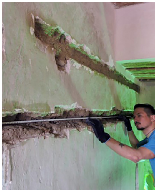
FIGURE 7.17. Stitching of cracked earth block masonry with fiberglass bars (a). The arrangement of the needles should be staggered (b). Source: ZRS, Christof Ziegert.
