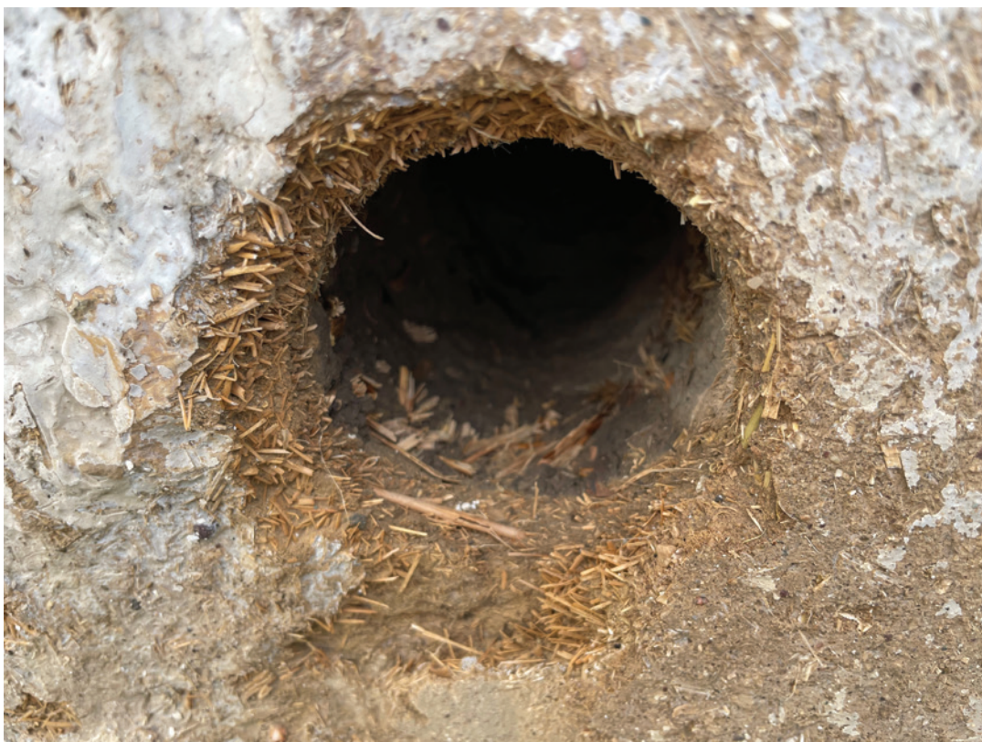
FIGURE 8.3. The different fibers of the base and top plaster can be seen in the core drilling. While the base coat contains coarser straw fibers, fine flax shives are visible in the top coat. Source: ZRS, Christof Ziegert.
