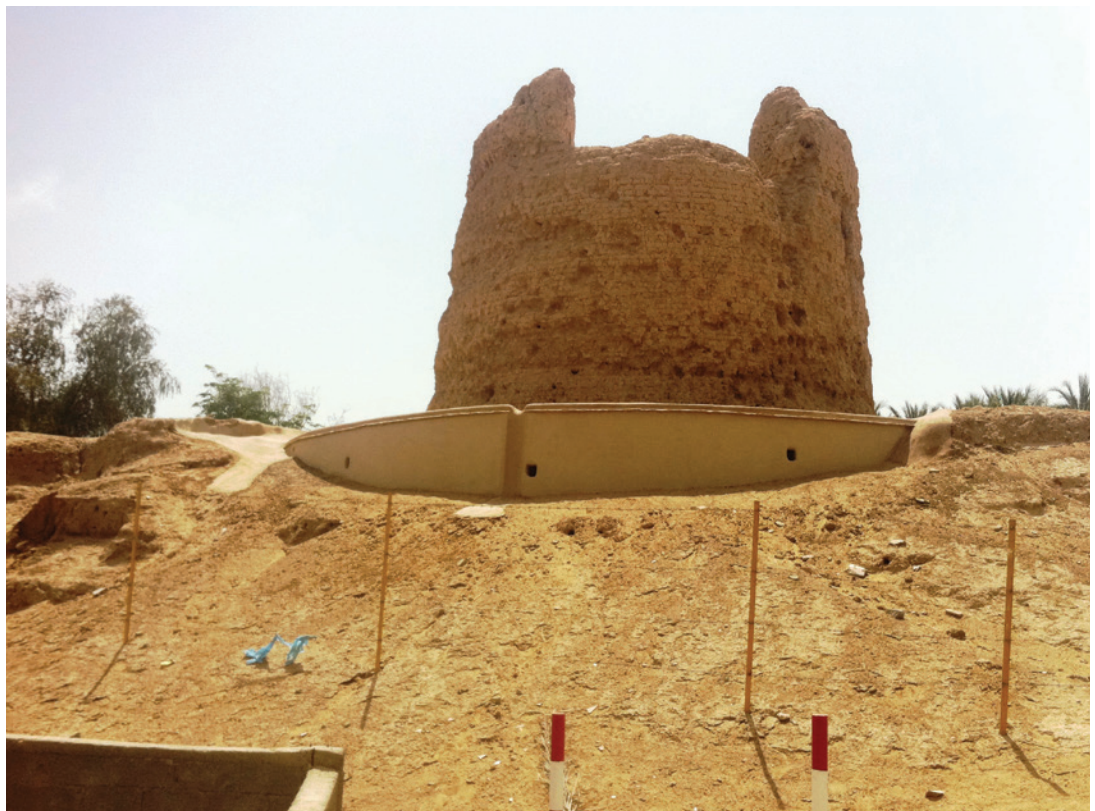
FIGURE 11.4. Daramkah Tower, Al Ain, after building the wall buttress. Source: DCT Abu Dhabi.
