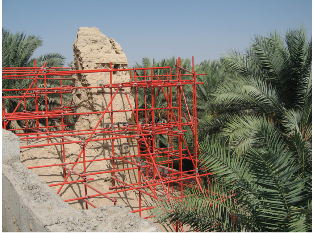
FIGURE 11.1. Scaffolding structural supports around Bin Suroor Southern House in Al Ain. Source: DCT Abu Dhabi.
