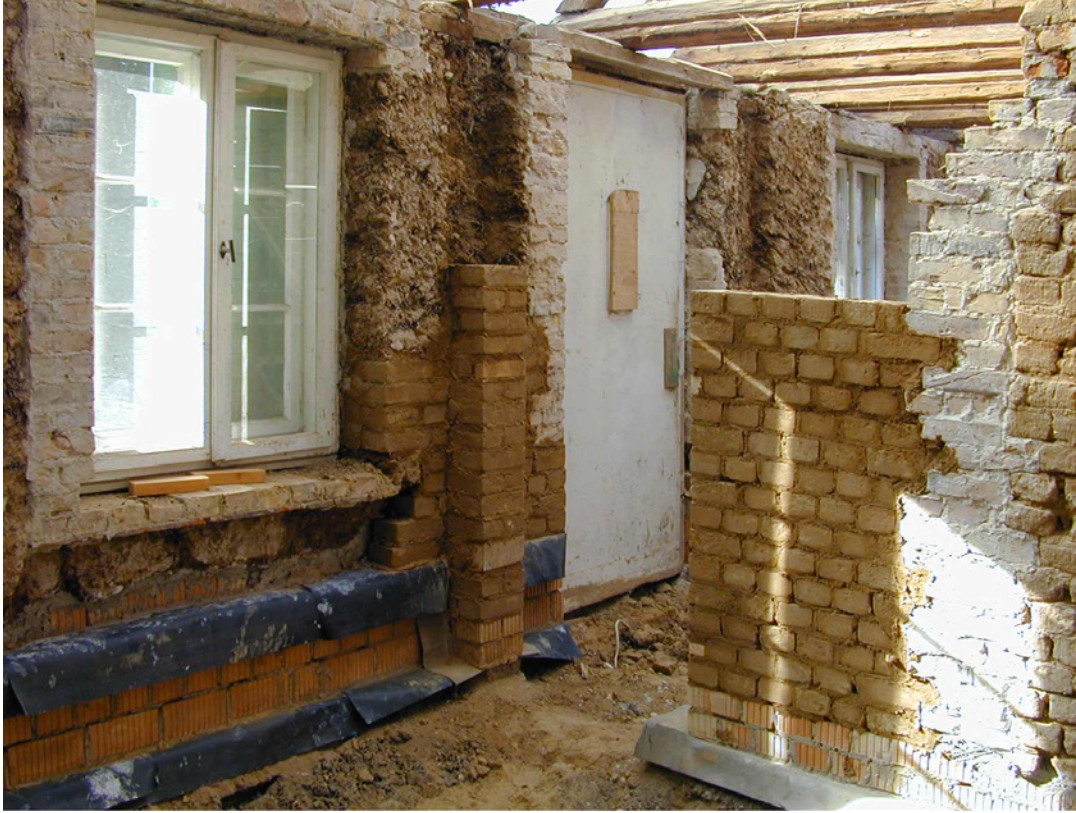
FIGURE 7.12. Small residential building in Germany in which the damaged plinth in the splash water area (up to 30 cm above ground level) was replaced with mud bricks. Source: ZRS, Christof Ziegert.
