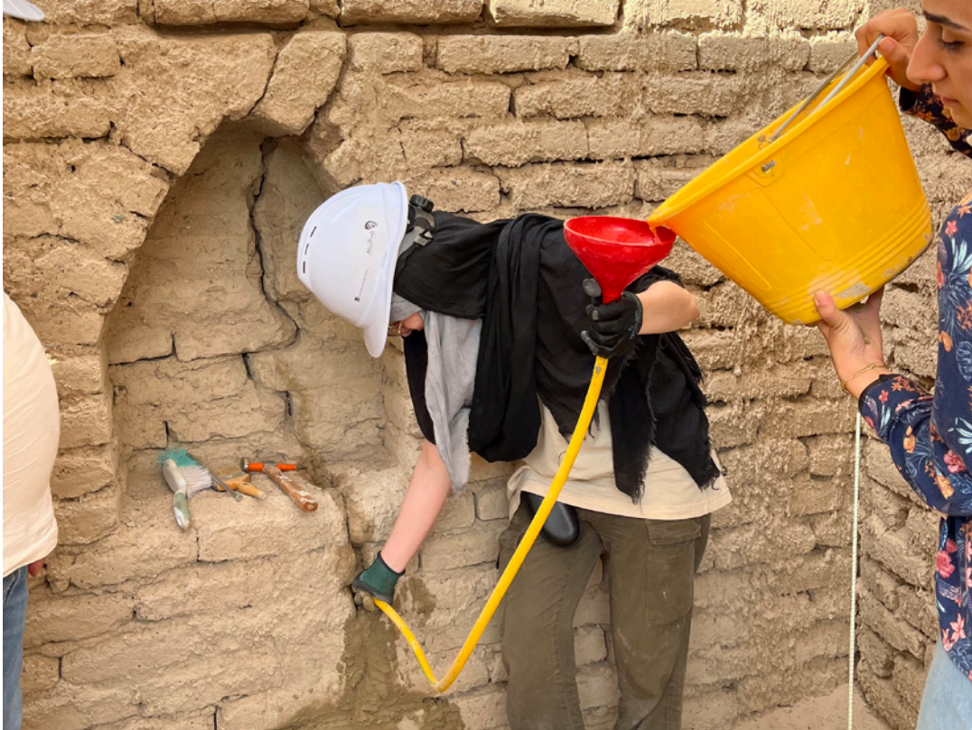
FIGURE 7.15. Example of gravity-fed grouting of an earthen wall using an earthen grout with sand aggregate. Source: Benjamin Marcus.
