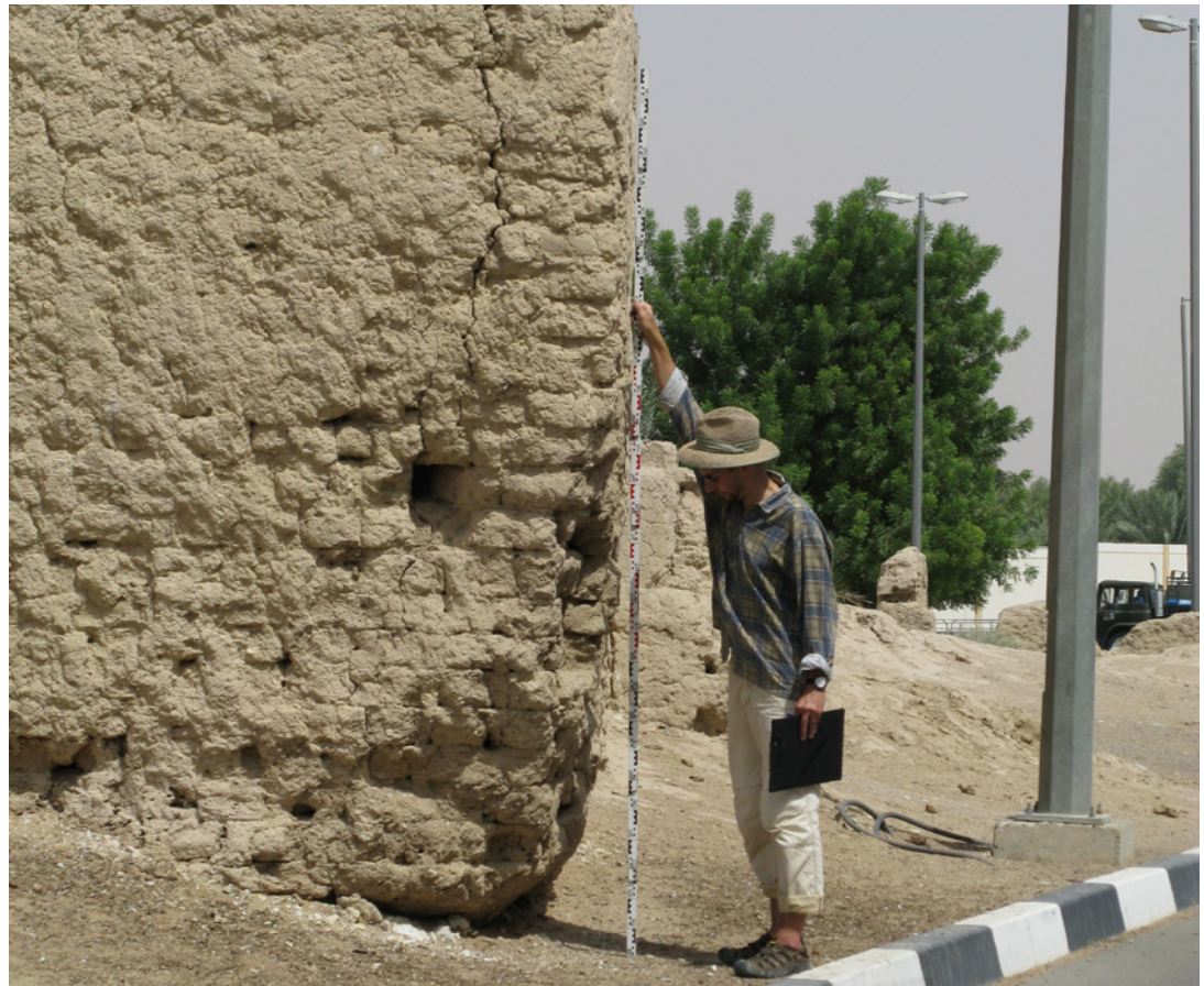
FIGURE 7.1. Structural assessment of a threatened earthen building with a serious crack directly on a public area, Al Ain, United Arab Emirates (UAE). Source: ZRS, Christof Ziegert.
