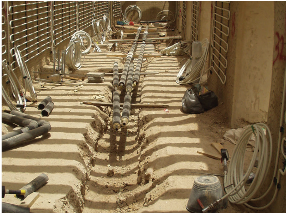
FIGURE 10.13. View of the temporary exhibition space at Al Jahili Fort during installation of the cooling system and MEP. Source: DCT Abu Dhabi.
