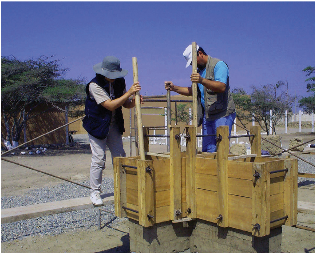
FIGURE 3.15. Traditional formworks use a combination of wood and attachment elements including metal anchors. Source: Wilfredo Carazas Aedo.
