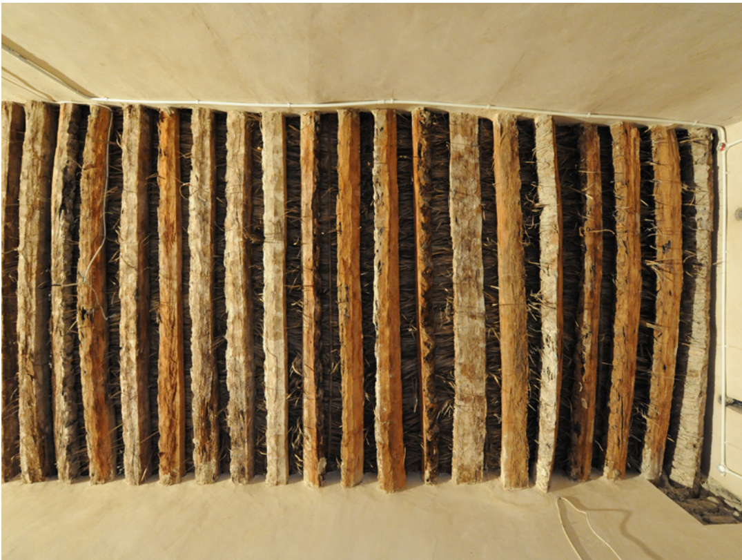
FIGURE 7.36. Looking up at the ceiling in Al Jahili Fort, showing the palm beams from the interior. Source: Aqeel Ahmed Aqeel, DCT Abu Dhabi.
