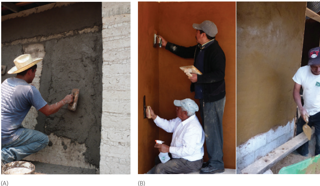
FIGURE 3.33. (a) A technician creates an initial base layer of earthen plaster on a wall. (b) Technicians apply the second, refining layer of plaster to a wall. Source: Wilfredo Carazas Aedo.
