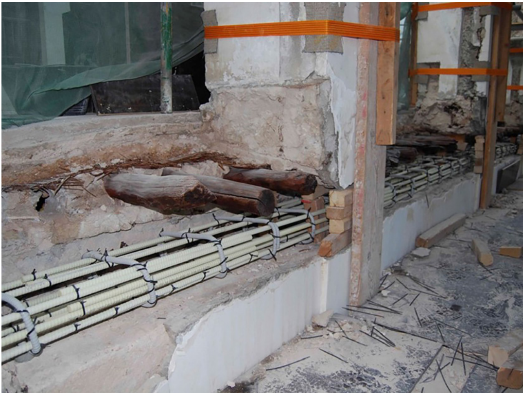
FIGURE 7.21. A ring beam in fiberglass to be filled in with lime mortar. Old Palace, Doha, Qatar. Source: ZRS, Christof Ziegert.
