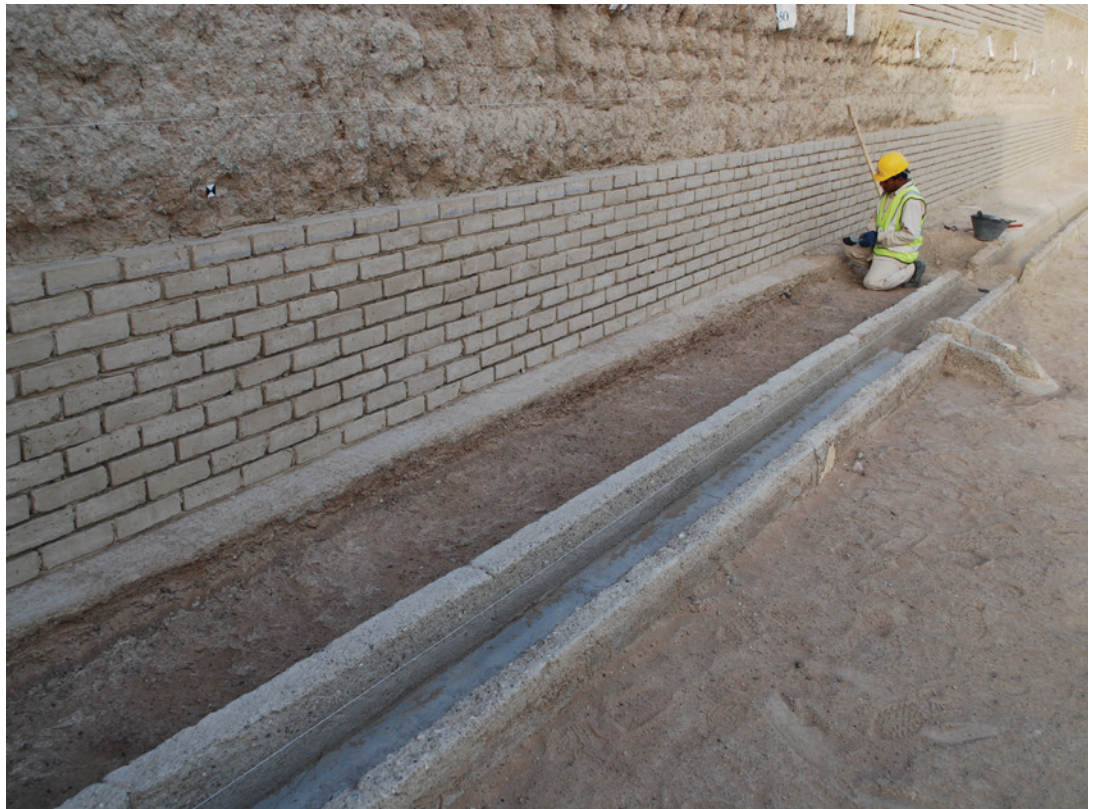
FIGURE 10.22. Reintegration of the mud bricks in the base of the walls. The adjacent traditional water channels are cleared and ready for consolidation. Source: DCT Abu Dhabi.
