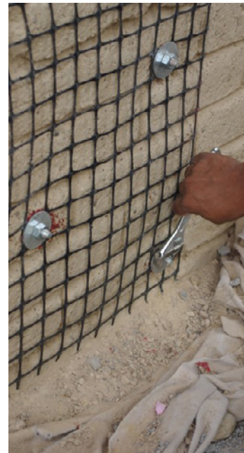
FIGURE 7.18. A polypropylene geomesh wrap is anchored to an entrance at Muwajji Fort, Al Ain, to strengthen the union of original nineteenth-century masonry and earth blocks added later during restorations in the twentieth century. Source: ZRS.
