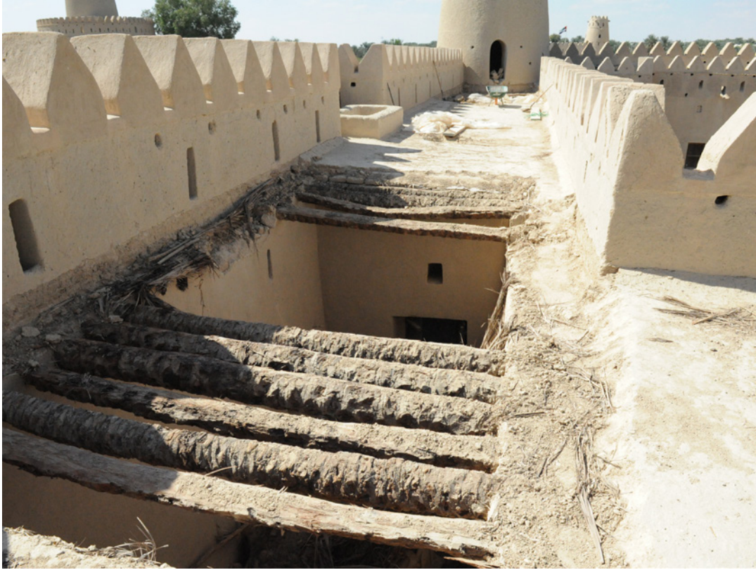
FIGURE 7.35. A closer look at the layers of the roof at Al Jahili Fort before restoration: after removing the layer of mud and palm branches, the beams were exposed. The rectangular opening leading to the water spout can be seen in the background. Source: Aqeel Ahmed Aqeel, DCT Abu Dhabi.
