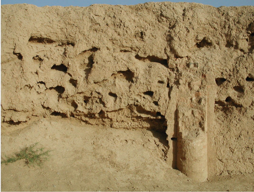
FIGURE 9.3. Portion of a wall at Nisa, Turkmenistan, showing cracks and holes in the exposed surface in which birds have nested. Source: Gaetano Palumbo.
