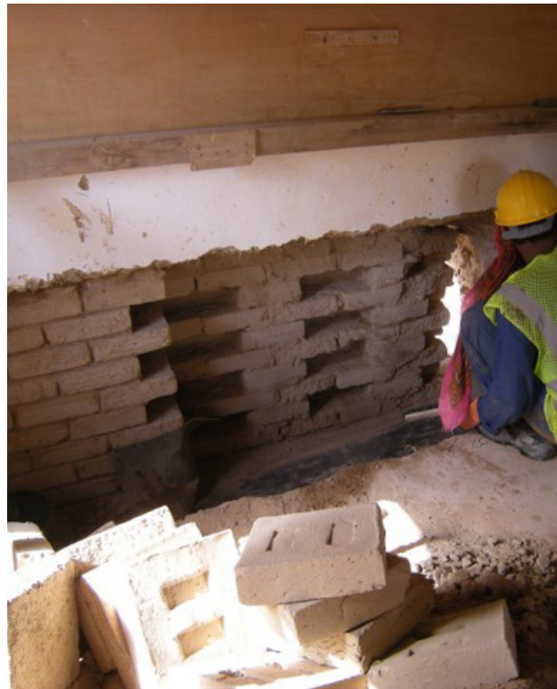
FIGURE 7.13. Muwajji Fort, Al Ain, with replacement of the material over the entire cross section and installation of a horizontal moisture barrier. Source: ZRS, Christof Ziegert.
