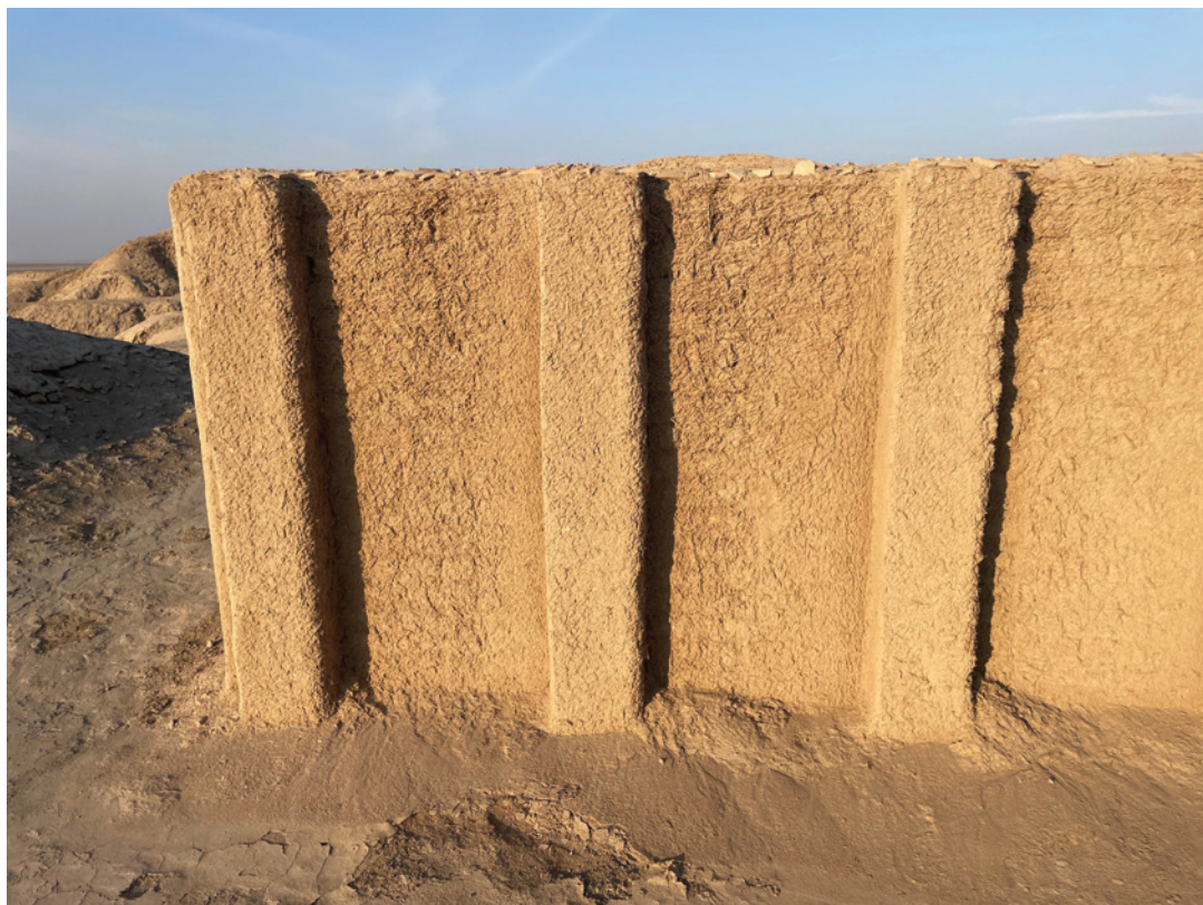
FIGURE 8.4. The earth plaster has weathered to such an extent that the structure of the earth blocks is visible. Further rainfall would erode the earth blocks. This is therefore a critical time to apply a new layer of plaster. Source: ZRS, Christof Ziegert.
