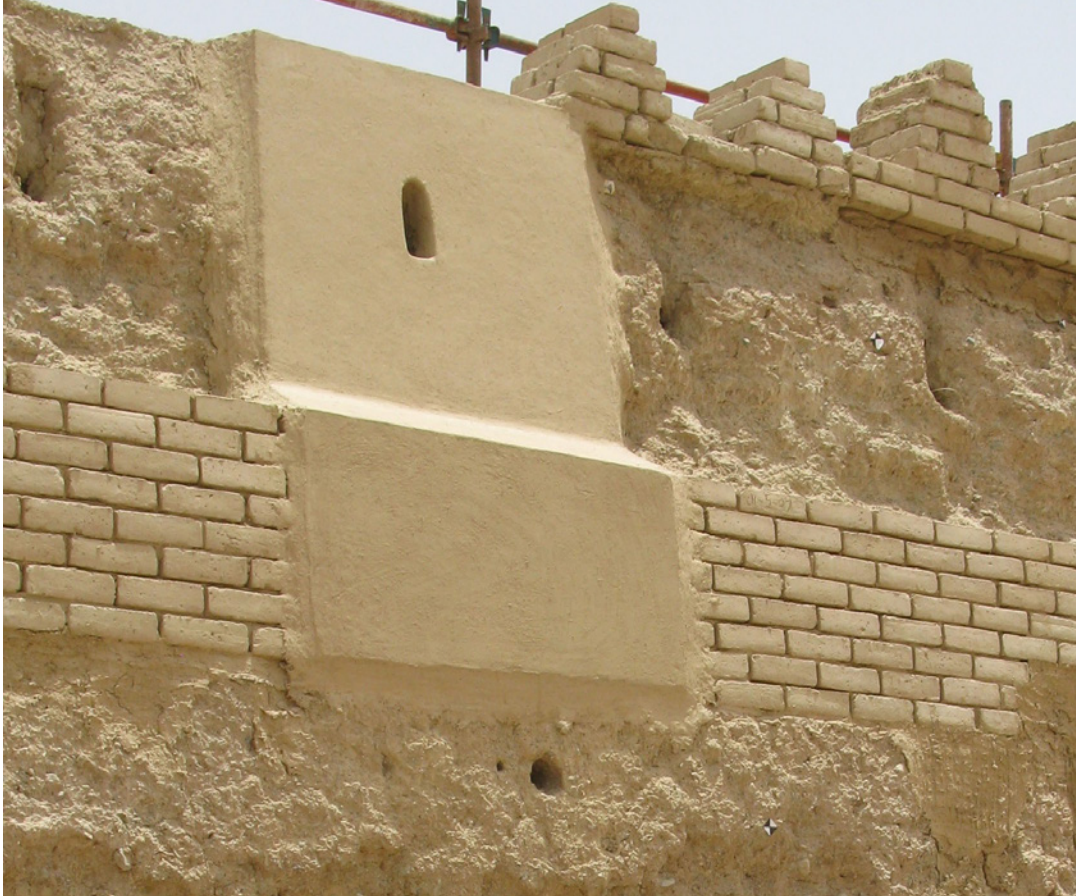
FIGURE 7.6. Muwajji Fort, Al Ain, after removal of damaged plaster, preparation of the surface, and reintegration of losses. Source: ZRS, Christof Ziegert.
