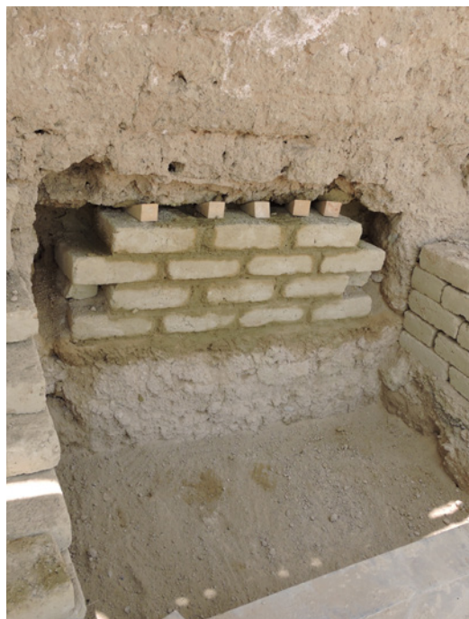
FIGURE 7.9. Al Muwaiji Fort, Al Ain, with stepped removal of damaged material (a). Al Jahili Fort courtyard wall, Al Ain, with area of eroded wall base removed at right angles and partial repair in place (b). Source: ZRS, Christof Ziegert.
