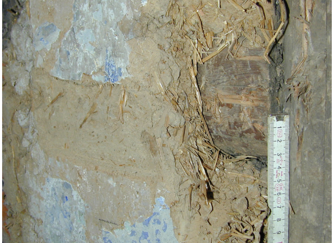
FIGURE 8.10. Detail of earthen plaster layer in an indoor application. The long straw in the plaster base can also be used to bridge wider timbers in the plaster base. Source: ZRS, Christof Ziegert.
