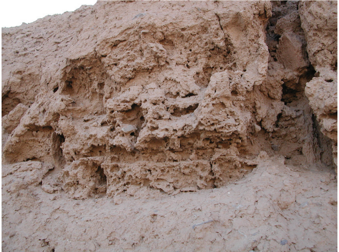
FIGURE 9.1. View of a portion of the exterior wall of the ancient city of Nisa, Turkmenistan, showing evidence of wind and water erosion. Source: Gaetano Palumbo.
