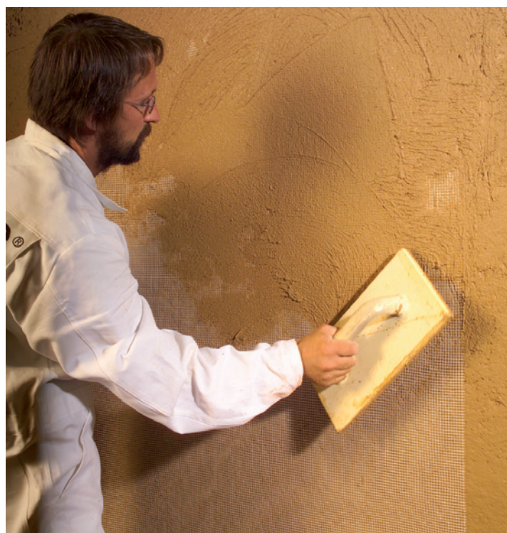
FIGURE 8.11. Insertion of flax fiber mesh. Source: CLAYTEC.
