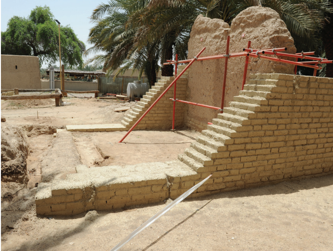
FIGURE 11.2. Freestanding wall at Bin Biduwa House, Al Ain, supported by the partially reconstructed walls. Source: DCT Abu Dhabi.
