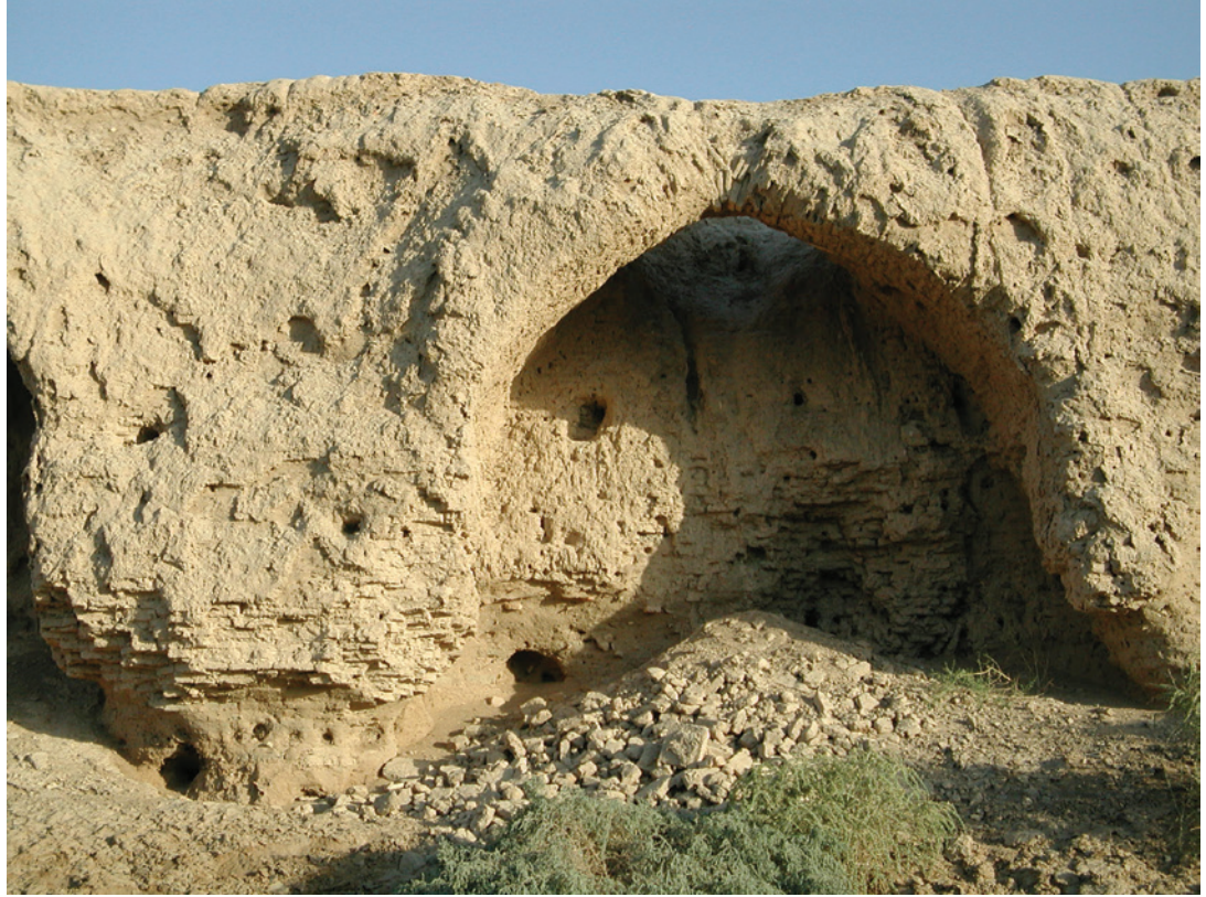
FIGURE 9.11. Portion of the walled city of Abdullah Khan Kala, Merv, Turkmenistan, showing damage to the foundation at the base of the wall caused by rising damp. Source: Gaetano Palumbo.
