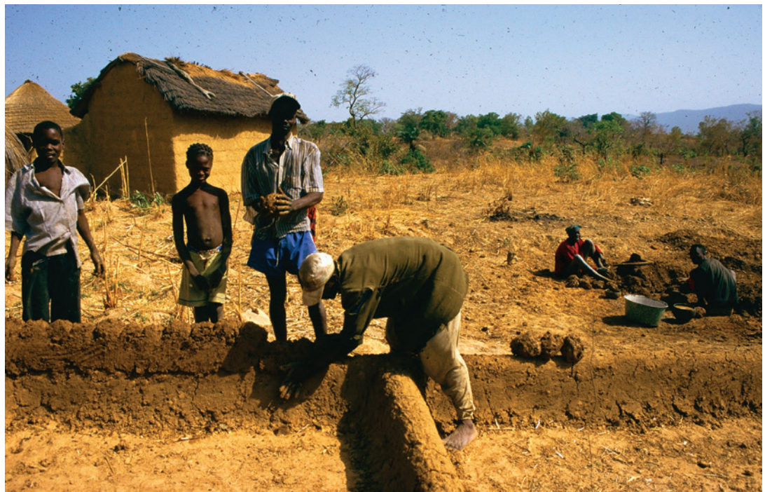
FIGURE 3.26. Traditional cob construction, West Africa. Source: Wilfredo Carazas Aedo.
