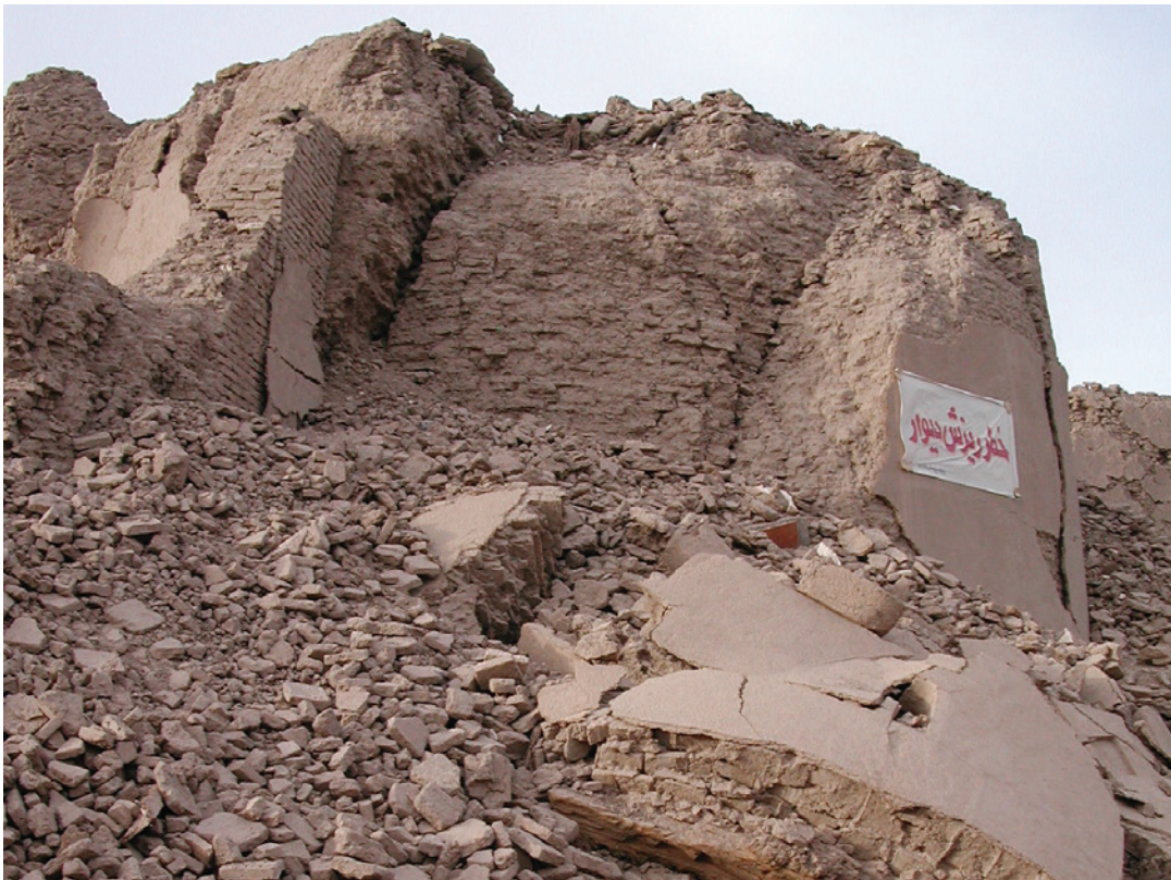
FIGURE 9.10. View of damage at Arg-e Bam, Iran. The outer layer of this tower, a modern addition, collapsed following the 2003 earthquake. Source: Gaetano Palumbo.
