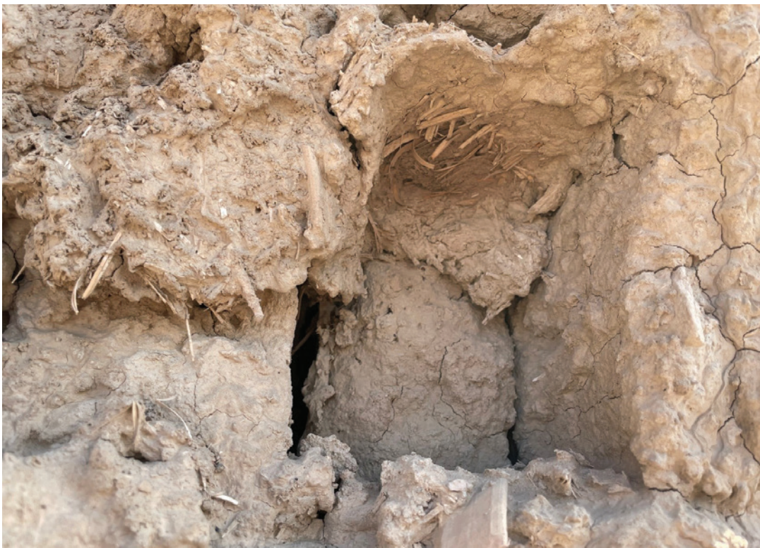
FIGURE 8.1. Historical earthen plaster made of earth and fiber. Source: ZRS, Christof Ziegert.
