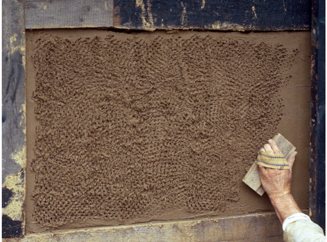
FIGURE 8.7. Combing of earthen plaster substrate layer before plaster application. Source: ZRS.
