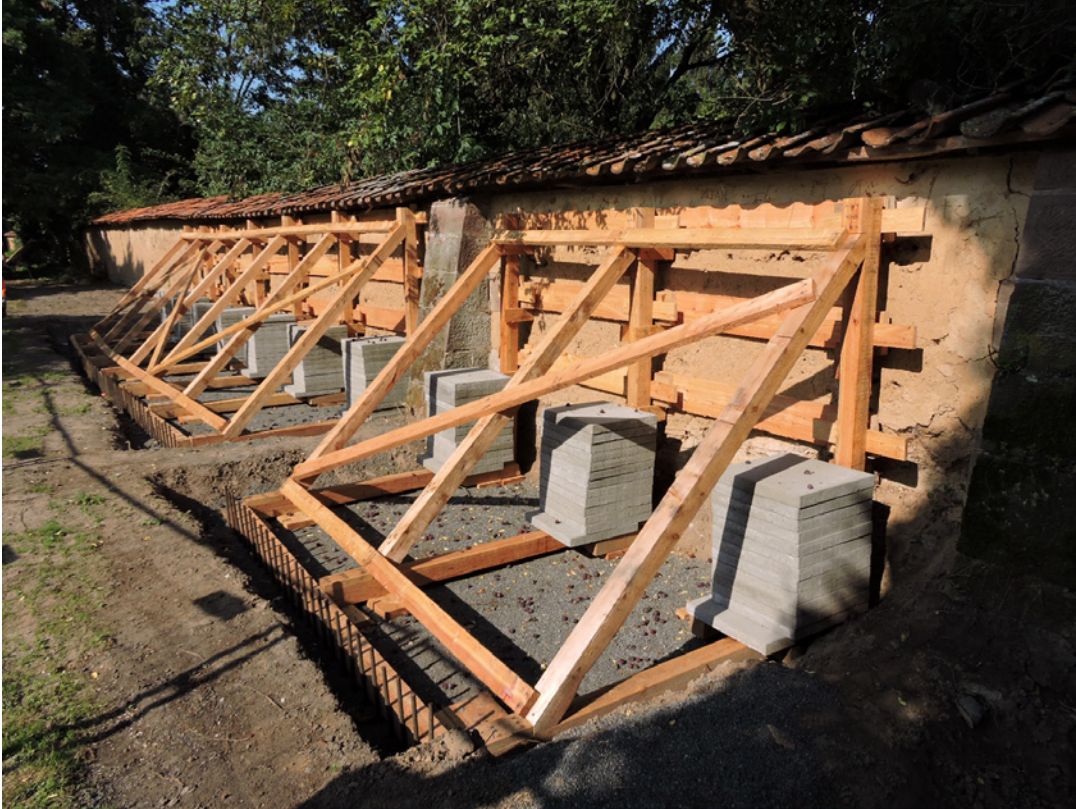
FIGURE 7.23. Timber system for an unstable earthen wall in Germany. Source: ZRS, Christof Ziegert.
