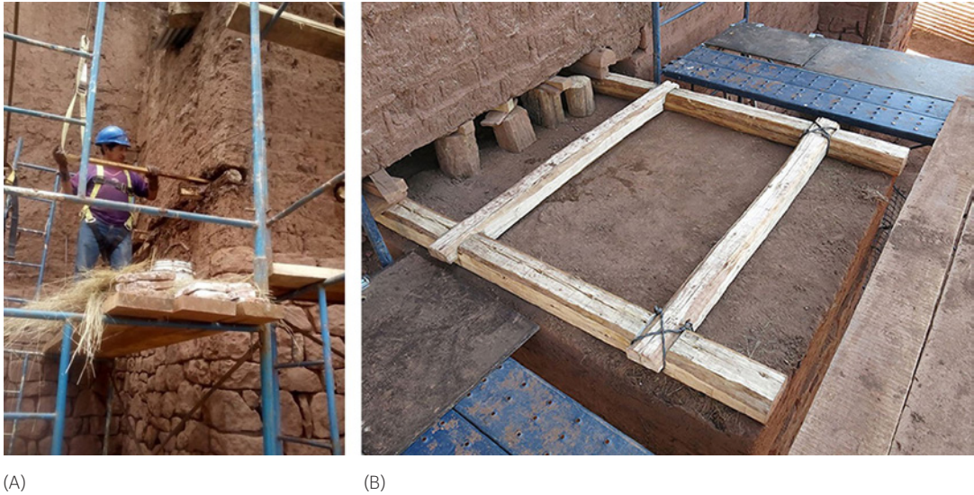
FIGURE 7.48. Images from the strengthening and rehabilitation project at the church of Kuñotambo: (a) integration of timber keys in new adobe buttress; (b) workers implementing the system of tie beams and bond beams into the church walls. Source: University of Minho for the J. Paul Getty Trust and Ministry of Culture.
