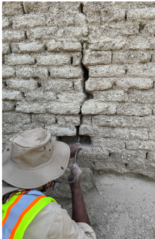
FIGURE 7.16. Stitching of cracked earth block masonry with earth blocks at the Murabb'a Fort Tower, Al Ain, UAE. Source: ZRS, Christof Ziegert.
