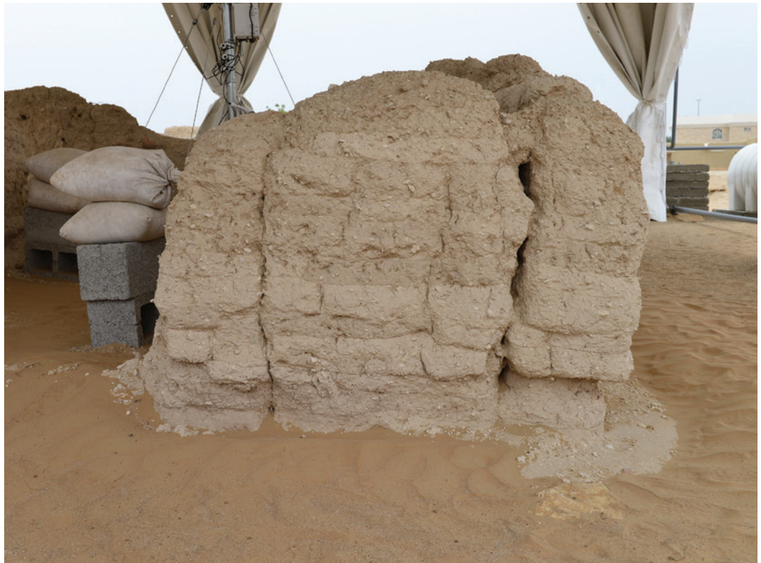
FIGURE 9.2. View of Hili 2, Al Ain, an Iron Age archaeological site, showing a vertical separation in the wall of a residential building. Source: Gaetano Palumbo.
