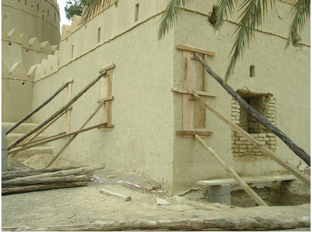
FIGURE 10.12. Photo of the south wing of Al Jahili Fort. Supports were installed to stabilize the corner walls while the foundations were reinforced underground. Source: DCT Abu Dhabi.
