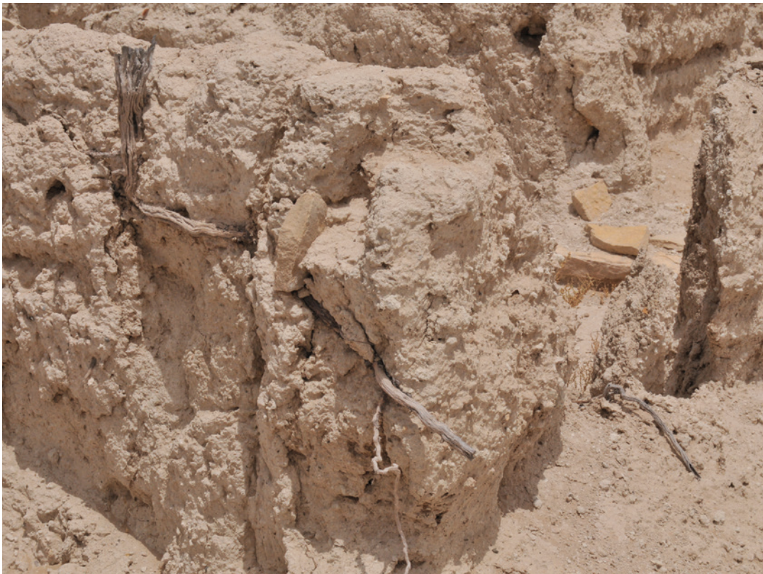
FIGURE 9.7. Roots embedded in a wall at Hili 17, Al Ain, UAE. As the vegetation continues to grow, the roots may weaken the entire structure. Source: Gaetano Palumbo.
