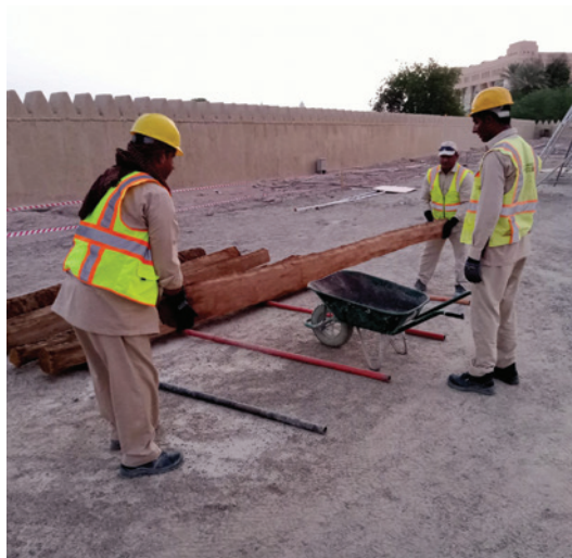
FIGURE 7.38. Prior to installation in a building, the wooden elements are chemically treated to prevent termite infestation: they are first soaked in a chemical bath for a day and then dried for about three weeks depending on climatic and environmental conditions. Source: DCT Abu Dhabi.
