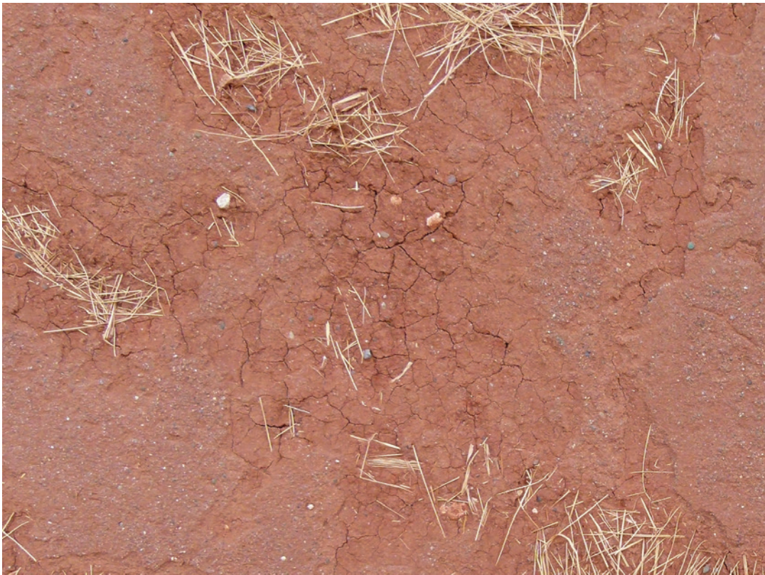
FIGURE 8.17. Detail of figure 8.20 showing the lack of cohesion of a weathered wall from a private house in Peru. Source: Clemencia Vernaza.
