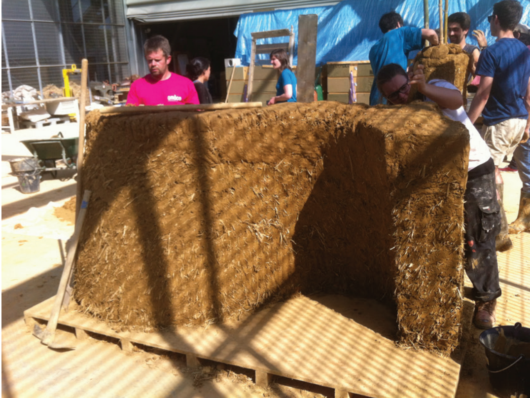
FIGURE 3.27. Traditional cob wall, Europe. Source: Wilfredo Carazas Aedo.
