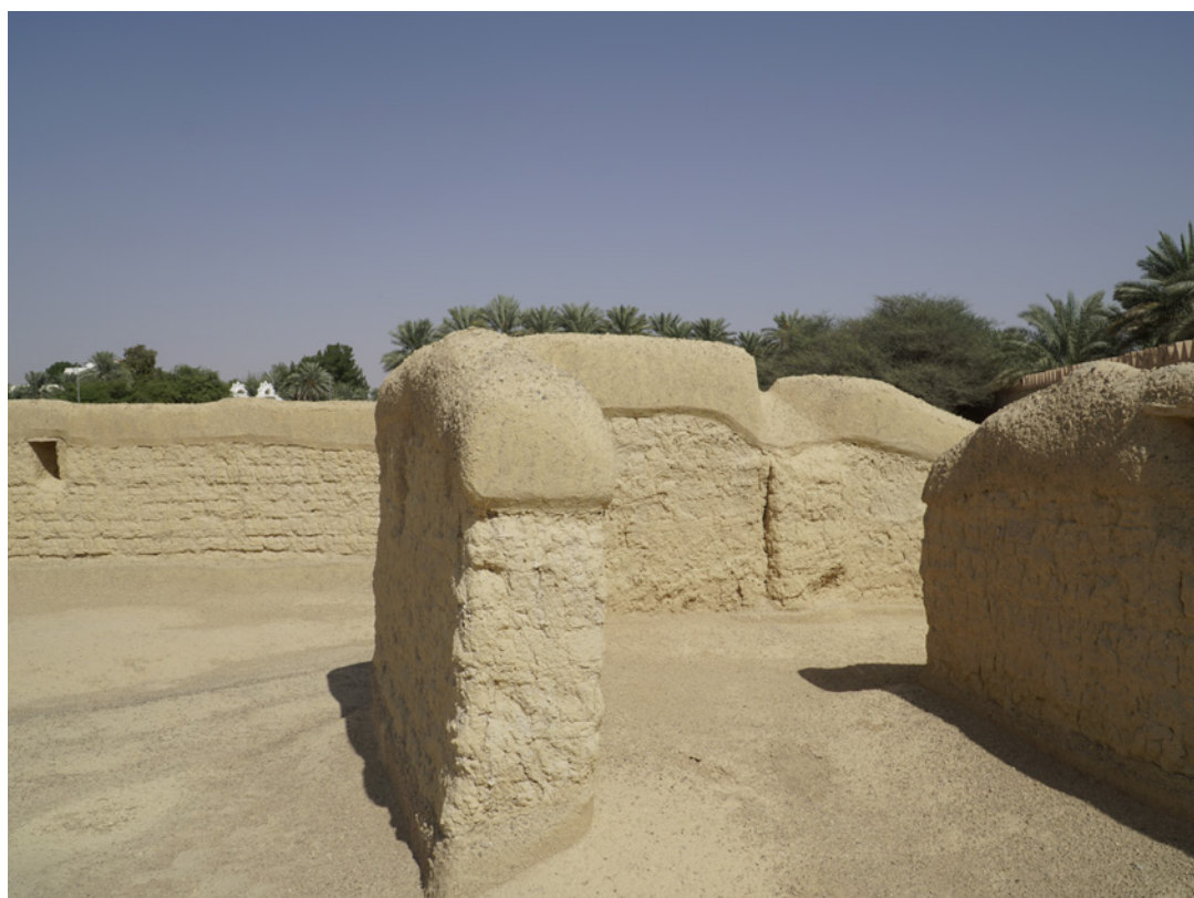
FIGURE 8.5. Earthen plaster sacrificial coating and capping on an archaeological site. The different color tones of the wall and the capping are problematic. With erosion, the color of the supplementary mortar will become mixed with that of the existing material. Source: Alessandra Sprega.
