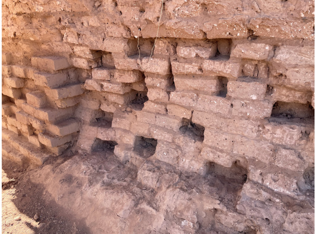
FIGURE 7.10. Regularly incorporated interlocks, where headers are inserted in the existing earth block masonry. Source: ZRS, Christof Ziegert.
