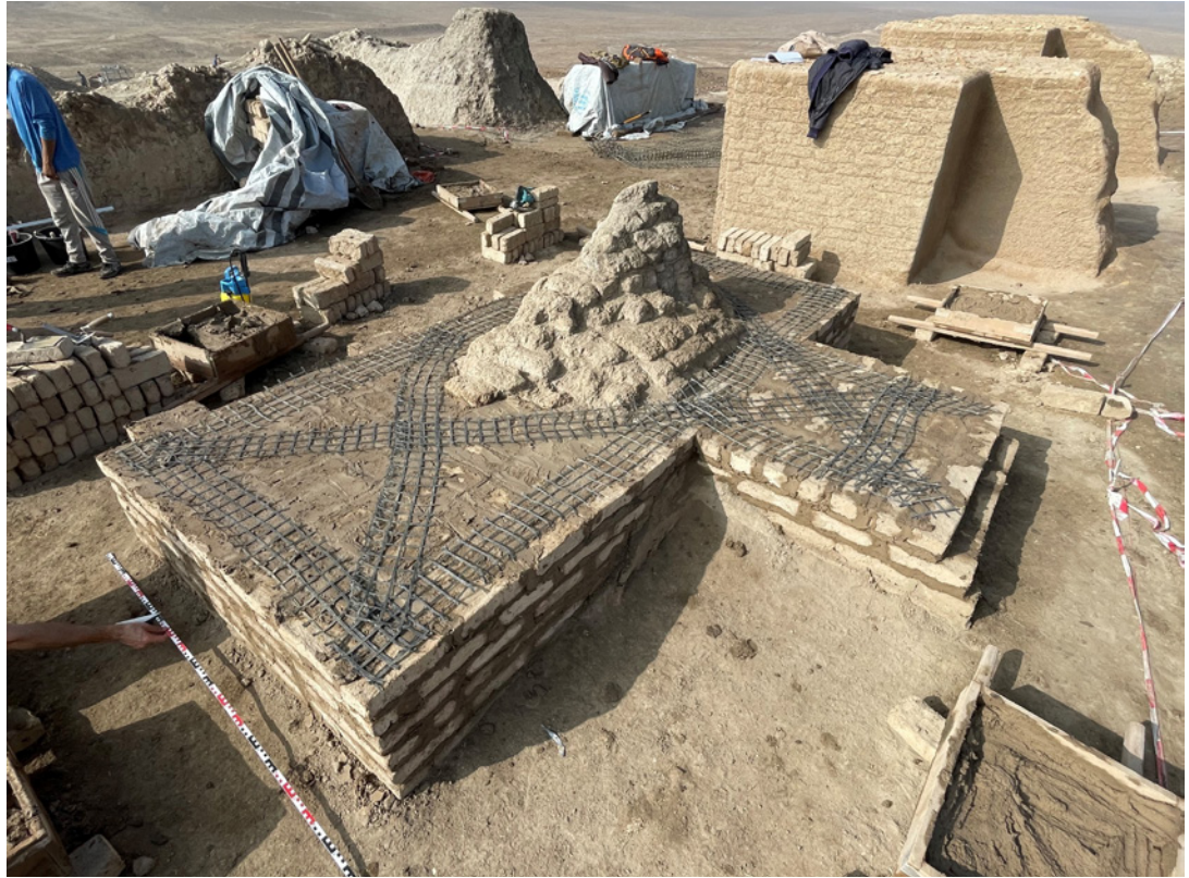
FIGURE 7.19. Horizontal reinforcement of the joints with geomesh strips. The positioning follows possible tensile stress orientations. The material is spread into the joint mortar. Protective masonry reinforcement at the White Temple in Uruk, 3500 BCE. Source: ZRS, Christof Ziegert.
