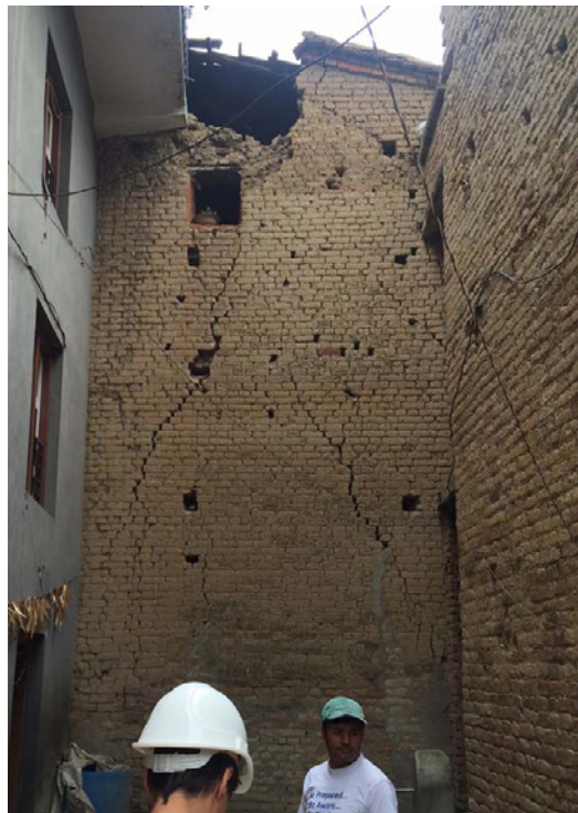
FIGURE 6.11. Cracks in solid earthen walls caused by different stiffness of materials and earthquakes. Source: ZRS, Christof Ziegert.
