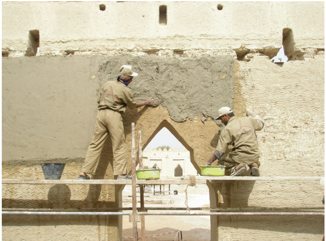
FIGURE 8.8. Application of earthen plaster on a masonry wall. Source: ZRS.
