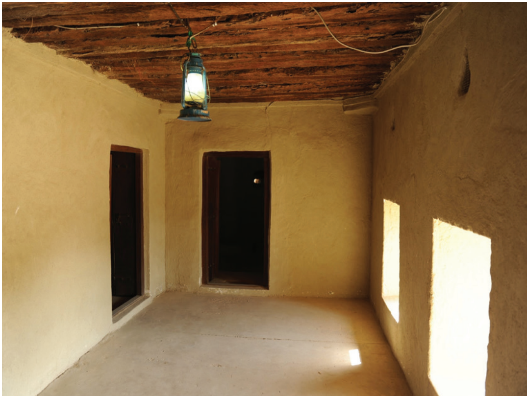
FIGURE 8.9. Earthen plaster in an indoor application. Source: ZRS, Christof Ziegert.
