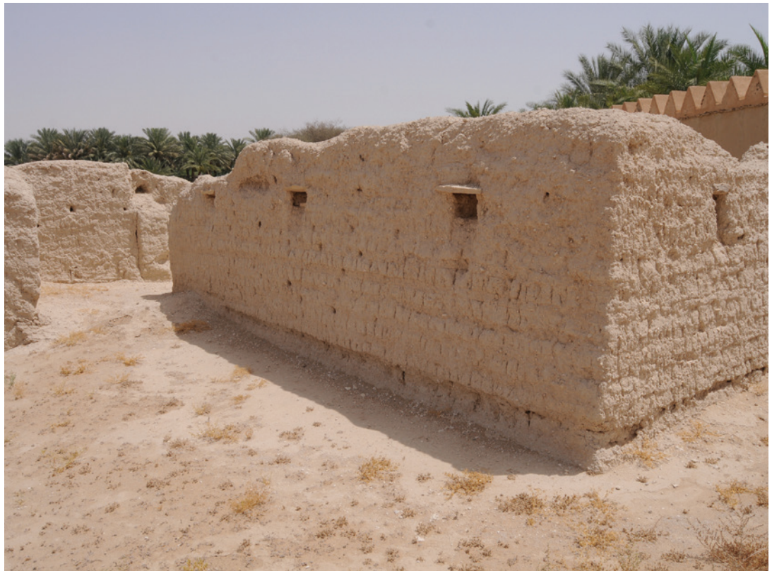
FIGURE 9.5. View of a structure at Hili 2, Al Ain, UAE. The bottom of the wall has been undercut by stagnant water and rising damp. Source: Gaetano Palumbo.
