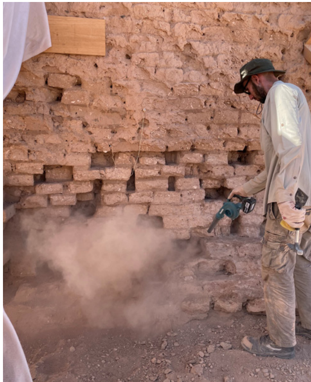
FIGURE 7.11. In addition to interlocking, (a) vigorous blowing off of the dust and (b) subsequent repeated gentle wetting are basic requirements for good bonding between the existing and supplementary masonry. Source: ZRS, Michelle Härder.
