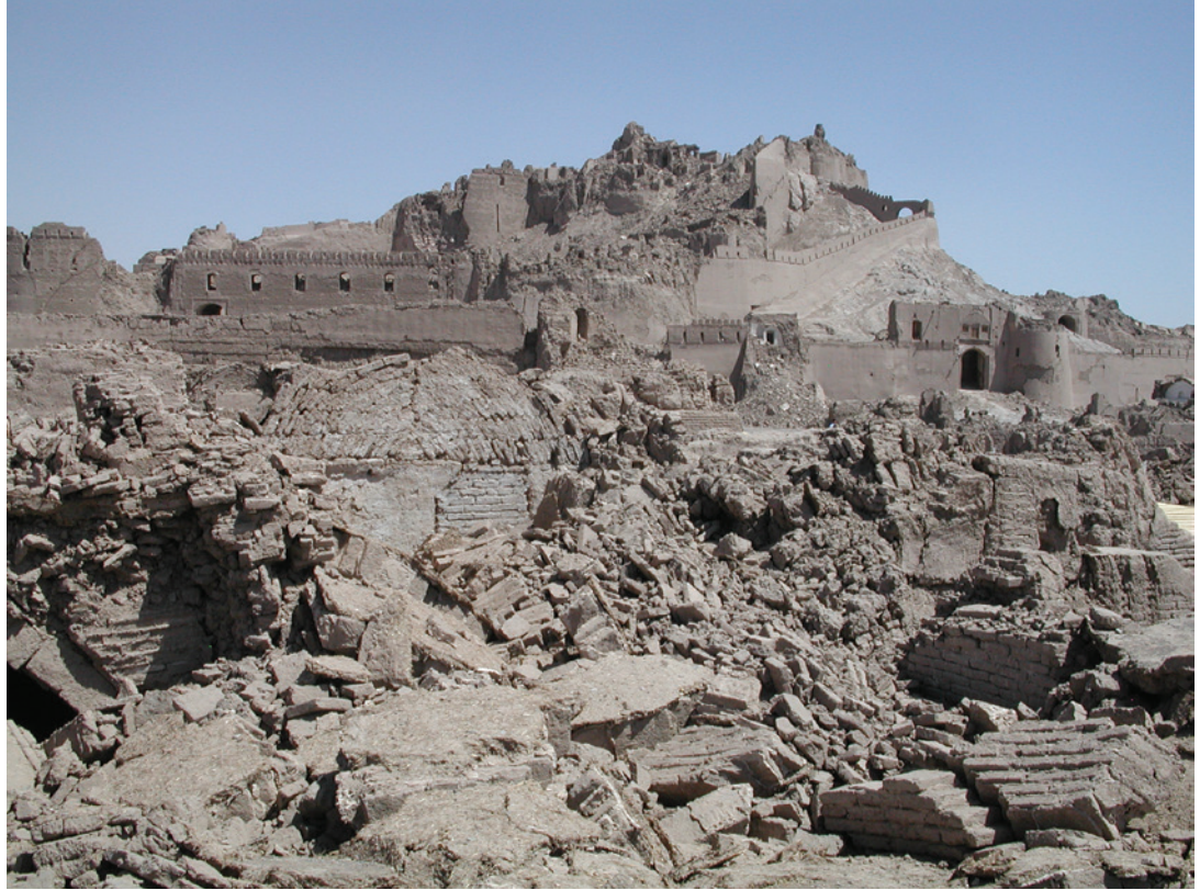
FIGURE 9.8. View of the earthen citadel at Arg-e Bam in Bam, Iran, showing extensive damage following a powerful earthquake in 2003. Source: Gaetano Palumbo.
