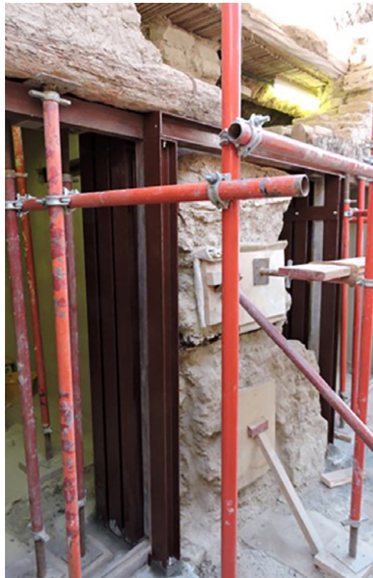
FIGURE 7.31. The slimline frame integrated for support blends in visually with the doorframe system. Al Ain, UAE. Source: ZRS, Christof Ziegert.
