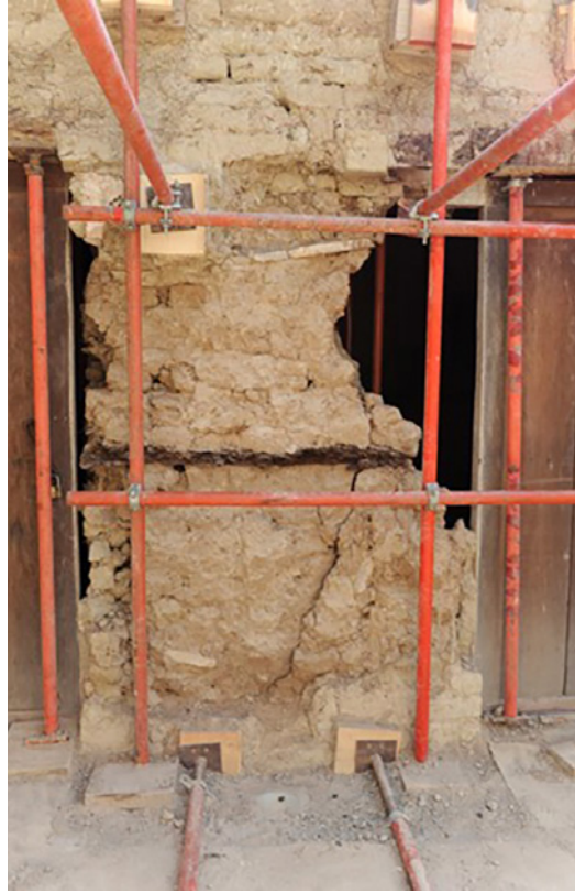
FIGURE 7.30. Collapsed masonry because of a flat-tened damaged lintel. Al Ain, UAE. Source: ZRS, Christof Ziegert.
