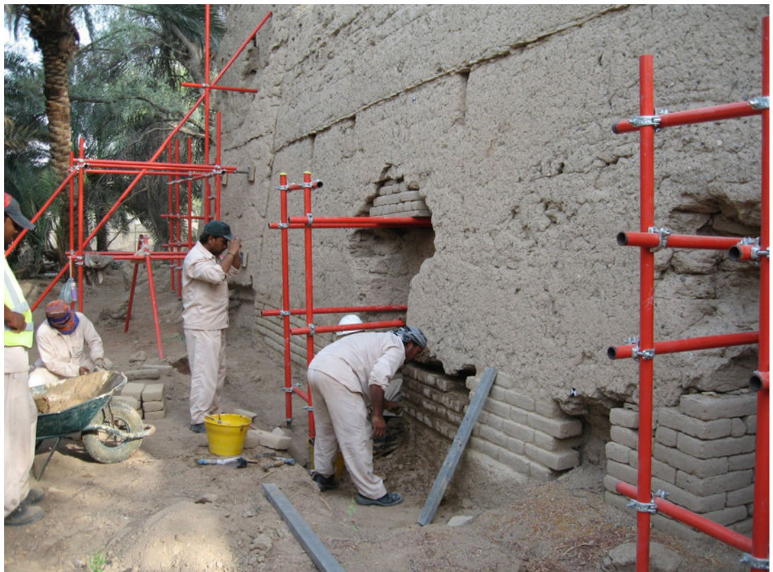
FIGURE 7.3. A team carrying out emergency shoring and basal erosion repair. Source: Benjamin Marcus.
