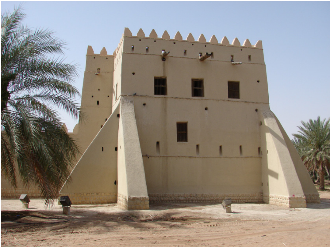
FIGURE 7.24. Historic mud-brick masonry buttresses at the North-West-Tower of the Muwajji Fort, Al Ain, UAE. Source: ZRS, Christof Ziegert.
