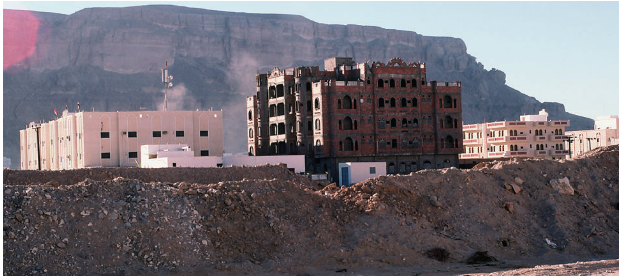
Modern concrete and block constructions in Wadi Hadhramaut. Photo: © Pamela Jerome.
