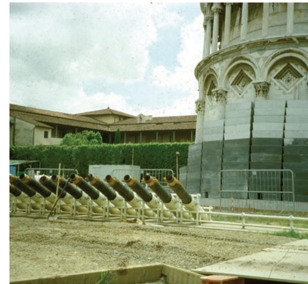
Lead weights were used to reduce the tower's lean. Photo: © Giorgio Croci.
