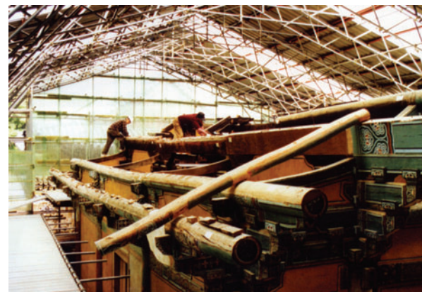
The Hall of Paradise, during restoration. Dismantlement of the temple allowed each building component to be documented individually. Photo: © Soon-Kwan Kim.
