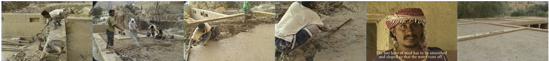
Series of stills from the documentary, showing the completion of a building. Workers are finishing off the new roof with mud. Photos: © Caterina Borelli.
