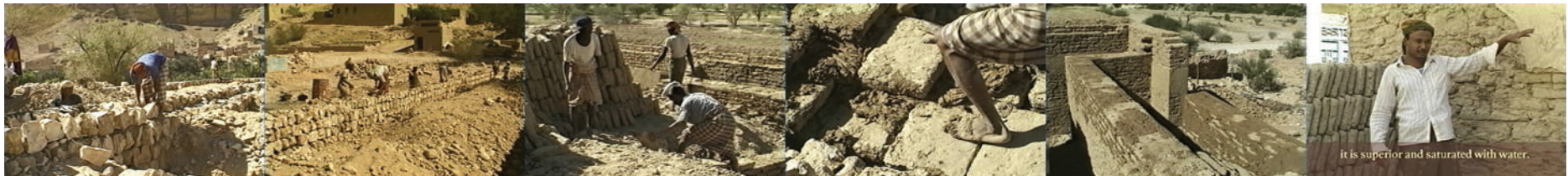
Series of stills from the documentary, showing workers erecting a new building. After the stone foundation is laid, the mud bricks are stacked to build a wall. Photos: © Caterina Borelli.
