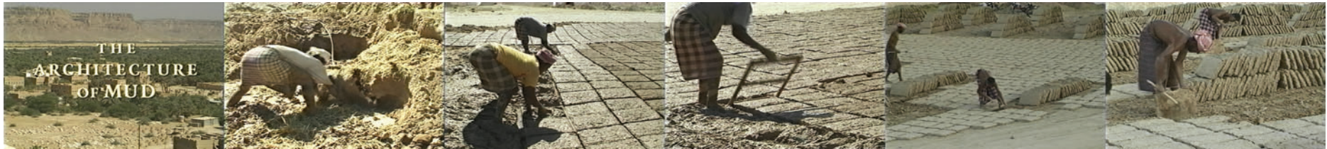
Series of stills from the documentary, showing workers in Seyoun creating mud bricks for new construction. Soil is gathered and mixed with straw and water. The mixture is spread out evenly in a mold, which is lifted immediately. The mud bricks are then left to dry in the sun for a week. Photos: © Caterina Borelli.
