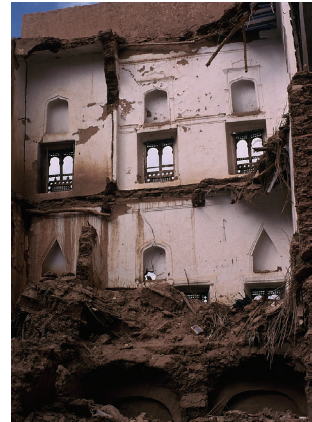
Abandoned historic building in Wadi Hadhramaut, in disrepair. Photo: © Pamela Jerome.
