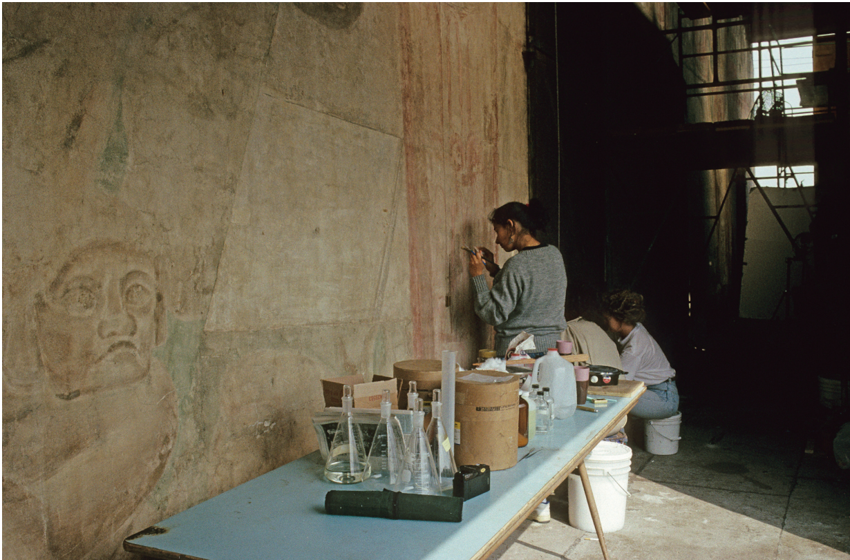
Figure 5 Conservation treatment of the mural. In 1990 a team of conservators led by Agustín Espinosa performed preliminary treatment, including surface cleaning, reattachment of plaster to the wall, removal of tar, and surface consolidation. Photo: Nancy Kaye, © J. Paul Getty Trust; mural: © 2012, Artists Rights Society (ARS), New York/Sociedad Mexicana de Autores de las Artes Plásticas (SOMAAP), Mexico City
