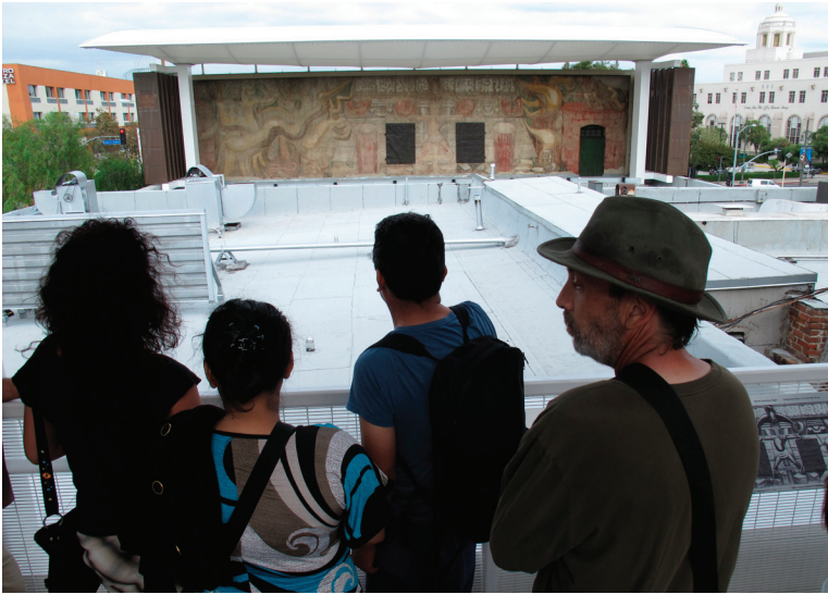
Figure 6 The mural with its protective canopy, seen from the viewing platform at the opening of the site in October 2012. The canopy protects the mural from direct sunlight, rain, and birds and allows an unobstructed view of the mural from a nearby rooftop. Mural: © 2012, Artists Rights Society (ARS), New York/ Sociedad Mexicana de Autores de las Artes Plásticas (SOMAAP), Mexico City
