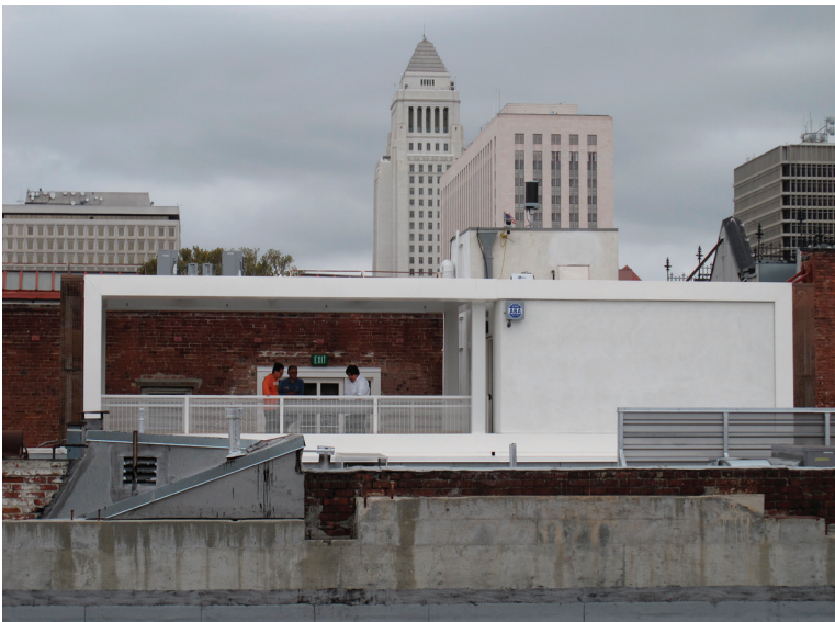
Figure 7 The viewing platform, designed by Brooks + Scarpa Architects, which is accessible from the América Tropical Interpretive Center. Up to twenty visitors can view the mural at one time. A large black-and-white image of the mural positioned on a rail of the platform provides information on the painting's iconography
