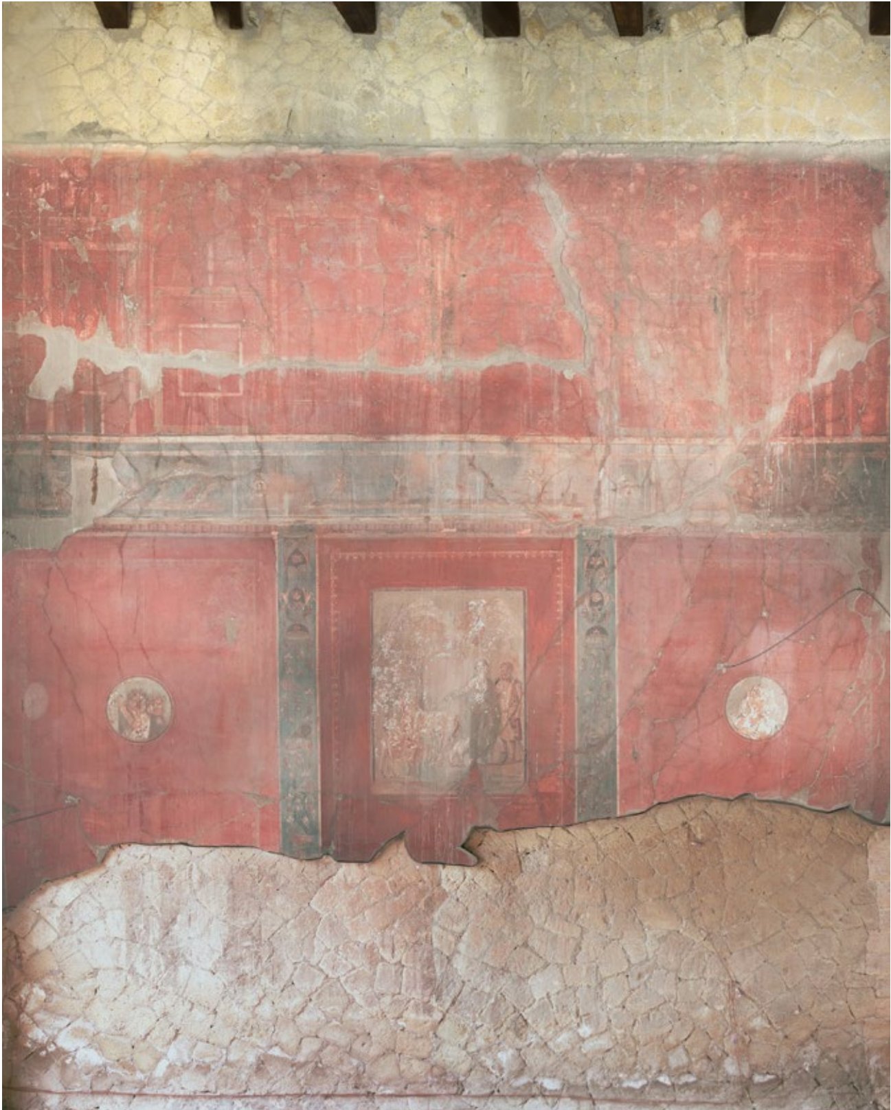
FIGURE 1.10. West wall of the tablinum, 2011. (Photo: Massimo Brizzi)
