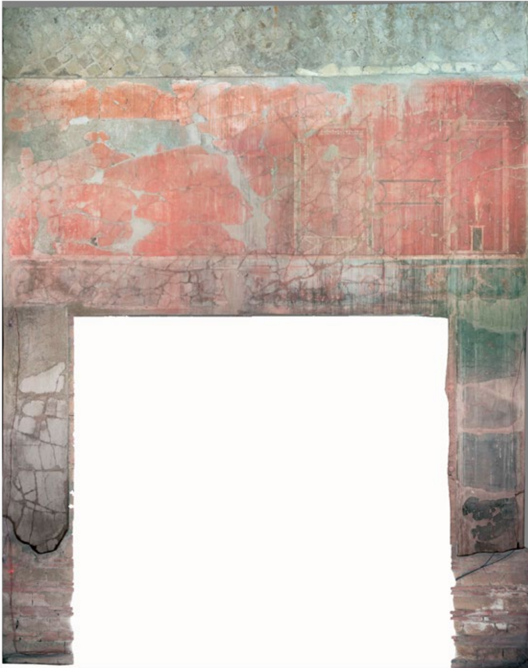
Casa del Bicentenario, Tablinum, South Wall - Overall
