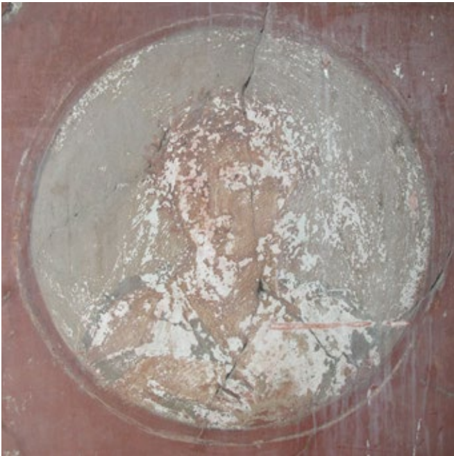
FIGURE 6.29. Medallion at the north end of the west wall, presenting severe deterioration of the figure's robe, neck, and face, with most of the loss down to the exposed underlayer. A deep scrape is seen on the lower right.
