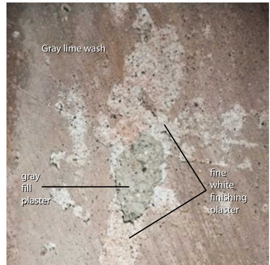
FIGURE 2.26. Flaking paint and plaster expose the stratigraphy of the reconstruction plaster in a loss on the east wall: gray lime wash over a thin white plaster covering a thick layer of gray fill plaster.
