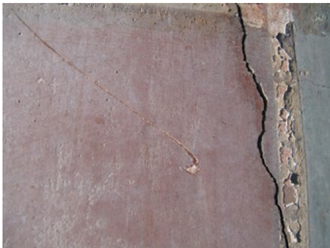
FIGURE 6.9. Open vertical cracks are observed in all four corners of the tablinum.
