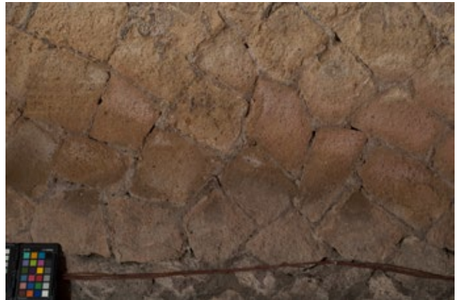
FIGURE 6.51. The same biopatina, visible on the exposed tuff along the base of the west wall. This biopatina is also present along the base of the walls in other parts of the house.
