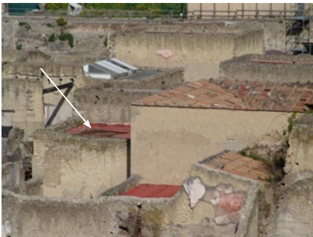
FIGURE 3.2 (ABOVE LEFT). View of roof of the tablinum in 2008, showing pooled rainwater (indicated by white arrow) on the surface.
