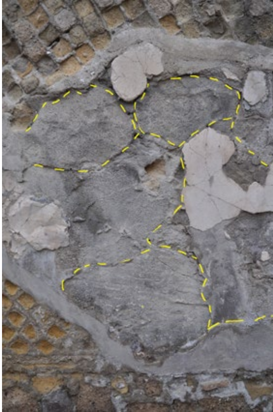
FIGURE 2.13. A remounted section of plaster from another area of the site that has lost almost all the Roman plaster, exposing the backing plaster and leaving an imprint of the original Roman plaster fragment (shown by the yellow dashed line).
