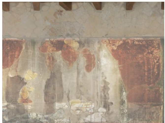
FIGURE 6.8. Damage along the south end of the upper east wall includes powdering and spalling tuff, drips down the wall, and biogrowth, the result of the roof leak and water infiltration.
