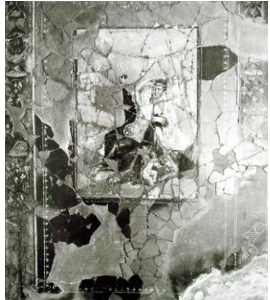
FIGURE 2.28 (RIGHT). Central section, east wall, 1983, showing the sgraffito design in the reconstruction plaster surrounding the central rectangular scene. (Historical Archives of the Soprintendenza Pompei, Maiuri, D29302)
