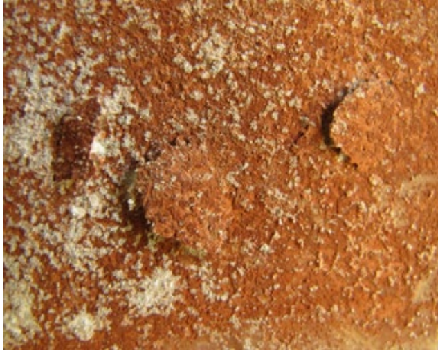
FIGURE 6.55. Detail of damage caused by salt activity in the lower east wall, where the original painted plaster is spalling due to subfluorescence of salts.
