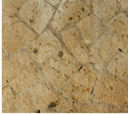
FIGURE 1.26. Example of 1938 construction technique using opus incertum , in which blocks were placed following no regular pattern.
