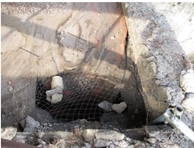
FIGURE 6.7. A large hole in the roof over the tablinum led to water infiltration in the past, particularly in the southeast corner of the room. In 2011, a new slab roof was installed.
