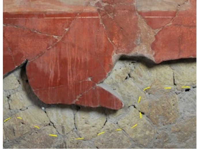
FIGURE 2.31. Lower edge, west wall. The lighter-colored strip (outlined by the yellow dashed line) is the location of the first sloped edging plaster.
