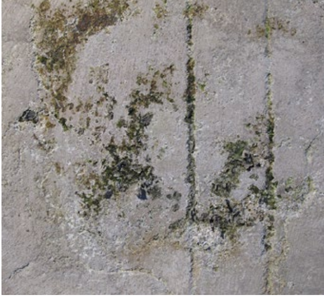
FIGURE 6.48. Detail of the south end of the east wall, showing biogrowth appearing as dark-green marks and black-green deposits.
