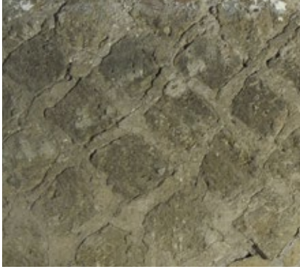
FIGURE 1.25. Original wall construction of tuff blocks in opus reticulatum , an original Roman construction technique in which blocks were placed in a diagonal linear pattern seen along the top of the walls.
