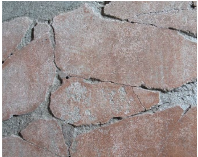
FIGURE 6.12. Detail of the south wall, showing decohesive plaster and powdering paint layers.
