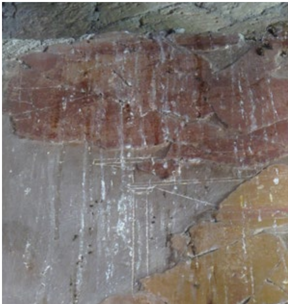
FIGURE 6.46. Drips of bird excrement on the east wall. The upper edges of the wall paintings serve as ideal locations for birds to perch.
