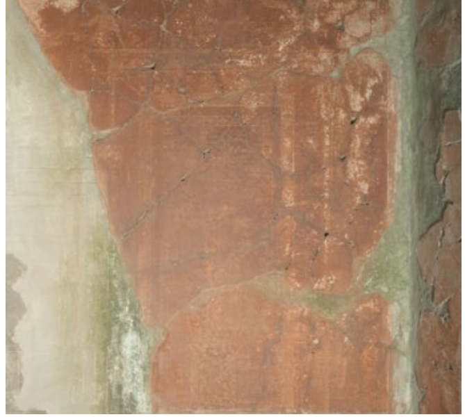
FIGURE 6.49. The southeast corner of the tablinum shows a green microbiological growth that follows drips in areas of previous water infiltration and covers post-1938 fills.
