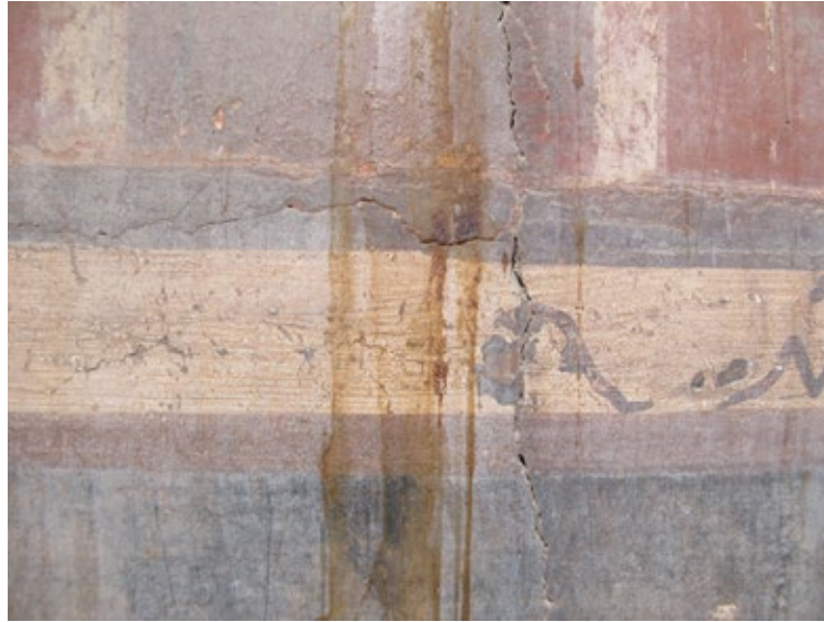
FIGURE 6.45. Detail of the south end of the upper west wall, showing a brown drip that most likely is from a stain used on the beams above.
