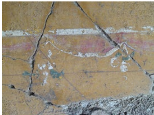
FIGURE 6.23. Decorative borders are composed of different designs executed with thickly applied paint, which exhibits widespread flaking and loss, particularly in specific colors such as green and red.
