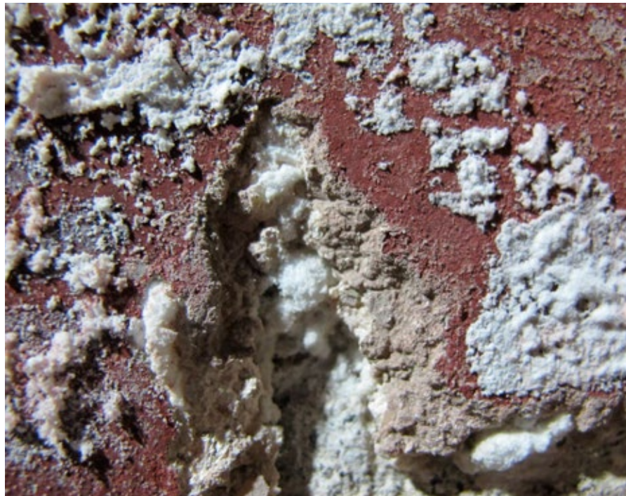
Efflorescence 2013
