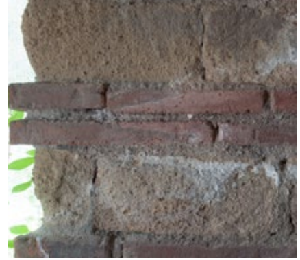
FIGURE 1.27. View at the base of the south wall, showing the original wall construction in opus vittatum , alternating layers of tuff blocks and bricks.
