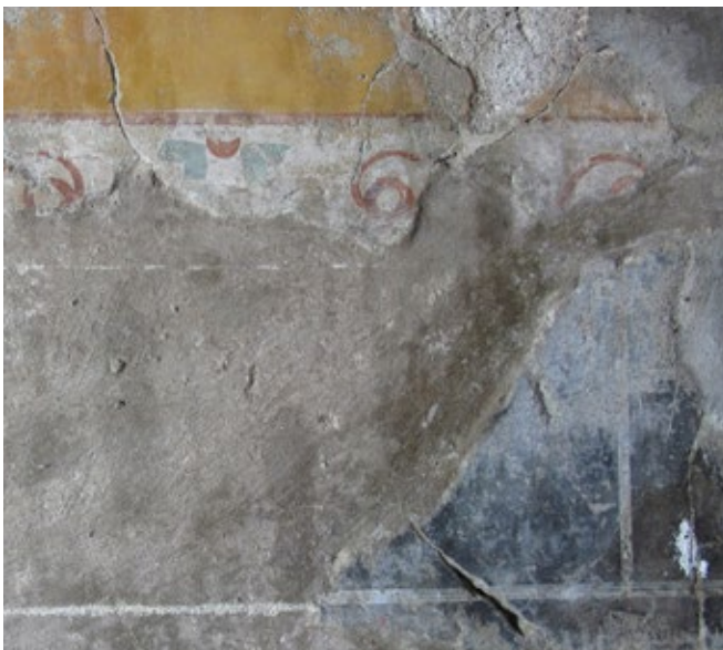
FIGURE 6.37. Remnants of original painted decoration along the base of the wall are extant only in the southeast corner on the east wall with traces of paint on original plaster in some places along the base of this wall.
