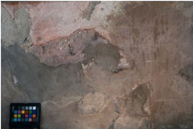
FIGURE 6.50. A pink biopatina along the base of the east wall covers original and reconstruction plaster. This form of bacteria appears to be sensitive to both light and salts, and fluctuates according to environmental conditions.
