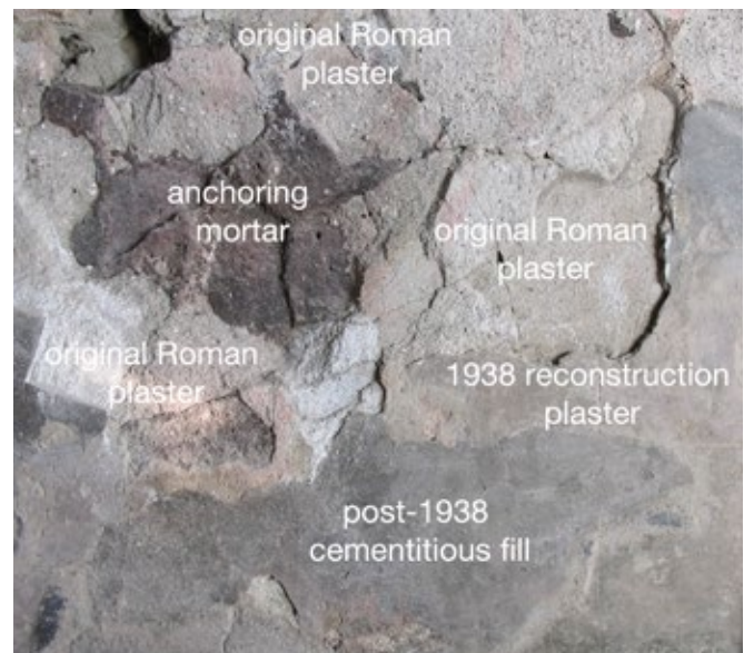
FIGURE 6.38. Detail of base of the east wall, showing plaster stratigraphy with fragments of original plaster remaining under modern fills. Salt efflorescence surrounds the fills.
