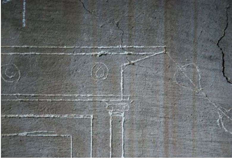
FIGURE 2.25. Reconstruction of the basic design of architectural elements on the upper east wall by Maiuri's team in area of large loss made by incising a line through a gray lime wash applied to the surface to reveal the thinly applied fine white lime plaster below.
