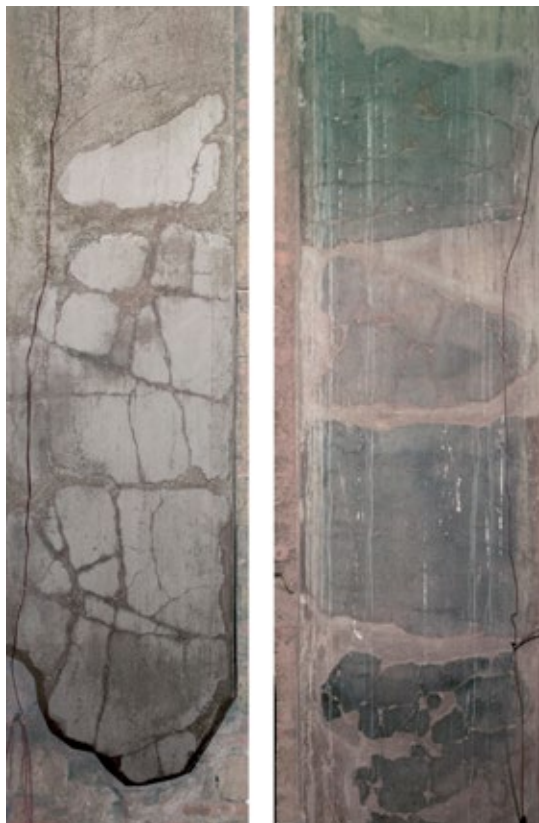
FIGURE 6.18. On the lower section of the south wall, the black paint layer on the east side (left) has been washed away; on the west side (right), the layer is more coherent, although the condition varies across the surface.
