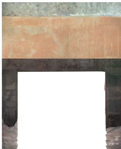
FIGURE 5.19 Basemap of south wall showing presumed location of original background colors.
