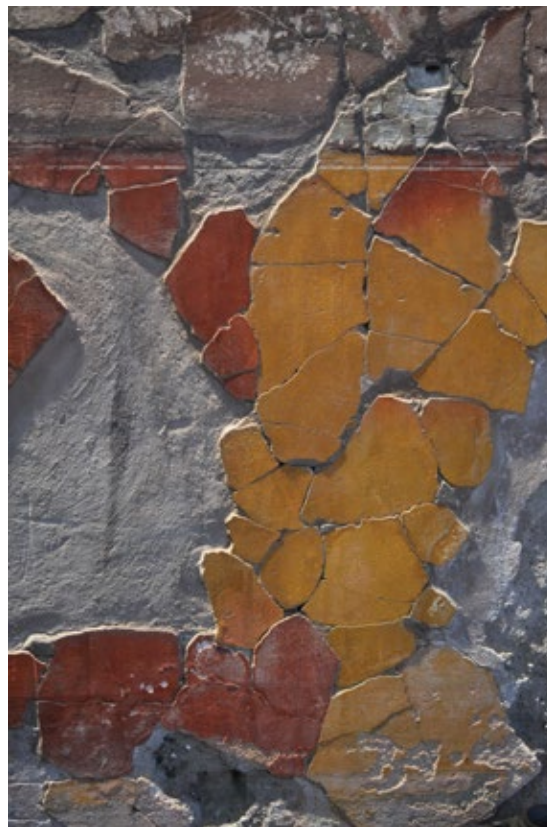
FIGURE 2.8. East wall. Lower register (raking light), showing principally yellow fragments somewhat irregularly fitted together.
