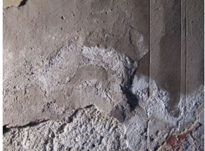
FIGURE 6.56. Subsequent repairs using cementitious plasters have led to salt activity, resulting in further damage to the surrounding original and 1938 reconstruction plasters.
