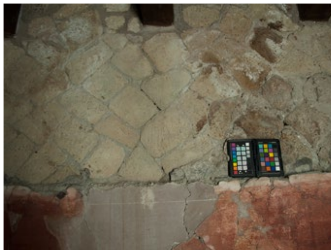
FIGURE 6.10. Tuff blocks on the upper east wall are spalling and powdering in areas of previous water infiltration.
