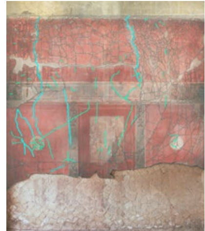
FIGURE 2.11. West wall. The yellow outline indicates an area without significant fractures. The thicker blue lines indicate cracks. The thin lines indicate fragments.
