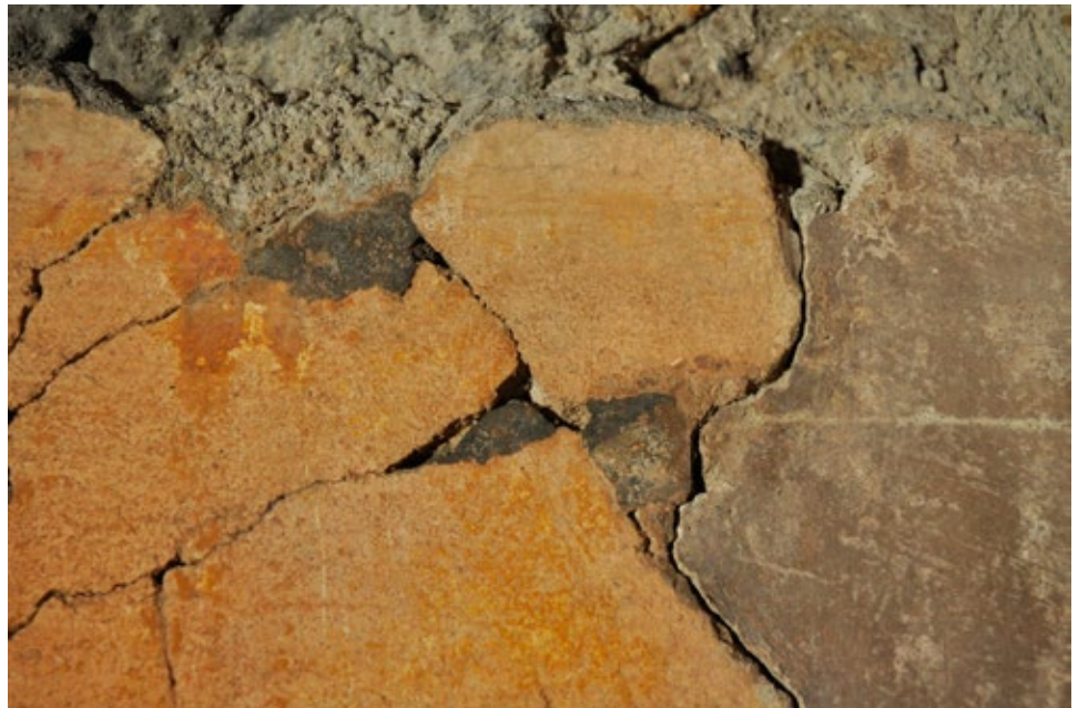
FIGURE 2.13. A remounted section of plaster from another area of the site that has lost almost all the Roman plaster, exposing the backing plaster and leaving an imprint of the original Roman plaster fragment (shown by the yellow dashed line).
