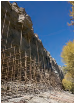
Cliff stabilization included consolidation and rock bolting with cable (Mogao).
