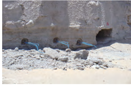
Cliff stabilization included consolidation and rock bolting with cable (Mogao).
