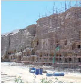
Cliff stabilization included consolidation and rock bolting with cable (Mogao).
