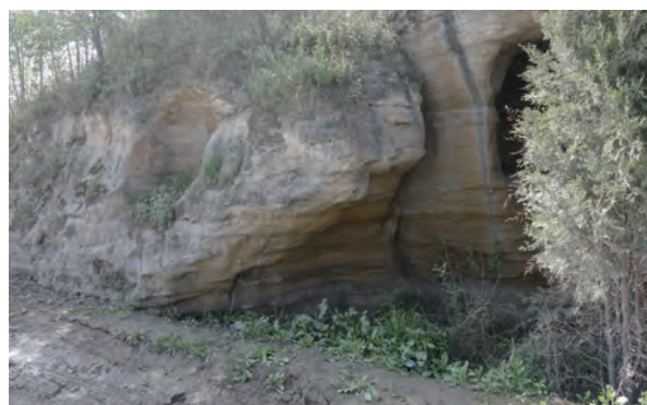
Grottoes located in humid areas require regular maintenance to prevent deterioration caused by soil accumulation and vegetation growth.
