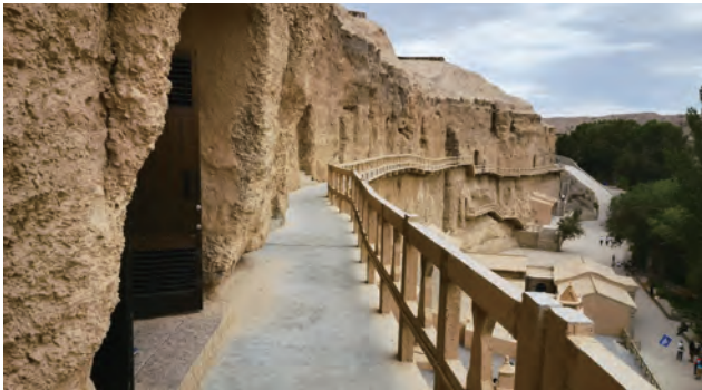
Cliff stabilization, walkways, and cave doors contribute to stabilizing the cliff face (Yulin).
