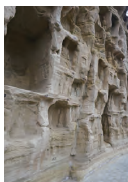
Rock erosion and instability of cliff face (Beishikusi; Wugemiao).
