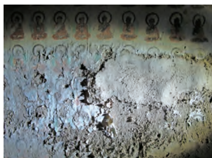
On-going deterioration from natural soluble salts (Mogao, now repaired).
