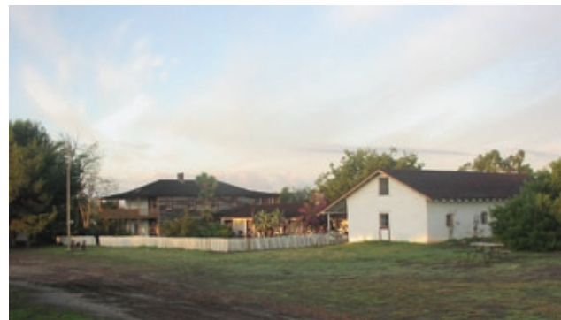
FIGURE 6 The Las Flores Adobe after completion of structural and seismic stabilization of the buildings. By the close of the 2004 construction season, porches on the Monterey block were reinstated, building envelopes were secured against weather, and interior rehabilitation was started.
