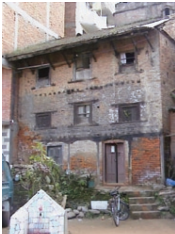
FIGURE 6 Original dalan structure walled in at a later time. Note that there is no external masonry pier adjacent to the external dalan column.
