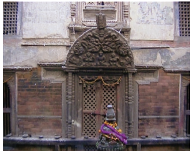
FIGURE 4 Structure with timber bands at mid-height of the wall.
