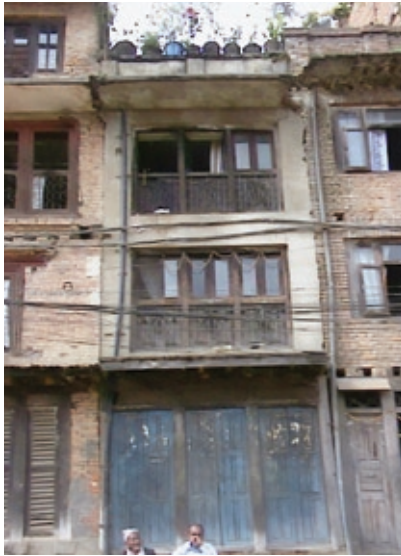
FIGURE 12 Full-width windows that do not leave sufficient width for the lateral pier.
