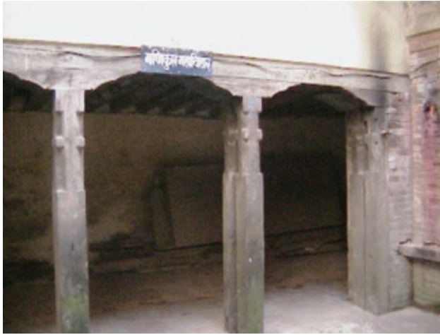
FIGURE 5 Dalan structure at the ground floor of a courtyard.
