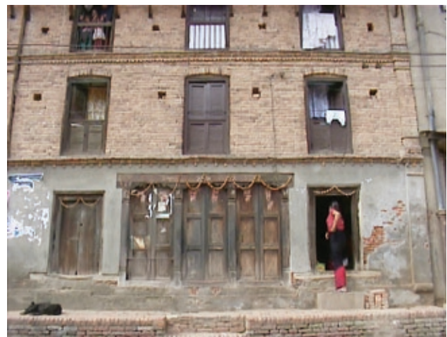
FIGURE 11 Full-height windows with flat brickwork arches.
