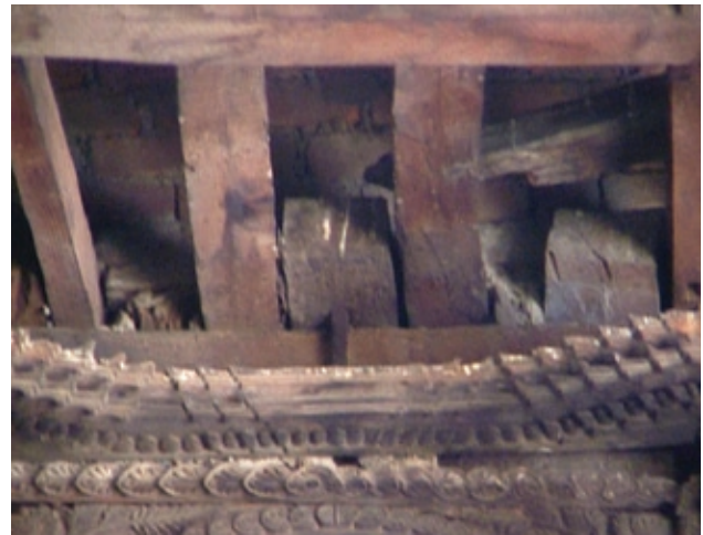
FIGURE 1 Timber pegs, or chokus .
