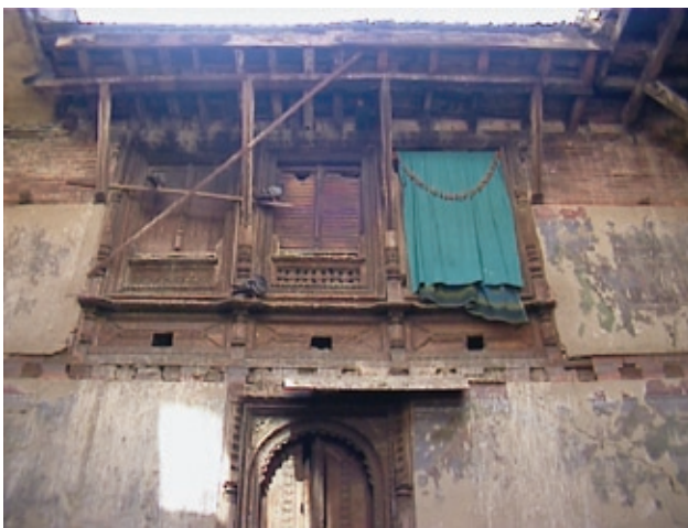
FIGURE 10 Full-height windows based on the San Jhya model.
