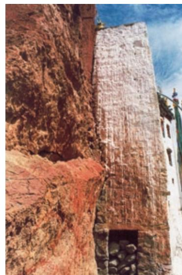
FIGURE 4 Vertical structural crack between buildings and the adjacent hill. This significant detachment was caused by the earthquake.
