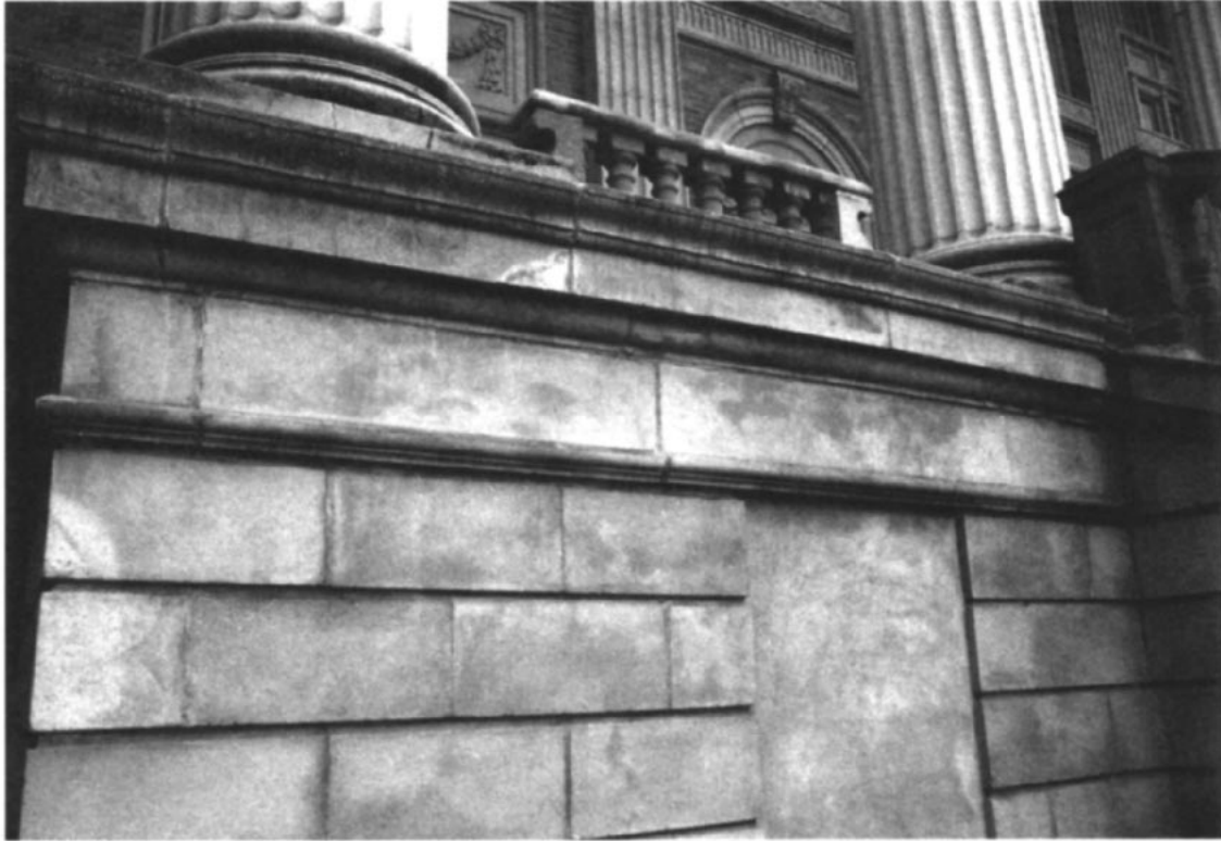
Figure 6. Exterior of Crescent Hill Baptist Church, Louisville, Kentucky, treated with epoxy resin in 1983. Figure shows the tones of the treated surface in 1989.
