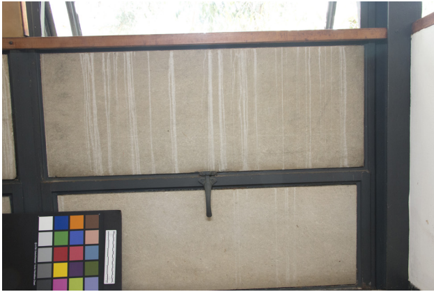
FIGURE 3.5 Photo showing white streaks on panel HE-3-5. Photo: Laura Matarese and Chandler McCoy, 2015. ©J. Paul Getty Trust.
