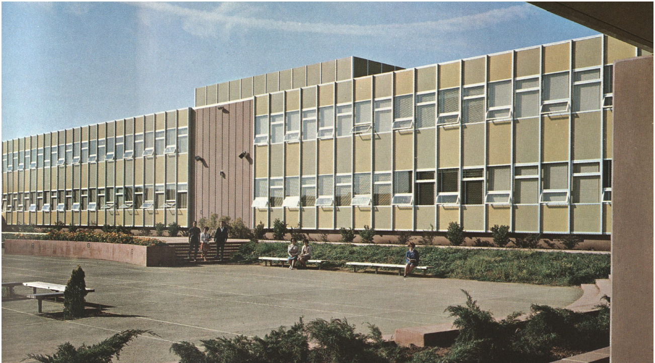
FIGURE A.5 Photo showing the use of Glasweld insulated sandwich panels with a mineral-enamel coating in curtain-wall construction (Sweet's Catalog 1965, 3b/Uni). Reproduced courtesy of Dodge Construction Network and The Ohio State University Libraries.
