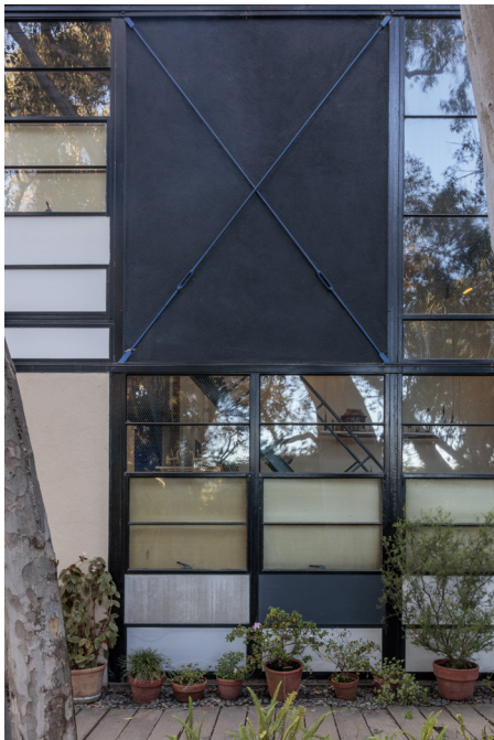
FIGURE 2.1 Photo of Eames House studio exterior showing various types of glass, stucco, and Cemesto and replacement panels (painted and unpainted). Photo: Joshua White, 2016. ©Eames Office.
