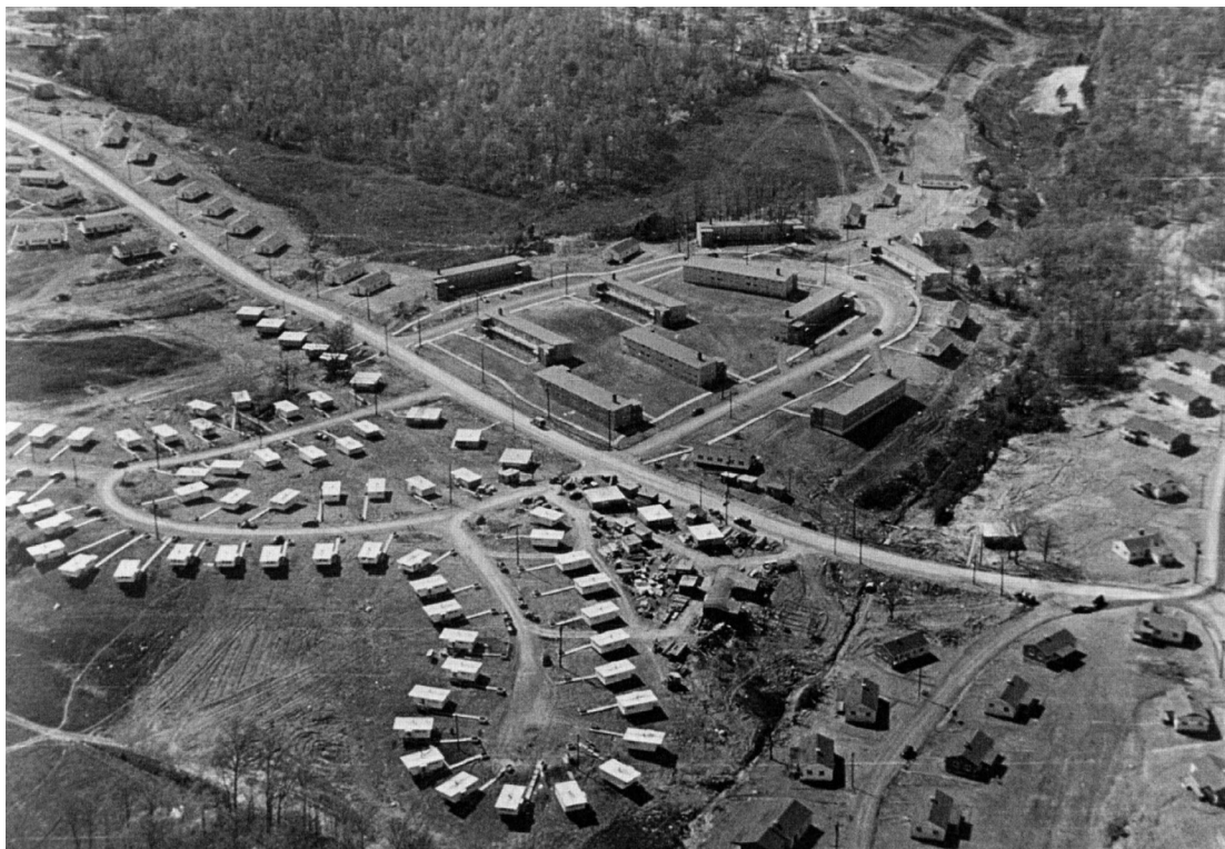
FIGURE 1.7 Aerial photograph of Hillside Road in the defense housing community at Oak Ridge, Tennessee, showing Cemesto houses and site layout (Hales 1997). Photo: James E. Westcott, US Army Corps of Engineers, Manhattan Engineer District, Oak Ridge, Tennessee.
