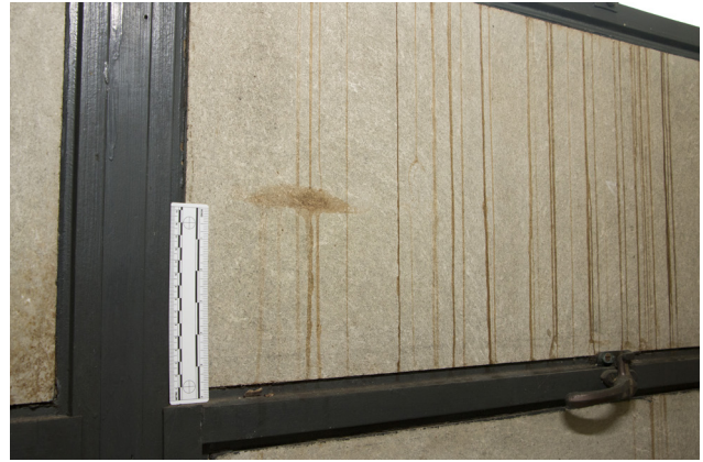
FIGURE 3.6 Photo showing brown marks on panel SW-1-5. Photo: Laura Matarese and Chandler McCoy, 2015. ©J. Paul Getty Trust.
