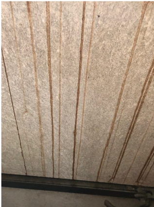
Image 3. Brown drip-like stripes from indoor Cemesto, top office. Sample 8.
