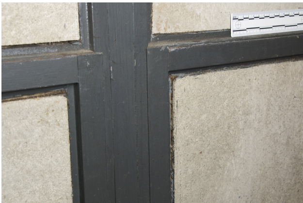
FIGURE 3.9 Panels on the studio interior, west elevation, shown protruding from the frame, exposing the Celotex fiberboard core. Photo: Laura Matarese and Chandler McCoy, 2015. ©J. Paul Getty Trust.
