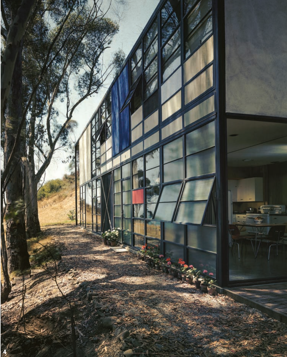
Figure 4 The Eames House in 1950, shortly after construction was completed. Set behind the historic row of eucalyptus trees, the building is a steel-frame structure with unusual exterior cladding made up of steel industrial windows and a variety of infill materials and colors.
