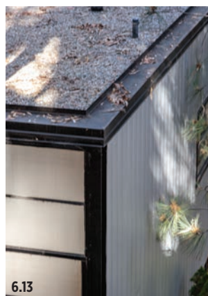
Figure 6.13 Southeast corner of the studio roof, in 2017, showing the curb added as part of the reroofing campaign in 2014 to improve weather tightness and drainage. Also visible at the top of the wall are the original and later (second) edge flashings.
