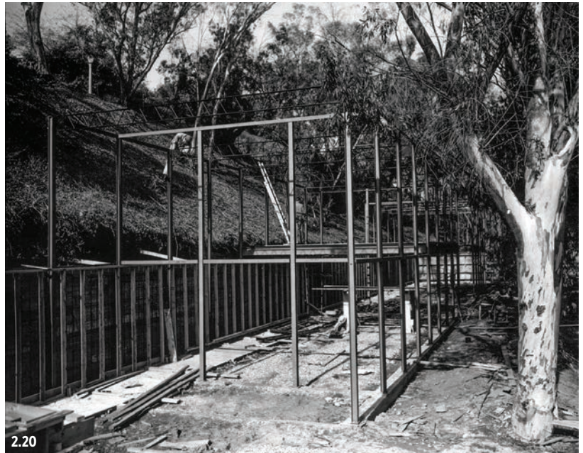
Figure 2.20 Photo showing the structural steel frame and retaining wall before installation of the roof decking and window units, ca. December 1948.
