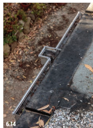
Figure 6.13 Southeast corner of the studio roof, in 2017, showing the curb added as part of the reroofing campaign in 2014 to improve weather tightness and drainage. Also visible at the top of the wall are the original and later (second) edge flashings.
