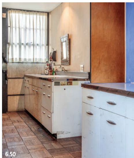
Figure 6.50 Original prefabricated painted steel cabinets in the studio kitchenette, 2017. The cabinets show rusting of the steelwork caused by the breakdown of painted surfaces and exposure to damp. An ongoing rust removal and surface protection program will be developed.
