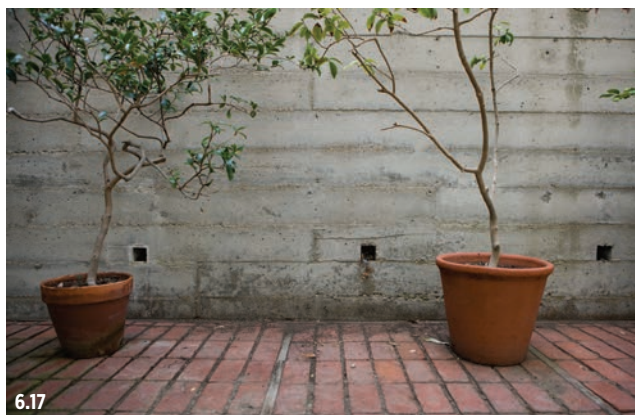
Figure 6.17 East face of the original concrete retaining wall facing the central court, in 2016, showing three weep holes from the original French drain, which runs behind the wall near the base.
