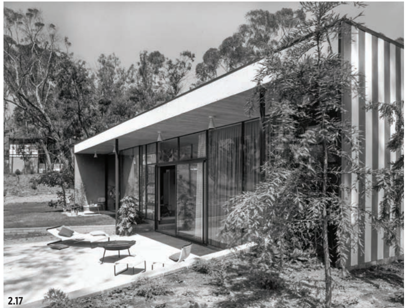
Figure 2.17 View of the living room facade of the Entenza House, which looks out toward the ocean, 1950. The house used many of the same construction and finishing materials as the Eames House, to different effect. Note the Ferrobord wall on the far right, painted in alternating stripes of gray and white. The Eames studio is visible at left, in the distance.
