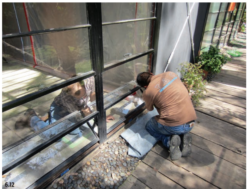
Figure 6.12 A worker repairing a Truscon hopper window in 2012. Repair of steel components should be carried out as part of a regular, cyclical maintenance schedule.
