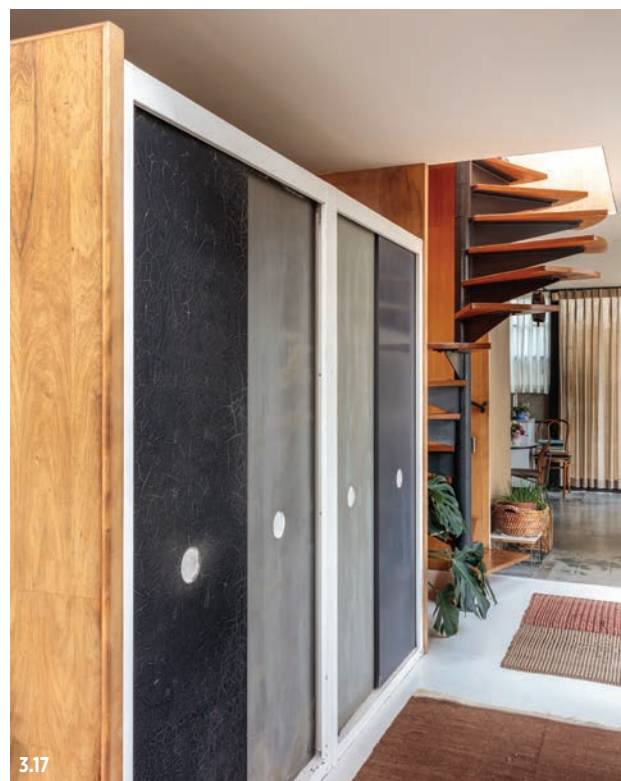
Figure 3.17 Freestanding closets that serve as the hallway's west wall, 2017. The closets are constructed of painted wood with prefabricated steel sliding-door assemblies. The end wall of the closet unit is paneled with rosewood.
