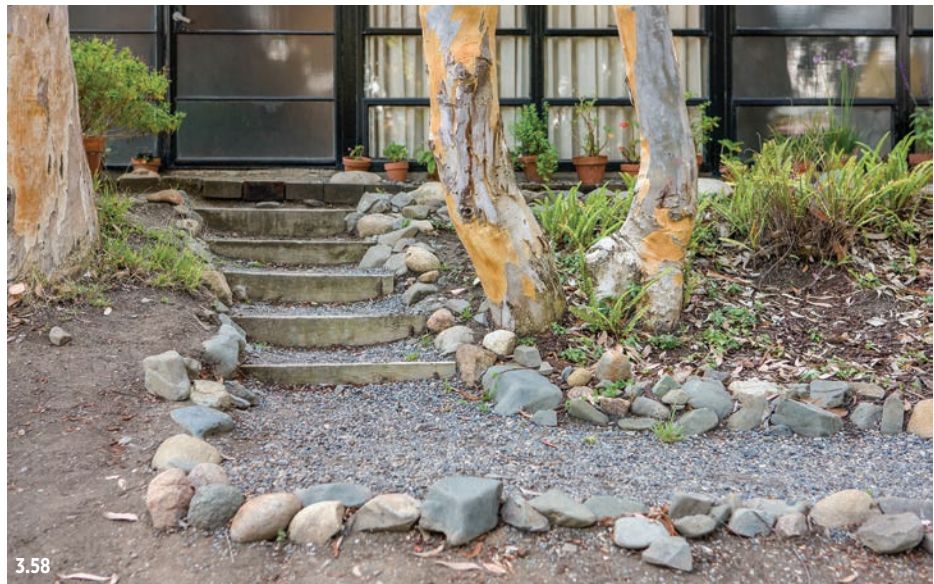
Figure 3.58 Lower pathway and steps leading to the front door, 2016. The pathway is lined in rubble stone and covered in river rock, and leads across the meadow to the front of the residence.
