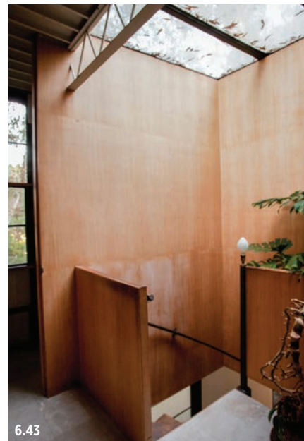
Figure 6.43 Upper-level area of the spiral staircase, 2011. The plywood veneer walls have suffered light and moisture damage and require conservation.
