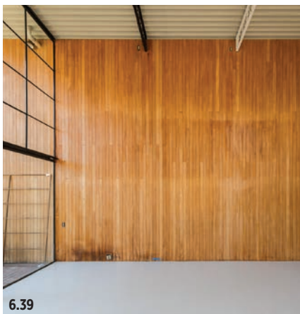
Figure 6.39 The tallowwood wall in the living room, cleaned and refinished in 2012, with the patina of use and age carefully retained.
