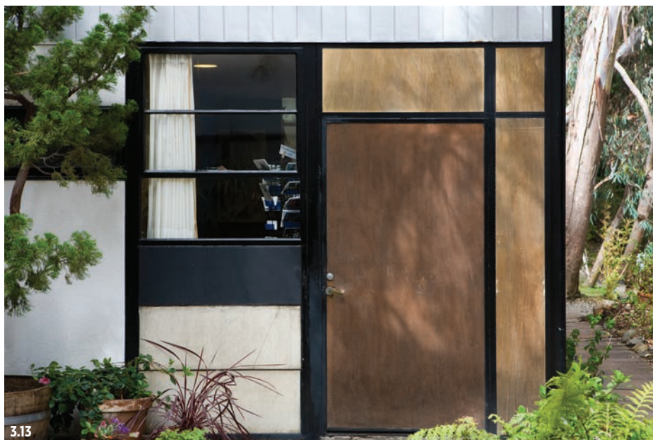
Figure 3.13 South entrance to the studio, 2017. The wood veneer door has smaller plywood panels above and directly to the right. To the left, a panel of Truscon sash is infilled with a combination of clear glass and opaque panels.
