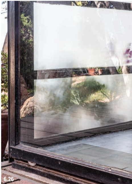
Figure 6.26 Base plates and sliding door of the kitchen after repair in 2012, maintaining the integrity of the steelwork and restoring the watertightness of the facade. Photographed in 2017.
