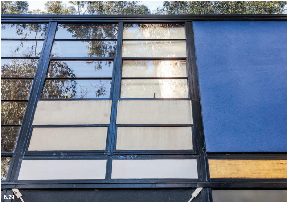
Figure 6.29 East elevation of the residence, in 2017, infilled with a variety of cladding materials, including solid stucco panels and sections of Truscon steel-framed sash filled with clear glass and Cemesto panels. At lower right is the gold-leaf panel above the front door.
