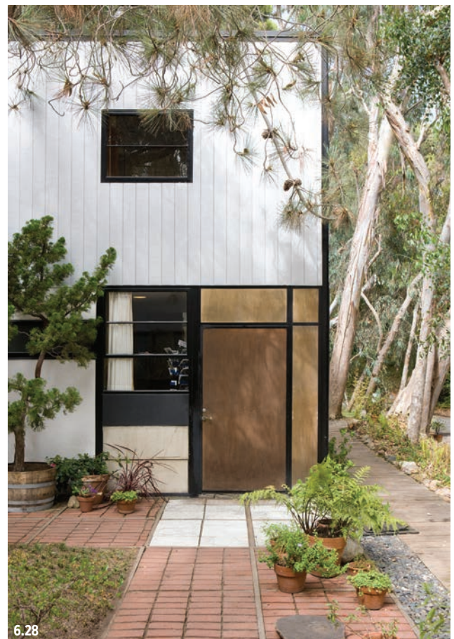
Figure 6.27 View from the kitchen toward the meadow, 2017. The Truscon steel sash contains operable hopper and awning windows and fixed windows, glazed with either obscure or clear glass. At left is the sliding door.
