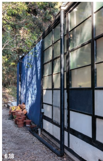
Figure 6.18 West elevation of the studio in 2017, showing new gutter and rain leaders connected to horizontal storm-water lines that keep all roof water away from buildings. These improvements were installed as part of the 2014 reroofing.
