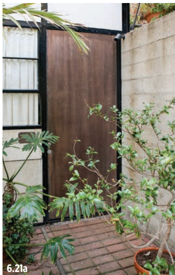
Figure 6.21a Entry door to the utility room from the central court, 2016. Mold growth and evidence of damp are observed on the adjacent retaining wall.
