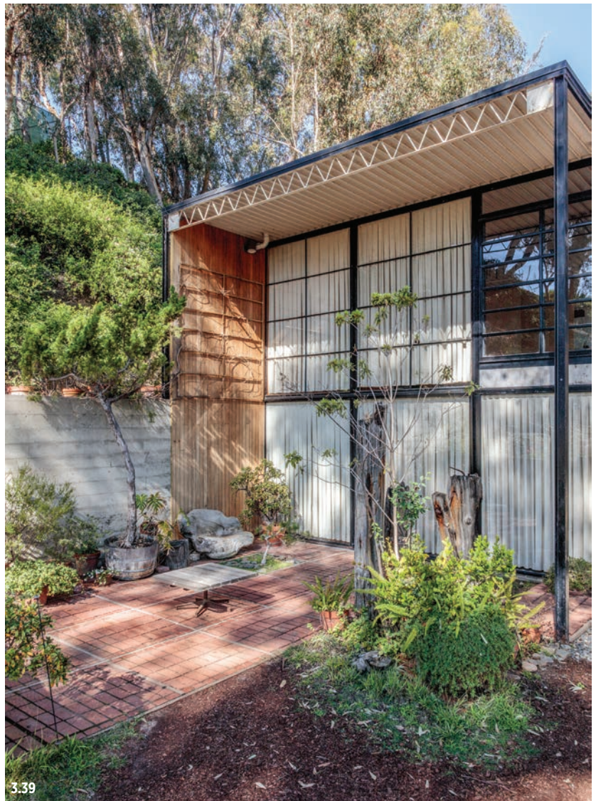
Figure 3.39 View of the south court off the living room, 2017. The fully glazed south wall and wide sliding door integrate indoors and outdoors. The roof overhang, one structural bay's width, along with the extension of the living room's tallowwood paneling to the exterior, heightens the sense that this is an outdoor room.
