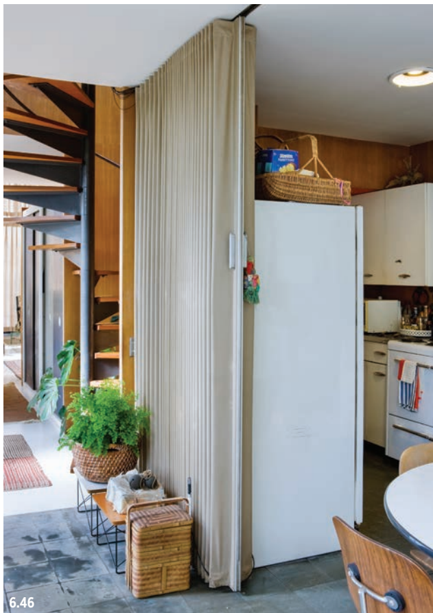
Figure 6.46 The original Modernfold door separating the kitchen and dining area/hallway, maximizing flexibility of the space, 2016. In practice, the Eameses kept the door folded, where it served as a wall to cover the back of the refrigerator as shown here.
