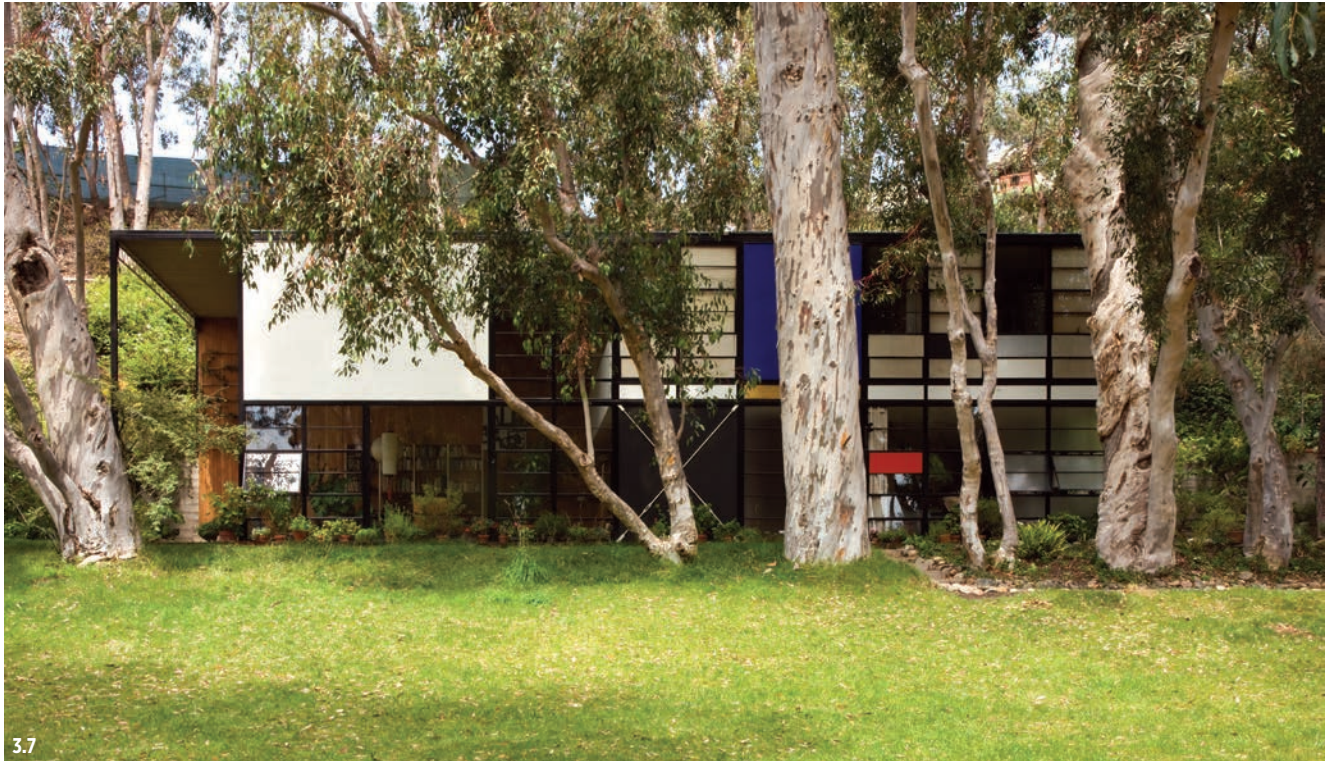
Figure 3.7 View of the east elevation of the residence, 2013. The strict geometric order conferred by the building's steel frame is enlivened by the various configurations of architectural sash infilled with glass or solid panels in a variety of textures, materials, and colors.
