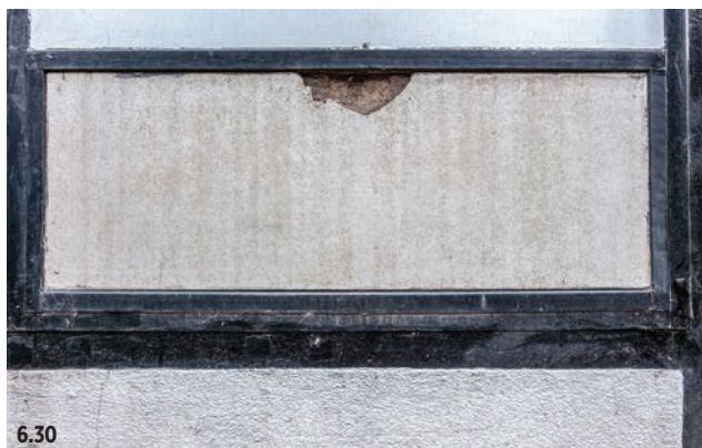
Figure 6.30 Cemesto panel, studio west facade, 2017. Damaged and deteriorating original Cemesto panels, which contain asbestos, present potential safety hazards.
