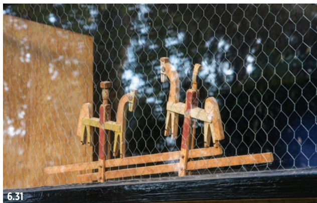
Figure 6.31 Wire glass in a window of the studio, 2016. Some original building materials, such as wire glass and Cemesto panels, are difficult to source or are no longer available.
