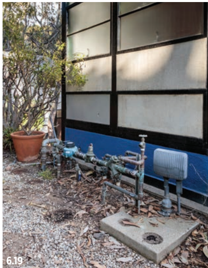
Figure 6.19 Spigots and pipes on the west elevation of the residence, 2017. The faucets, sprinklers, irrigation system, and watering regime for the upper path and slope are potential water hazards behind the retaining wall and require careful monitoring.
