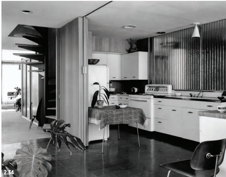
Figure 2.34 View of the kitchen, 1949. The Modernfold accordion door could be used to close off the kitchen, though in practice the Eameses kept it open. The corrugated glass wall above the kitchen cabinets obscures views of the service area while allowing light into the space.
