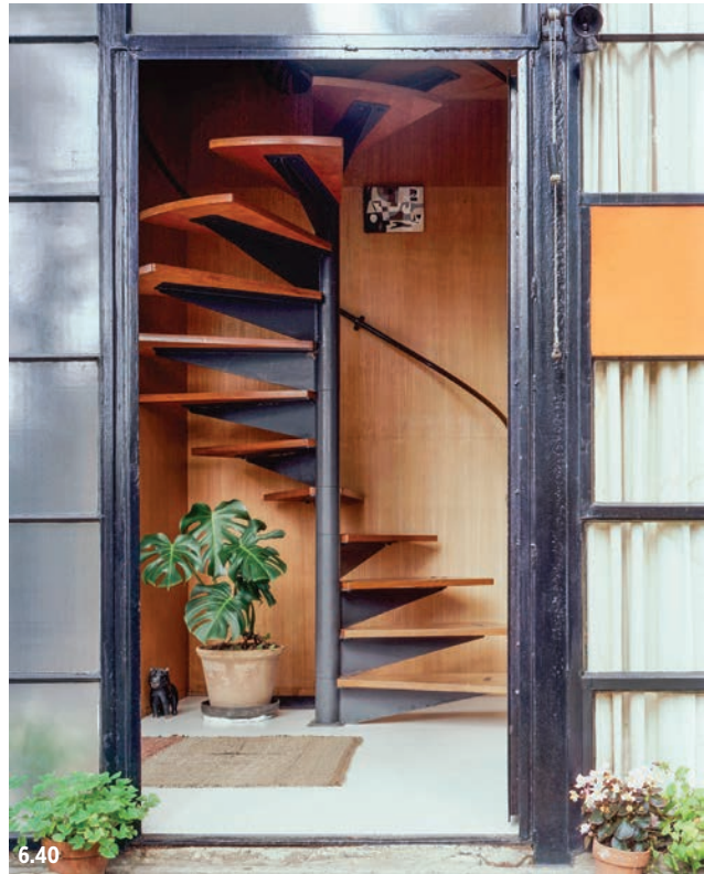
Figure 6.40 The residence's spiral staircase, as seen through the open front door, 2014. Plywood treads are mounted on custom-made steel flanges that radiate from the central steel column.
