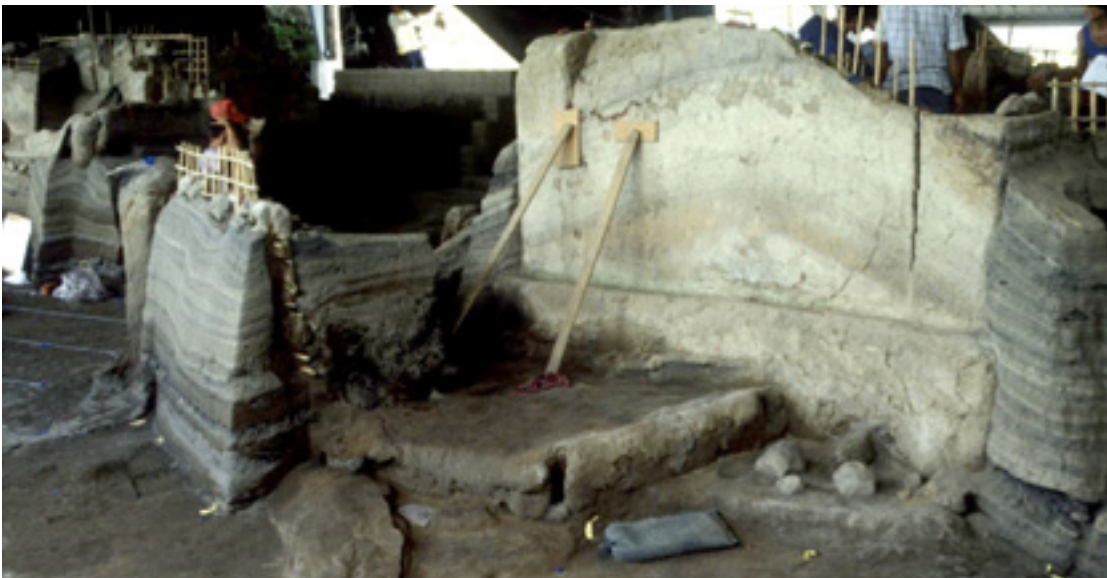
Conserving and managing a site entails integrating all needed actions to maintain and protect structures, for example the temporary shoring at structure 10. © J. Paul Getty Trust. Photo: Carolina Castellanos
