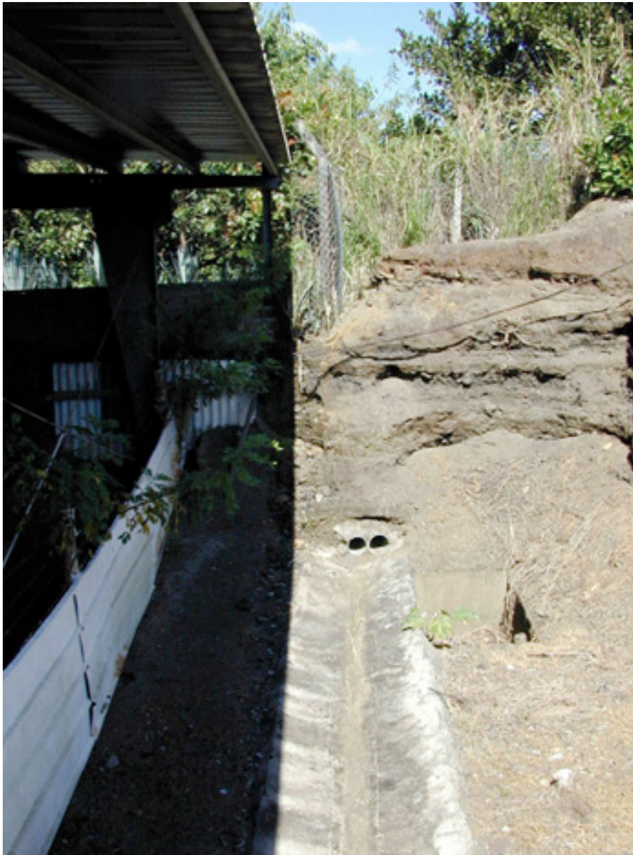
Conserving and managing a site requires prioritizing, for example having adequate drainages around the protective shelters. © J. Paul Getty Trust. Photo: Rand Eppich
