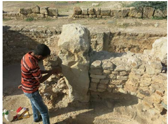
FIGURE 17 Mortar repair stabilization of wall faces and tops (Ermanno Carbonara)
