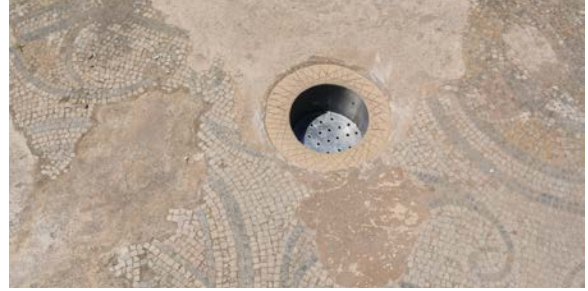
FIGURE 13 Drainage pit within a room with a mosaic, Maison de la Chasse (Ermanno Carbonara)
