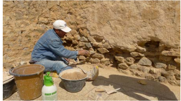
FIGURE 16 Mortar repair stabilization of wall faces (Livia Alberti)
