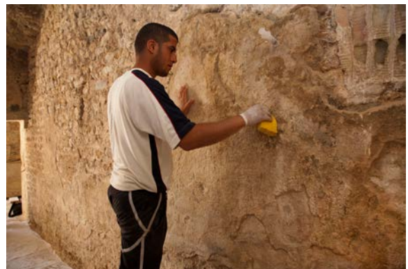
FIGURE 18 Mortar repair and injection grouting stabilization of wall plasters (Scott Warren)
