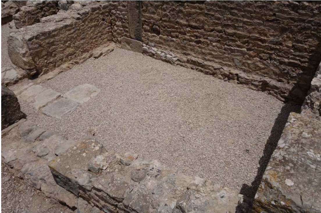
FIGURE 14 Reburial of lost part of pavement with a sand layer, non-woven geotextile separation membrane, and gravel layer covering, Maison de la Chasse (Ermanno Carbonara)
