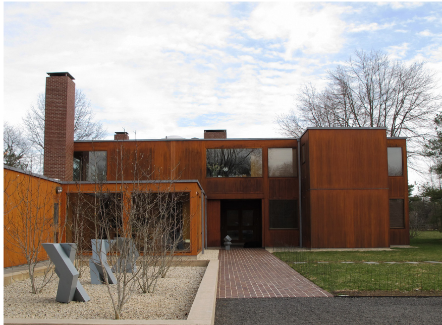
FIGURE 3. Steven and Toby Korman House, 1971–73, Whitemarsh Township, Pennsylvania. View of the north- west entrance elevation with its cypress wood detailing prior to con- servation, photographed 2014.
