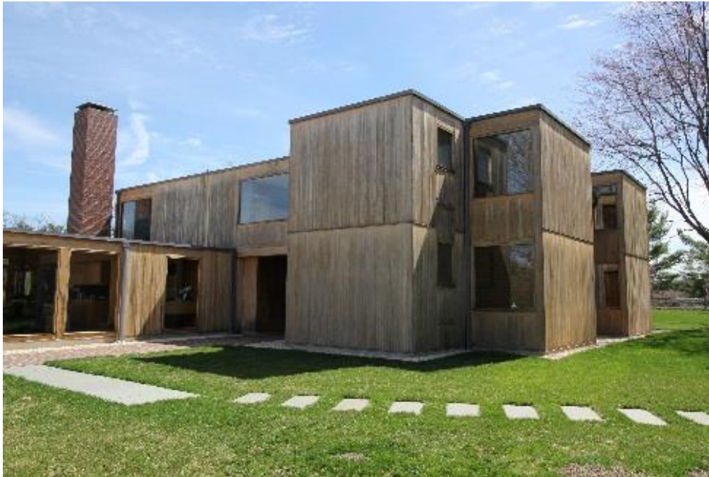
FIGURE CS-C.11 View of cypress siding during natural weathering process April 2015. Photo: Andrew Fearon
