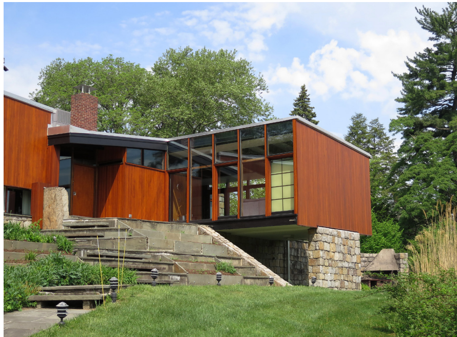
FIGURE 5. Samuel and Ruth Genel House, 1949–51, Wynnewood, Pennsylvania. View from the entrance elevation with vertical wood siding and rubble masonry, from the southeast, photo- graphed 2015.
