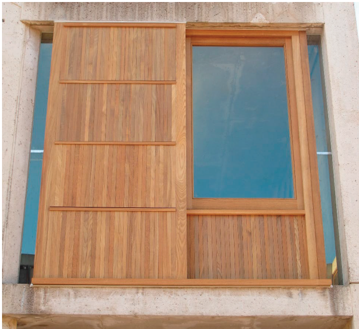
FIGURE CS-B.12 View of Mock-Up 3, after installation of new wall assembly, March 31, 2015. New teak (First European Quality grading) has been used for the sills, horizontal drips, vertical trims, and jambs, as well as the T&G boards (lower left two panels), and reclaimed teak has been used (top two panels at left and lower right panel below window). Photo: J. Paul Getty Trust
