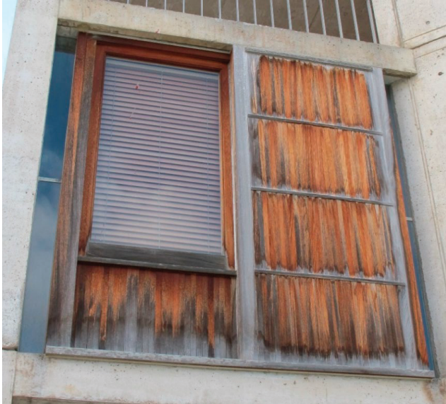
FIGURE CS-B.9 View Mock-Up 2 prior to treatment, September 18, 2014. This mock-up was originally intended to explore the feasibility of removing the exterior teak cladding for cleaning and repair in a shop, installation of performance-based improvements, and reinstallation of teak after completion. Based upon what was learned of the teak assembly and fastening details in Mock-Up 3, the team determined it was not feasible to remove the teak cladding without significant damage to it. Given that minimal to no moisture damage was observed in the internal framing this location, limited improvements were carried out with the teak in situ. Photo: J. Paul Getty Trust
