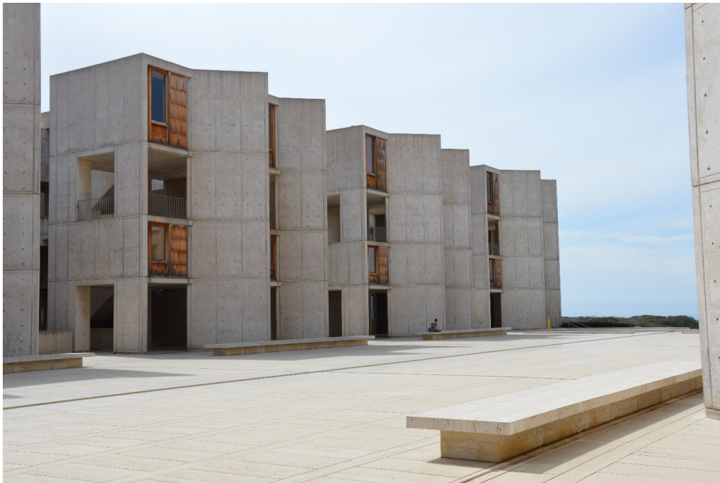
FIGURE CS-B.1 Salk Institute for Biological Studies, view of the teak window wall assemblies in the south study towers from the main plaza, 2014. Photo: J. Paul Getty Trust
