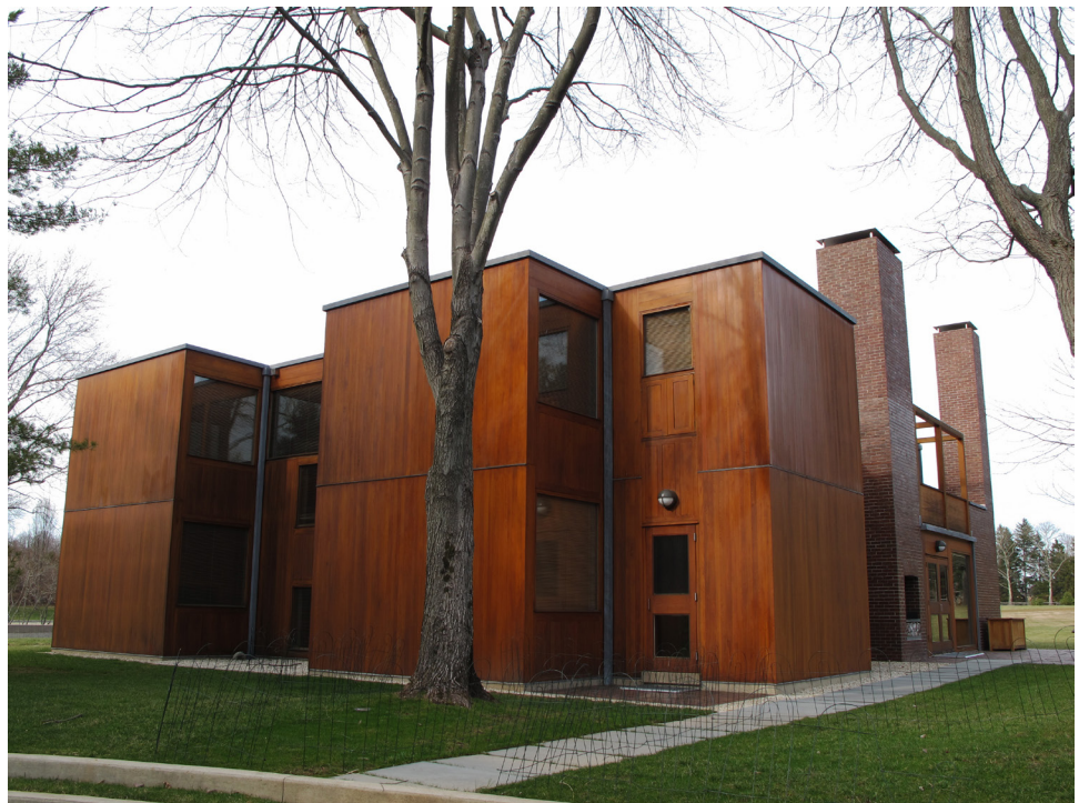
FIGURE 18. View of the Korman House, 2014. Later surface treatments applied to the cypress wood siding gave it a dark red-orange color.
