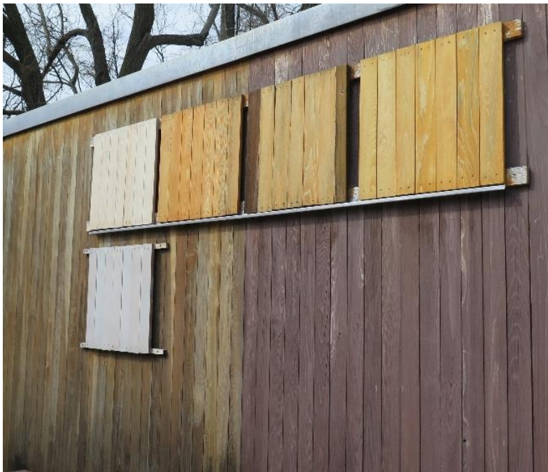
FIGURE CS-C.4 Test Panel of various finishes on sample boards at the site, February 2015. Photo: J. Paul Getty Trust
