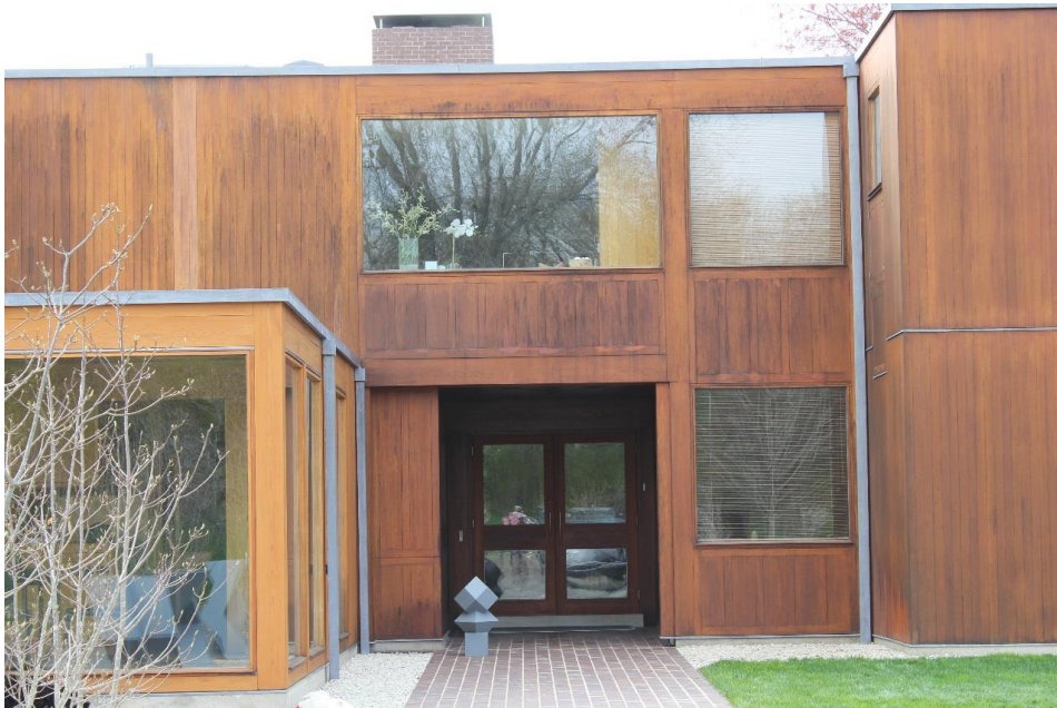
FIGURE CS-C.8 Photograph showing past surface treatment of the exterior wood siding, with a dark orange color, April 2014. Photo: Andrew Fearon
