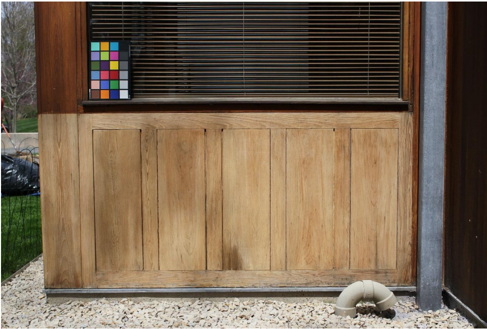
FIGURE CS-C.9 Finish removal Mock-up of the exterior wood siding, with a dark orange color upper left, May 2014. Photo: Andrew Fearon
