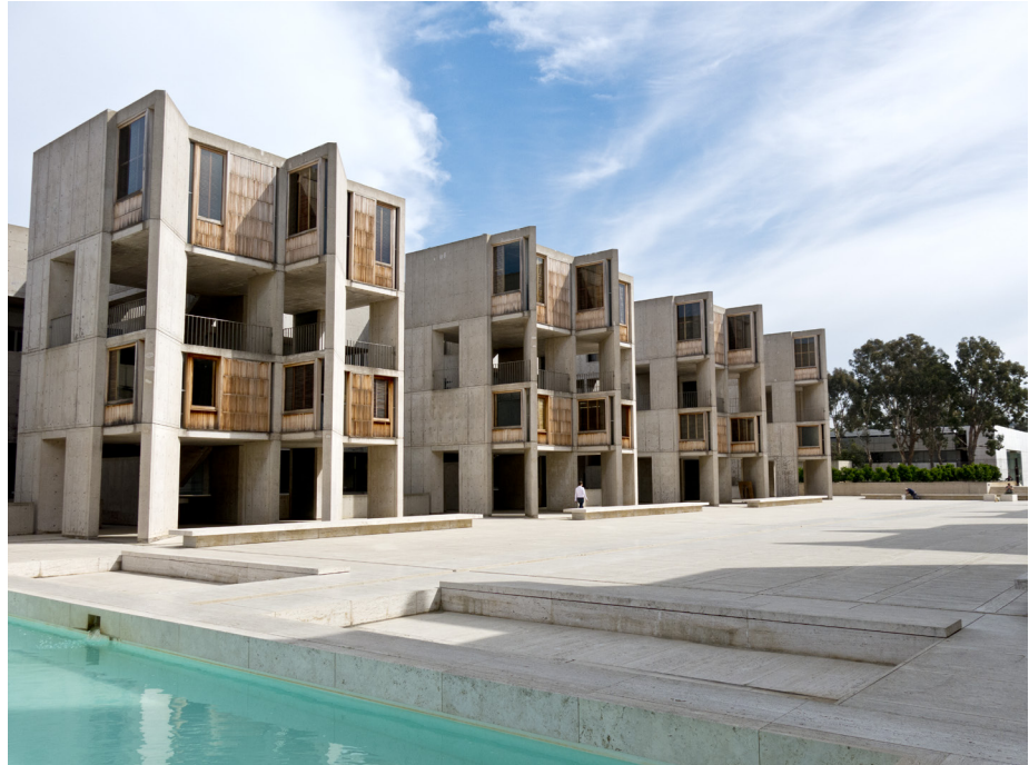
FIGURE 1. Salk Institute for Biological Studies, 1962–65, La Jolla, California. View of the main plaza prior to conserva- tion of the teak window wall assem- blies, photographed 2014.
