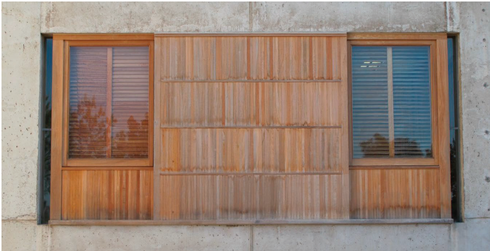
FIGURE CS-B.7 View of Mock-Up 1.A, at completion of treatment, March 30, 2015. Various cleaning trials were carried out, utilizing sodium percarbonate and detergent solutions, as well as D/2 Biological Solution. The effectiveness of sanding was also testing for the removal of the fungal biofilm and improving the overall appearance of the wood and its ability to take a penetrating surface treatment. Several "colorless" treatments were applied across the base of the wall including water repellent preservatives and borate-based treatments with sealers. Photo: J. Paul Getty Trust
