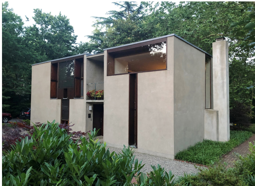
FIGURE 6. Margaret Esherick House, 1959– 62, Chestnut Hill, Philadelphia. View of the entrance elevation from the northwest, photographed 2015. Apitong wood is used at the win- dows and entry alcove. Photo: Paul Savidge.
