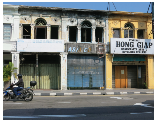
FIGURE 4.1. A row of shophouses with vacant second stories. The depopulation of the central city is evident from these empty second-floor units, where families once resided above the shops below. Photo: Jeff Cody © J. Paul Getty Trust.
