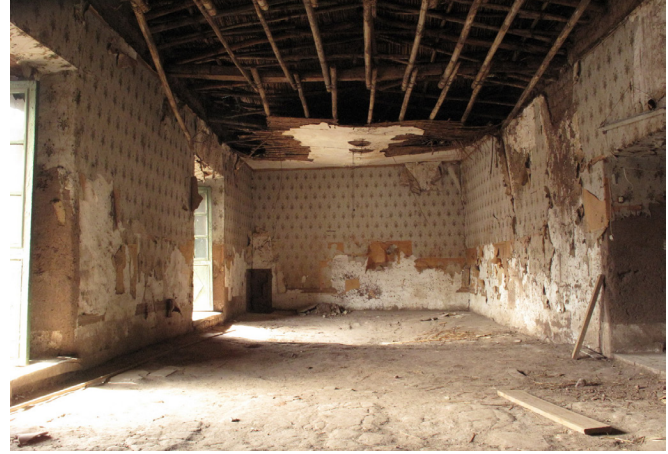
FIGURE 6.16 View of room A-204—a long rectangular second-floor room along Calle Arones—looking south. Image: Claudia Cancino.
