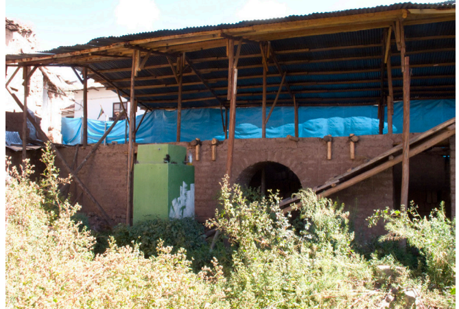
FIGURE 6.6 Collapsing rear wing of house along Calle Nueva Alta (not part of construction assessment), with shoring and temporary roof in place. Image: Amila Ferron.
