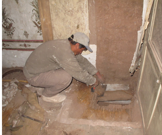
FIGURE 7.2 (FAR RIGHT) Prospection process: project team engineers inspecting the opened floor area at Casa Arones. Image: Sara Lardinois.
