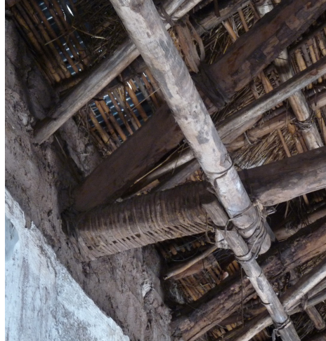
FIGURE 6.34 (LEFT) Prospection IIC-2, photographic view of tie beam end at mud brick wall (at left), with ceiling joist below. Image: Mirna Soto, for the GCI.
