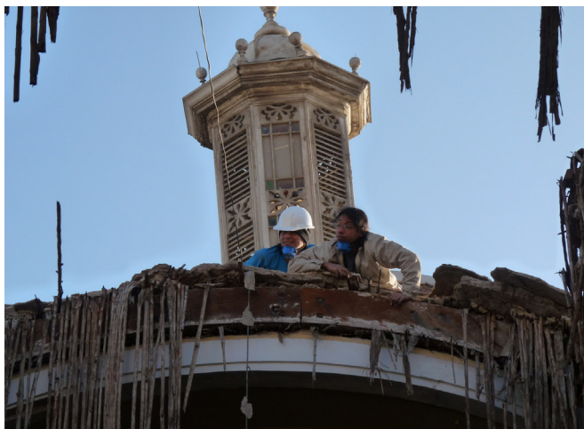
FIGURE 7.3 Prospection process: project team documenting the roof connections at the Cathedral of Ica, taking advantage of those areas made visible by the previous collapse of portions of the roof. Image: Mirna Soto, for the GCI.
