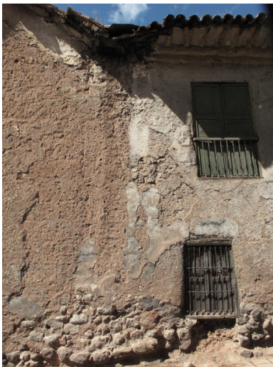
FIGURE 6.40 Erosion and loss of base course stones outside room C-109, north façade. Image: Claudia Cancino.
