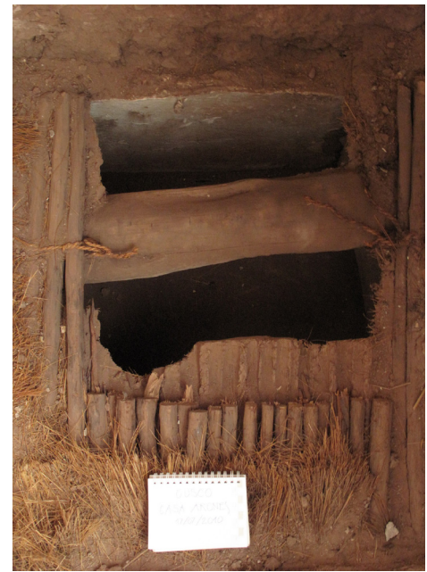
FIGURE 6.30 Prospection IIW-1, photographic view of floor construction at the northeast corner of room A-203. Image: Claudia Cancino.
