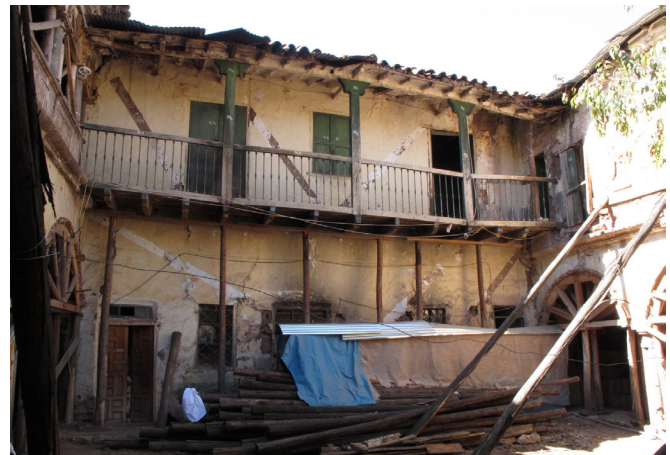
FIGURE 6.14 View of cantilevered wood balcony at east side of patio. Image: Sara Lardinois.
