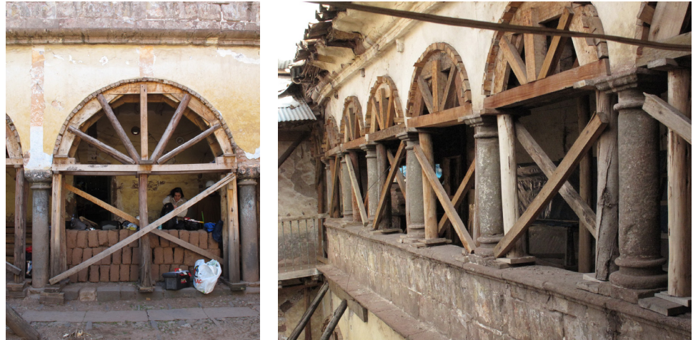
FIGURE 6.24 (LEFT) First floor arcade at the north side of the patio, with stone columns and fired brick arches (covered with plaster). Image: Sara Lardinois.
