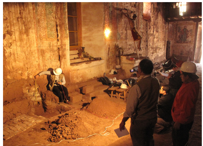
FIGURE 7.4 Prospection process: supervising architect narrating a video documenting what was discovered through a foundation prospection at the Church of Kufio Tambo. Image: Claudia Cancino.
