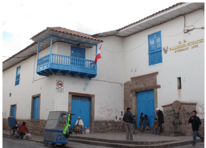
FIGURE 6.9 An example of an extant balcony at a nearby building on Calle Arones. The sawn-off beam ends at the northeast corner of Casa Arones suggest that it once had a similar balcony. Image: Sara Lardinois.
