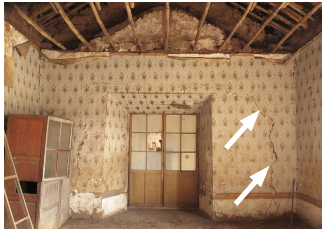
FIGURE 6.42 Vertical crack in transverse wall between rooms A-203 and A-204, adjacent to the east façade. Image: Claudia Cancino.
