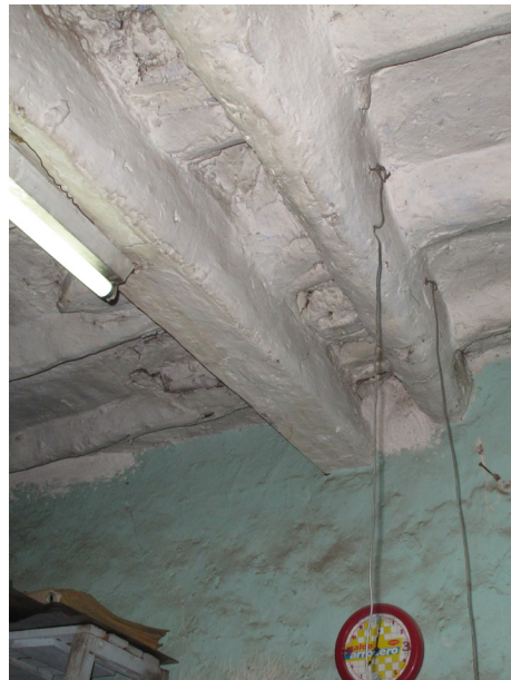
FIGURE 6.31 (LEFT) View of room C-109 ceiling, showing wood beam or girder, running in the east-west direction and supporting the floor joists above. Image: Sara Lardinois.
