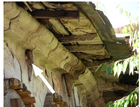
FIGURE 6.39 Wood key at intersection of tie beam and arcade wall, north side of patio. Image: Carina Fonseca.
