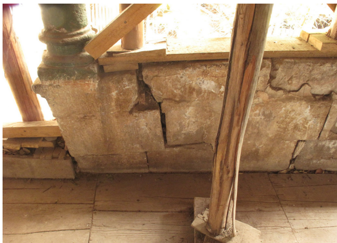
FIGURE 6.46 West end of stone masonry parapet wall at south arcade, as viewed from room B-206. Image: Sara Lardinois.
