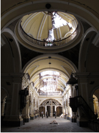
FIGURE 4.3 View of damages to the dome and vault resulting from the 2007 earthquake.
