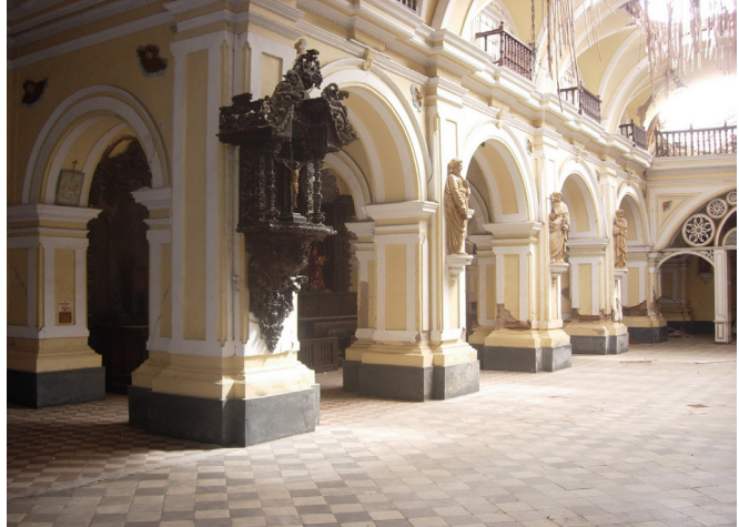
FIGURE 4.11 View of pillars between the nave and side aisles, 2007. Image: Philippe Garnier.
