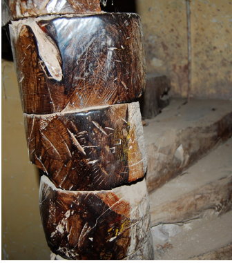
FIGURE 4.7 Heavy timber framing at spiral staircase in southeast bell tower, 2007. Image: Instituto Nacional de Cultura del Perú.
