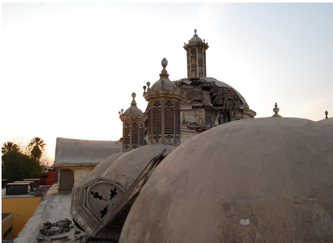
FIGURE 4.13 View of domes over south lateral aisle, with damaged main dome in the distance, 2007. Image: Instituto Nacional de Cultura del Perú.
