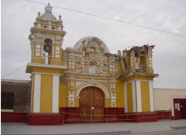
FIGURE 1.3 The earthen Church of El Carmen, Chíncha, Peru. The bell tower collapsed during the 2007 Pisco earthquake. Image: Philippe Garnier, for the GCI.
