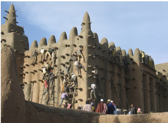
FIGURE 1.1 Great Mosque, Djenné, Mali. Regular maintenance of this earthen architectural masterpiece is carried out by the community at an annual festival. Image: Françoise Descamps.
