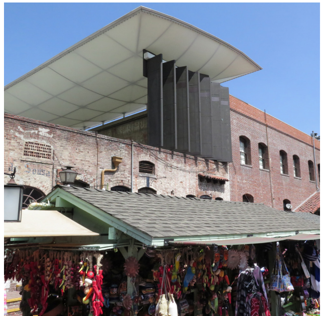
FIGURE 7 Protective shelter seen from Olvera Street, showing perforated copper side shades. Photograph by Leslie Rainer. © 2018 Getty Conservation Institute.
