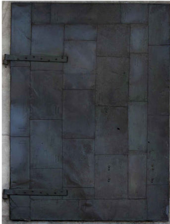
SHUTTER DOOR 1 (WEST) EXTERIOR
