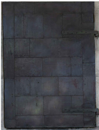
SHUTTER DOOR 2 (EAST) EXTERIOR
