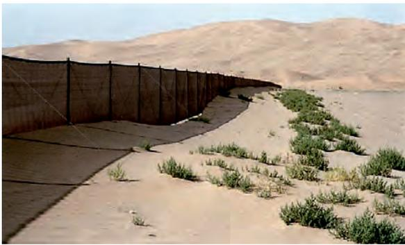
FIGURE 4 Sand accumulation around the wind fence.
