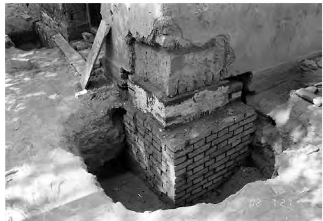
FIGURE 3 Wall stabilization with a brick footing.
