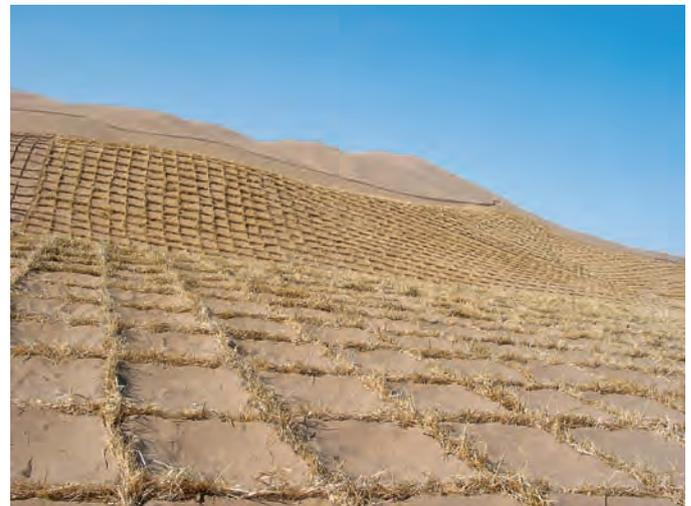
**FIGURE 2** Half-buried straw checkerboard barriers.
