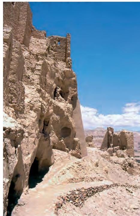
FIGURE 3 Cracking and threatened collapse of earthen architecture.
