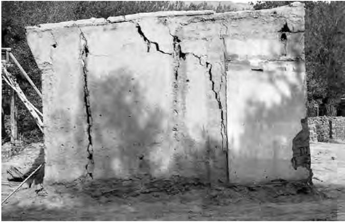
**FIGURE 1** Deteriorated north wall of a building in the Upper Temple before restoration.
