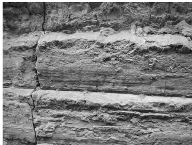
**FIGURE 2** Consolidation of the wall of the Yang Mausoleum. The left side is untreated; the right side is treated.
