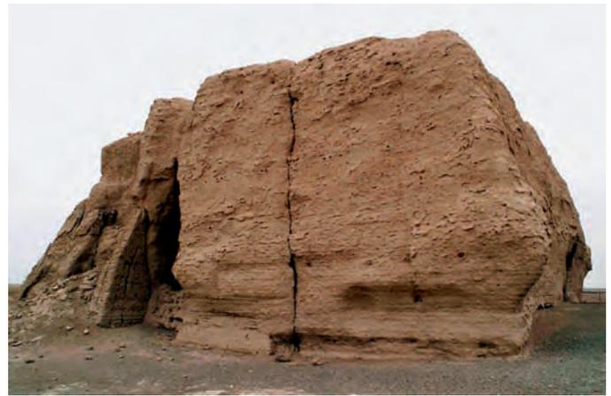
FIGURE 1 Condition of the Yumen Pass before consolidation.
