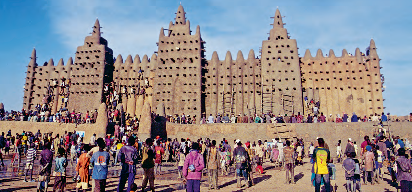
The annual community maintenance of the earthen Great Mosque of Djenné in Mali, in 2006. Photo: Jeanne Marie Teutonico, GCI.
