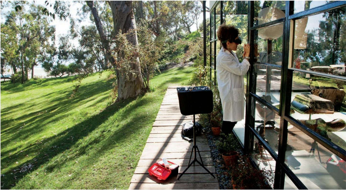
GCI project specialist Emily MacDonald-Korth carrying out on-site paint excavations on exterior metalwork at the Eames House. Right: A detailed view of the paint excavation being done with a stainless steel scalpel. Photos: Scott S. Warren, for the GCI.
