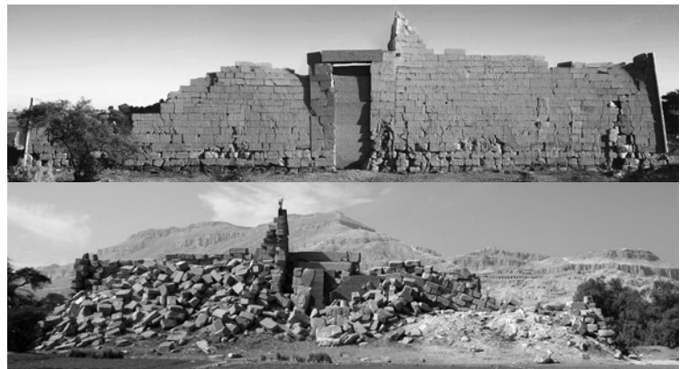
Views of both sides of the site’s first pylon, or gateway. The pylon suffers from both structural instability and a rising water table. The SCA and INSIGHT are currently engaged in a study to protect this monument. Photos: Courtesy of Christian Leblanc.
