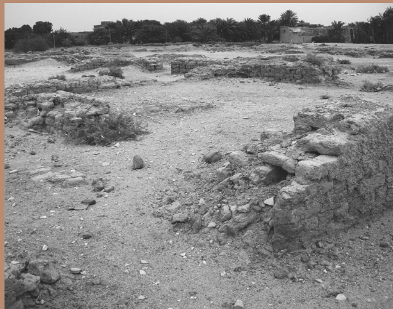
The crumbling mudbrick ruins of the sprawling palace complex of Amenhotep III, south of Medinet Habu. The mudbrick walls are displaying increasing decay because of changing weather and demographic conditions. Photo: W. Raymond Johnson.
