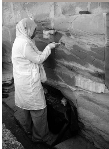
Chicago House conservator Hala Aly Handaqa infilling losses in the sandstone exterior wall blocks of the small Amun temple at Medinet Habu. Photo: W. Raymond Johnson.
