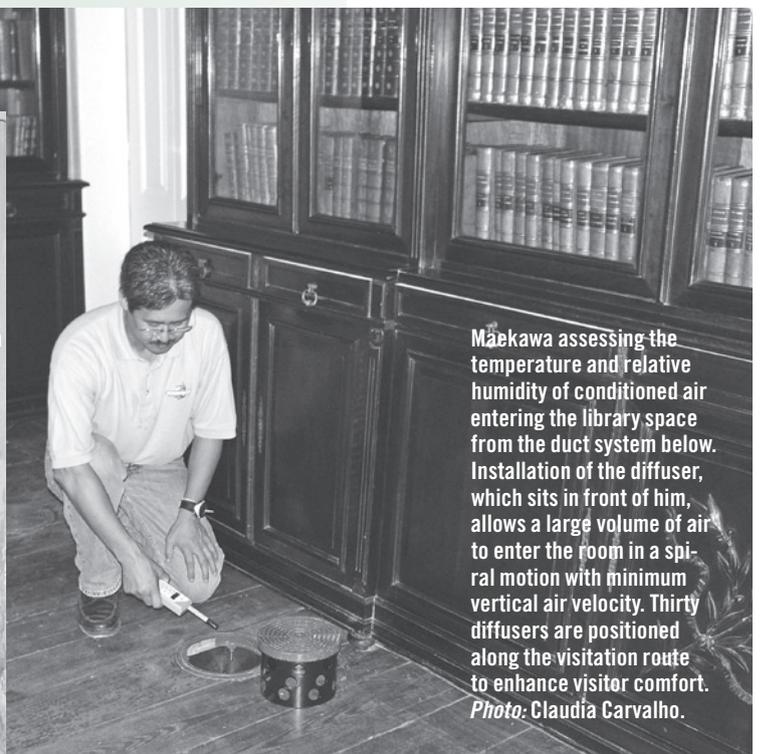
Maekawa assessing the temperature and relative humidity of conditioned air entering the library space from the duct system below. Installation of the diffuser, which sits in front of him, allows a large volume of air to enter the room in a spiral motion with minimum vertical air velocity. Thirty diffusers are positioned along the visitation route to enhance visitor comfort. *Photo: Claudia Carvalho.*
