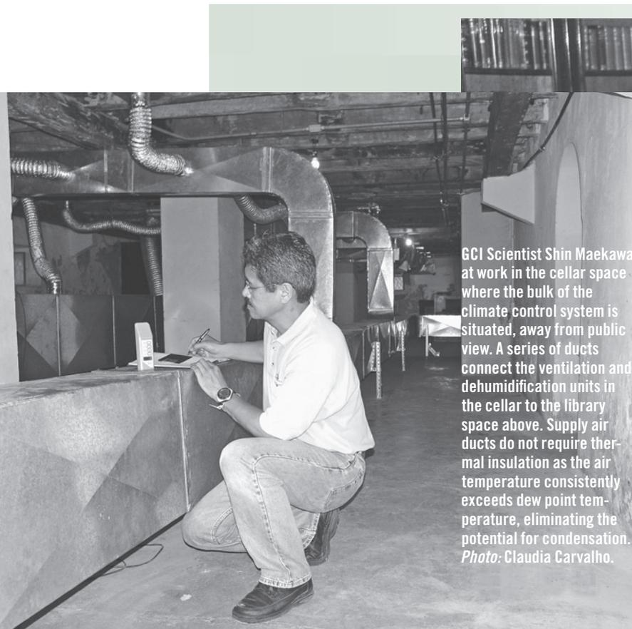
GCI Scientist Shin Maekawa at work in the cellar space where the bulk of the climate control system is situated, away from public view. A series of ducts connect the ventilation and dehumidification units in the cellar to the library space above. Supply air ducts do not require thermal insulation as the air temperature consistently exceeds dew point temperature, eliminating the potential for condensation. *Photo: Claudia Carvalho.*
