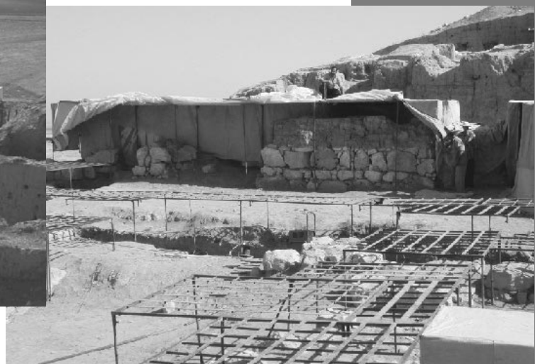
Left: A general view of the service wing of the Royal Palace, looking southwest. Tightly fitting canvas tents cover the metal cages to provide protection for the walls. Right: The covers can be quickly lifted to reveal the state of the walls. Photos: The International Institute for Mesopotamian Area Studies (images V13d8402 and V13d8567).
