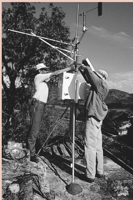
Installation this spring of site-monitoring equipment at the top of the hieroglyphic stairway in Copán. Photo: Shin Maekawa.
