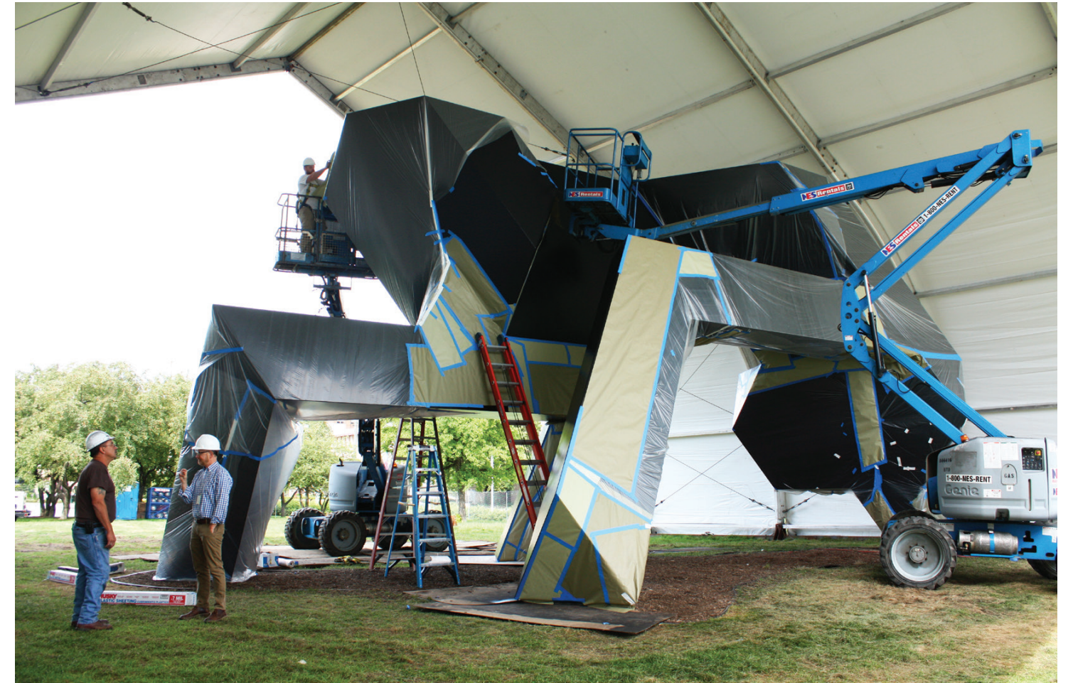
Above: On site application of high-performance coating for Gracehoper , 1961, Tony Smith. Welded steel and paint. Founders Society Purchase. Detroit Institute of Arts. Photo: Abigail Mack. © 2016 Estate of Tony Smith/Artists Rights Society (ARS), New York
