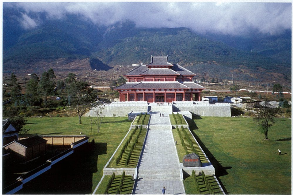
(Fig. 10) A place of local significance in Dali, Yunnan (stated by locals to have been destroyed in the Cultural Revolution), the Guanyin temple has been reconstructed in concrete and its bell tower made oversize to accommodate more tourists. (© J. Paul Getty Trust).
