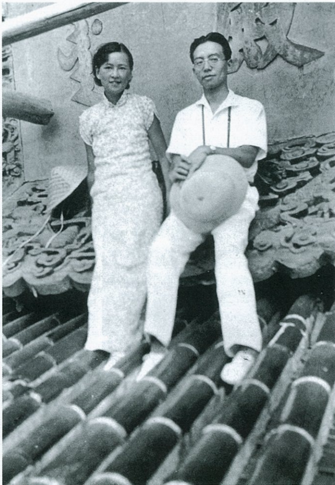
(Fig. 1) Liang Sicheng and his wife Lin Huiyin on the roof of the Temple of Heaven, Beijing, during field investigations (After Fairbank, 1994, fig. 18)
