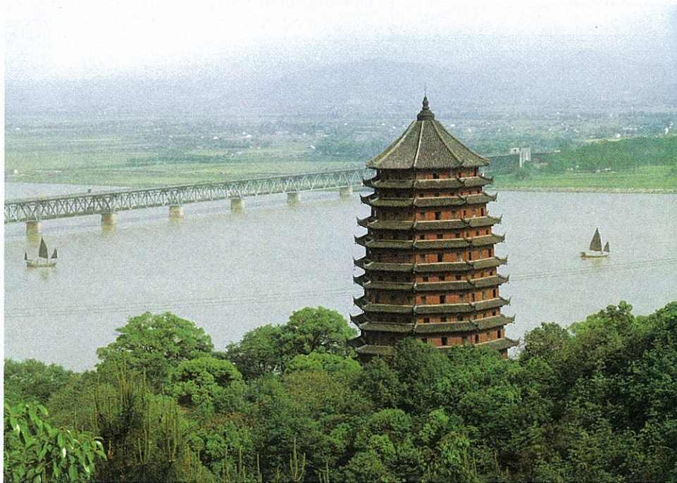
(Fig. 4) The Liuhe pagoda, Zhejiang. The brick core dates to the Southern Song dynasty (1127–1279); the outer wooden structure was built in 1900 (After Zhongguo jianzhu kexue yanjiuyuan, ed., Zhongguo gu jianzhu . Hong Kong, 1982, p. 110)
