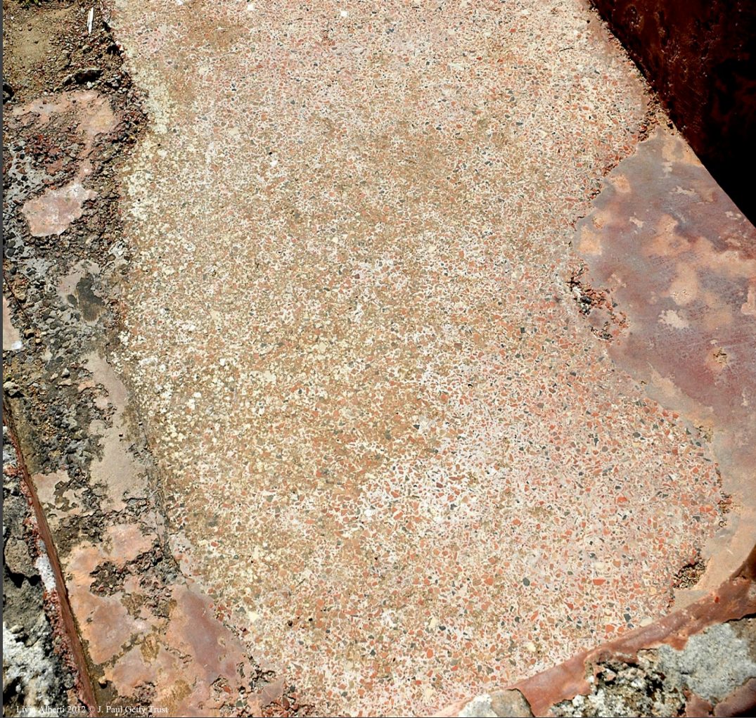
Cocciopesto - mortar with ceramic fragments
