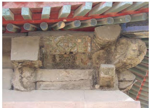
西北角，北墙 Northwest corner, north wall
