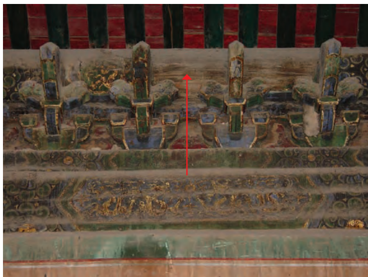
明间彩画细节，请注意檐檩上彩画的缺失 Detail of center bay showing loss of painting on the purlin.
