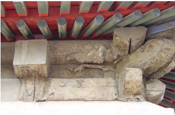
西南角，西墙 Southwest corner, west wall
