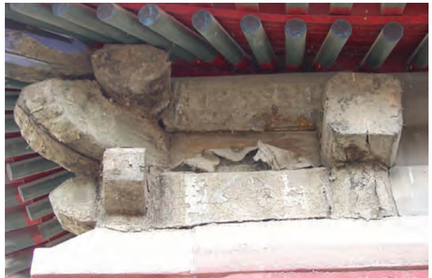
西南角，南墙 Southwest corner, south wall
