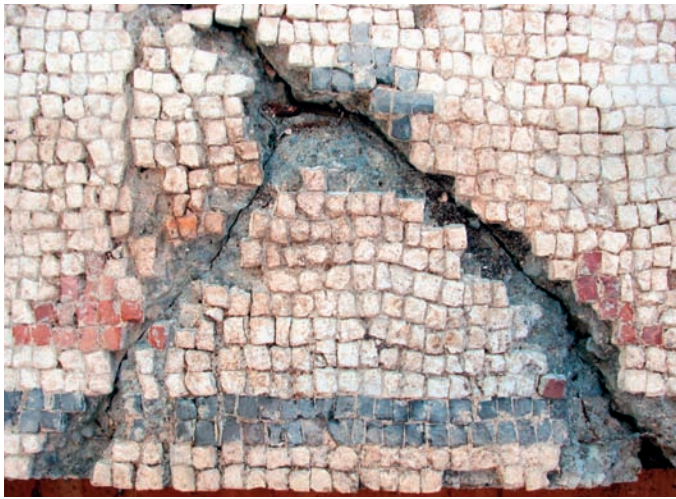
FIGURE 7 Damaged area resulting from cracked concrete backing before treatment. MFA 2002.128.2. Photo by C. Mei-An Tsu.
