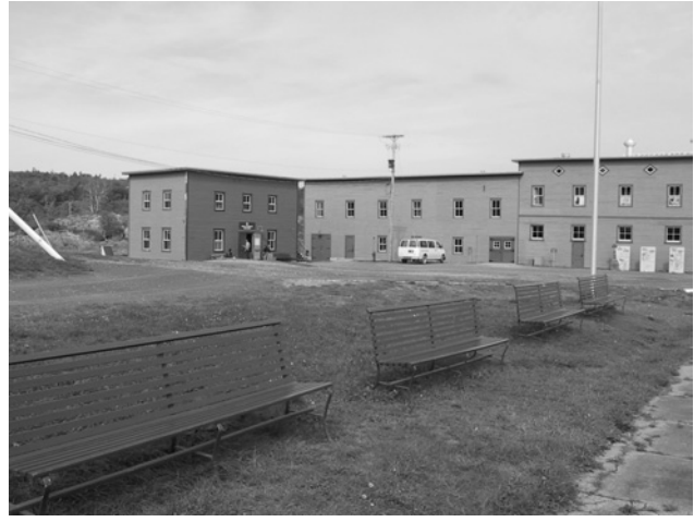
Figure 6. A view toward the east, showing the Disinfection Building and the Carpentry and Plumbing Workshop (now the Visitors Center and gift shop) at the left. Built in 1892 on the north end of the western wharf, the Disinfection Building housed three disinfection chambers and, eventually, showers. The south wing was erected in 1915 and the north in 1927. The Disinfection Building has been restored to its 1927 appearance; it is the first place modern visitors enter.
