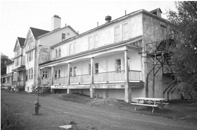
Figure 12. The First Class Hotel. Built in 1912 of concrete with some wooden cladding and other details, the First Class Hotel accommodated arriving passengers who were placed under medical observation. By the second half of the nineteenth century, the shipping companies had made it clear to the authorities that facilities for passengers being detained for medical reasons needed to correspond to their classes of passage, to avoid uncomfortable mixing of passengers.
