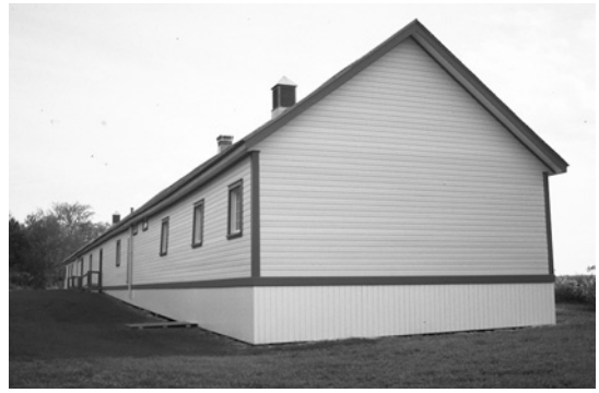
The west end and rear of the Lazaretto, showing some of the windows and doors in the back wall of the building, as well as the bead-board skirt that covers the replaced piers that support the building.
