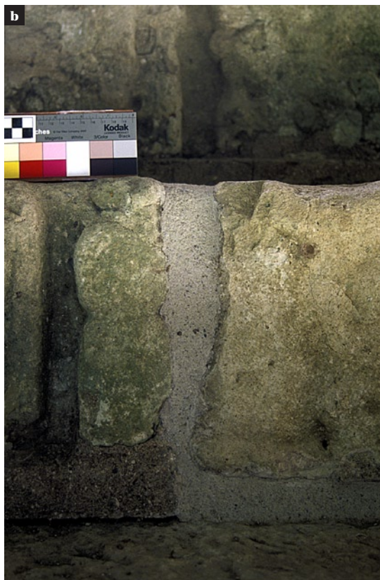
Figures 106a and b Comparison of two trial mortars for repointing: for block 406, step 43, the mortar was chosen to match the existing joint mortar (a); for block 488, step 52, the mortar was chosen to blend in with the variety of block colors (b).
