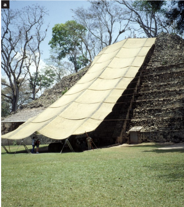
Figure 129 Shelter in 2005, with a modified lateral support system that keeps the tarpaulin taut.
