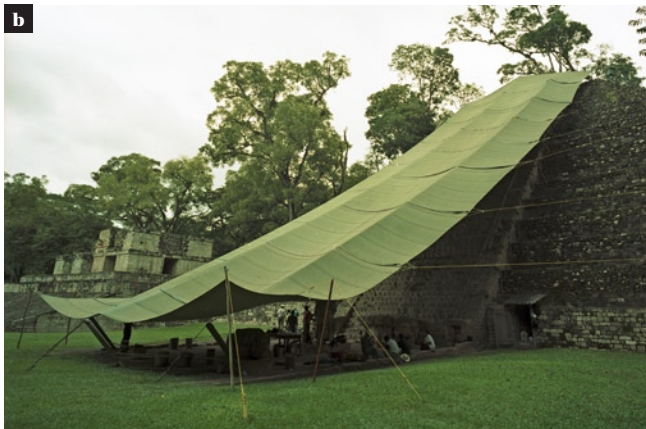
Figures 127a and b The shelter of the Hieroglyphic Stairway in 1992, with coverage that stops short of the top of the pyramid (a); a replacement tarpaulin, in place in 2001, offers greater coverage of the top of the pyramid (b).
