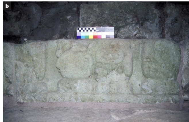
Figures 114a and b Treatment trial block 407, step 43, before (a) and after (b) treatment. There is an improvement in readability of surfaces after reduction of darkened consolidant from previous treatments and stabilization with edging repairs and with fills of lime-based mortars, colored with pigments to match the stone.
