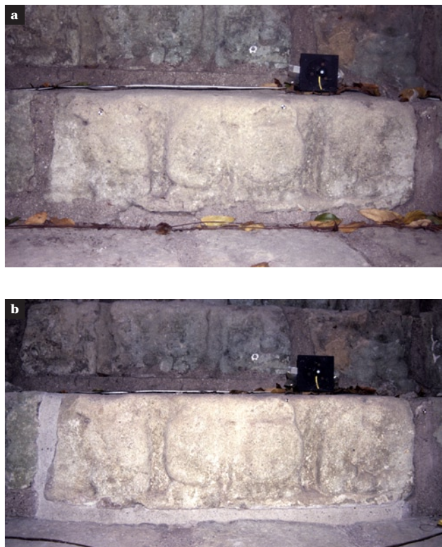
Figures 105a and b Treatment trial block 488, step 52, before (a) and after (b) mortar removal and repointing.
