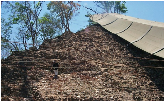
Figure 128 Shelter in 1998, with previous system of lateral supports.
