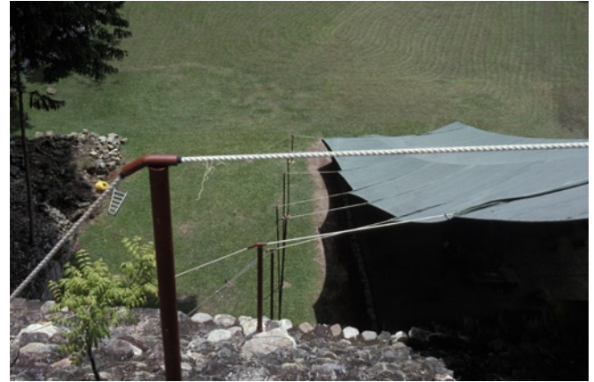
Figure 129 Shelter in 2005, with a modified lateral support system that keeps the tarpaulin taut.
