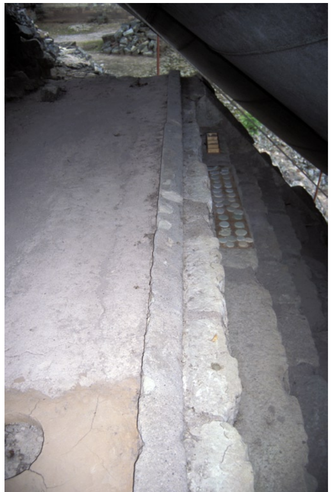
Figure 147 View of the mortar platform and cement lip above the last step of the reconstructed Stairway, looking south.
