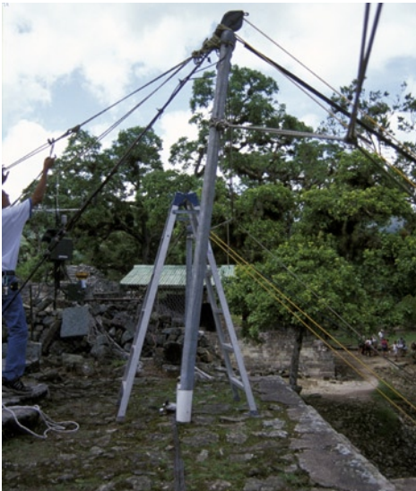
Figure 131 The central shelter cable support. Additional cable on the left keeps the support vertical.
