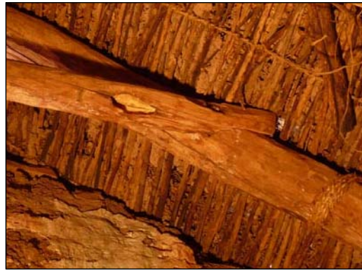
COLLAR TIE AND RAFTER JOINT
