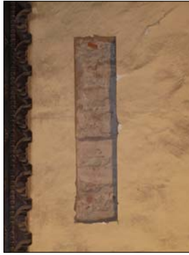
IS - 1B (CENTER OF WALL)
