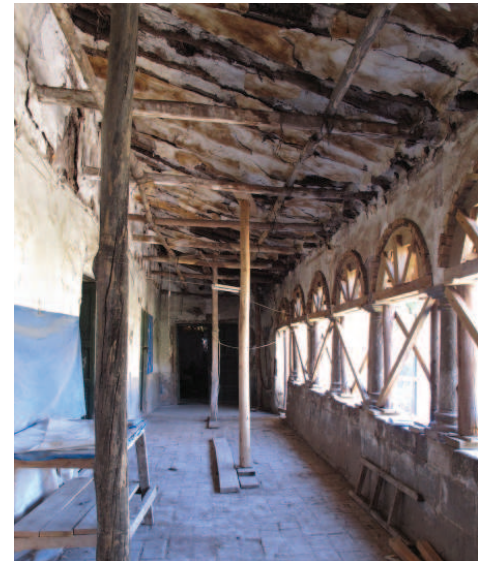
FIGURE 6.37 Exposed rafters at ceiling of gallery 210 Image: Sara Lardinois.
