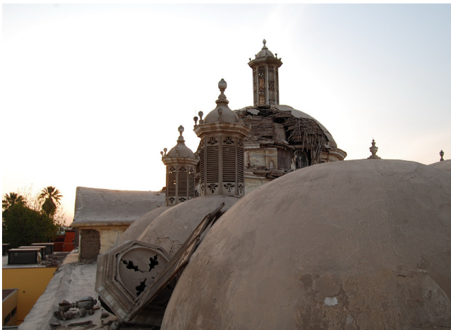
FIGURE 4.13 View of domes over south lateral aisle, with damaged main dome in the distance, 2007. Image: Instituto Nacional de Cultura del Perú.
