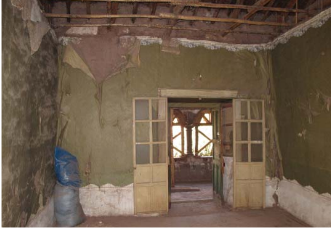
FIGURE 6.15 View of typical square-shaped room, C-201. Image: Sara Lardinois.
