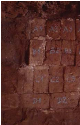
FIGURE 5.24 Fired brick floor pavers, as removed for the inspections and numbered for reinstallation. Image: Mirna Soto, for the GCI.
