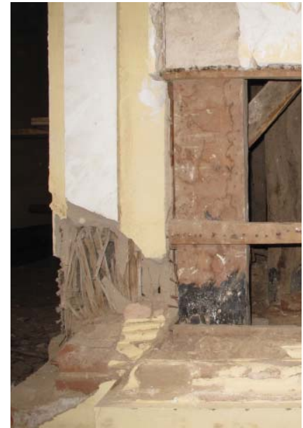
FIGURE 4.24 View of pillar base, above brick base. Image: Sara Lardinois.
