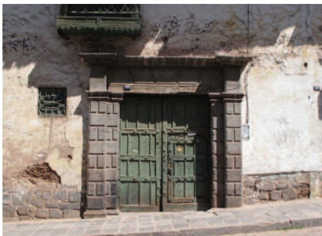
FIGURE 6.8 Detail view of entrance portal at east façade. Image: Sara Lardinois.
