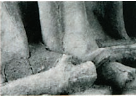
FIGURE 9. Detail of one of the figures from Frederiks Church showing places where water could be trapped by the shape of the figure. These areas have been filled with mortar to prevent damage from freezing water or to prevent water from seeping in through cracks and holes.
