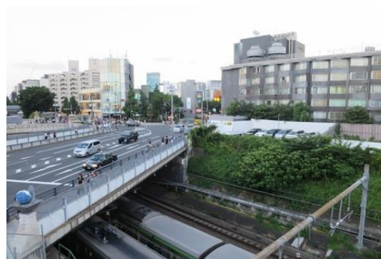
Fig. 3-2 Olympic Bridge (Source: http://tomagazine.jp/news/599/ )
