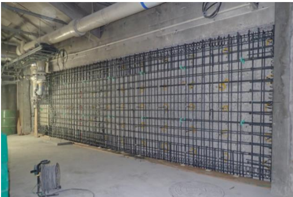
Photo 2-1 Wall repair (thickening the wall by newly adding a bearing wall)
