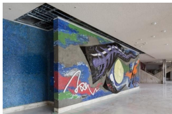
Photo 2-2 Wall repair (Reinforcing a concrete block wall)
