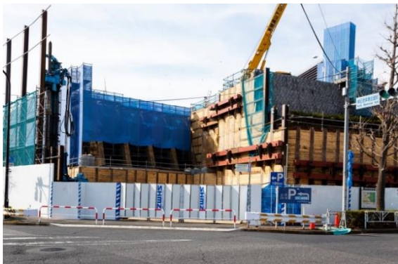
Photo 2-9 Retaining wall renovation
