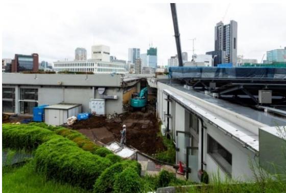
Photo 2-7 Restructuring the building frame of the area around the pool and connecting spaces
