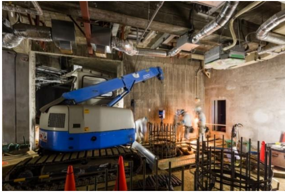
Photo 2-3 Pile installment and base reinforcement work
